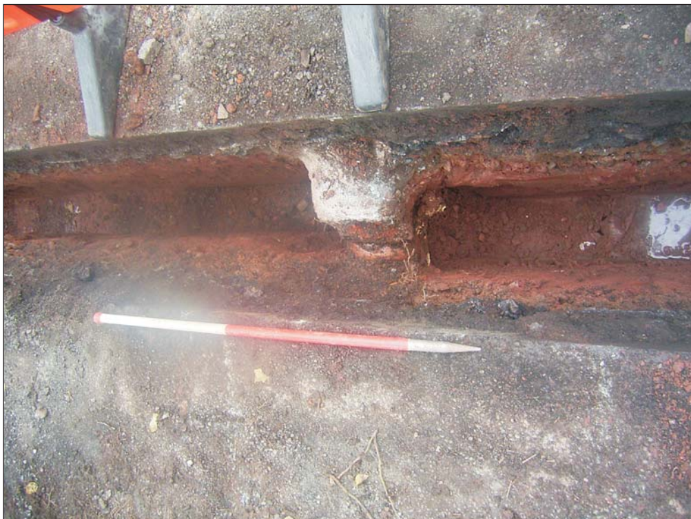
Plate 2: Concrete capped culvert
