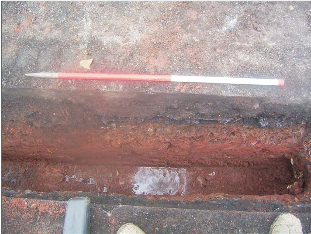
Plate 1: South west facing section of pipe trench
