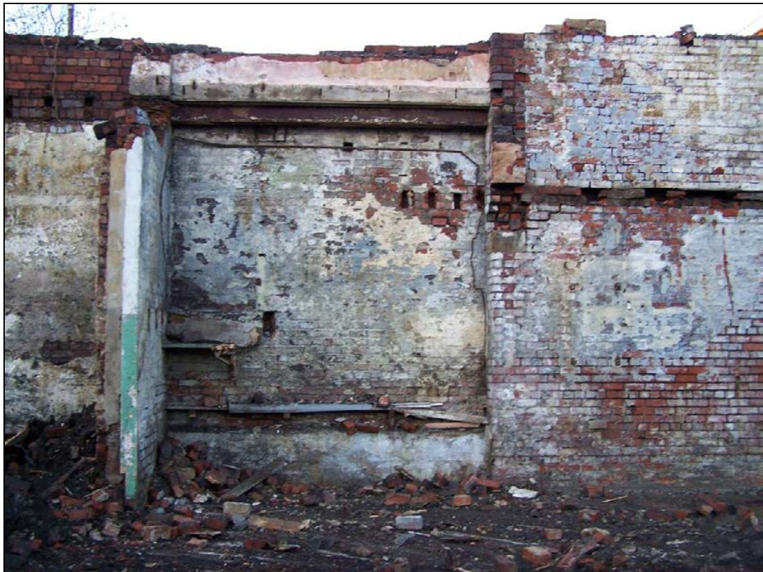
Plate 117: View of north wall of G3, west range extension, showing join with north and west ranges and I-section beam carrying first floor north wall (film D.2)
