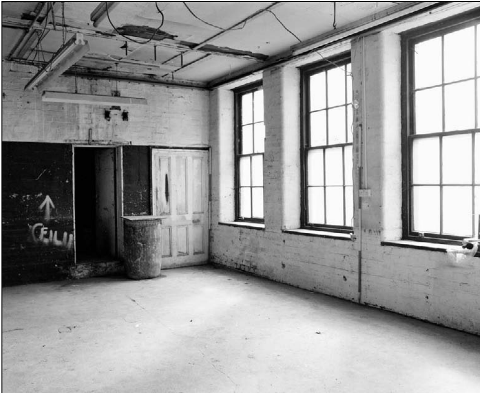
Plate 123: General view of room G21, west range (film 15.9)
