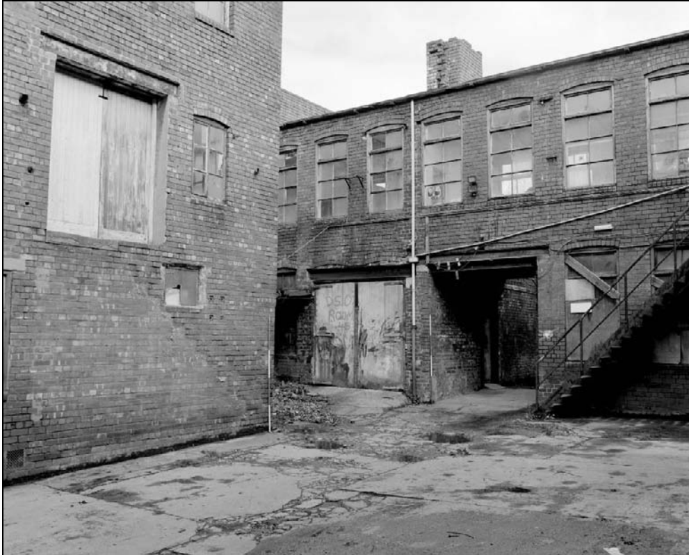
Plate 312: General view of west elevation of east range – removed second floor with projecting truncated chimney breast (film 9.6)
