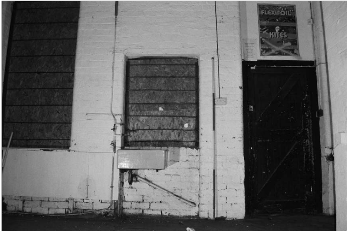
Plate 246: Detail of window within former doorway and doorway within former window, north wall of G20, south range (film 3.4)
