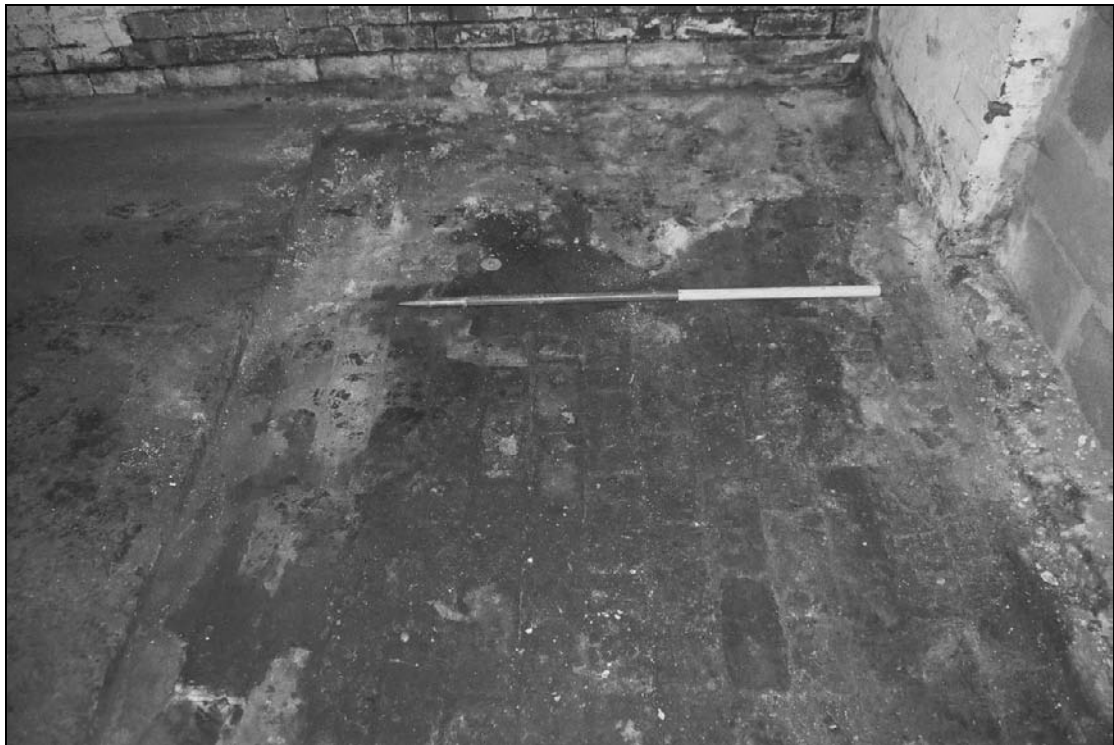
Plate 371: Detail of original brick floor of G6, north range (film 42.30)
