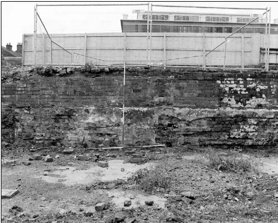
Plate 45: Detail of lower section of south elevation of south range (east end) showing paintwork from former attached structures (film 49.4)
