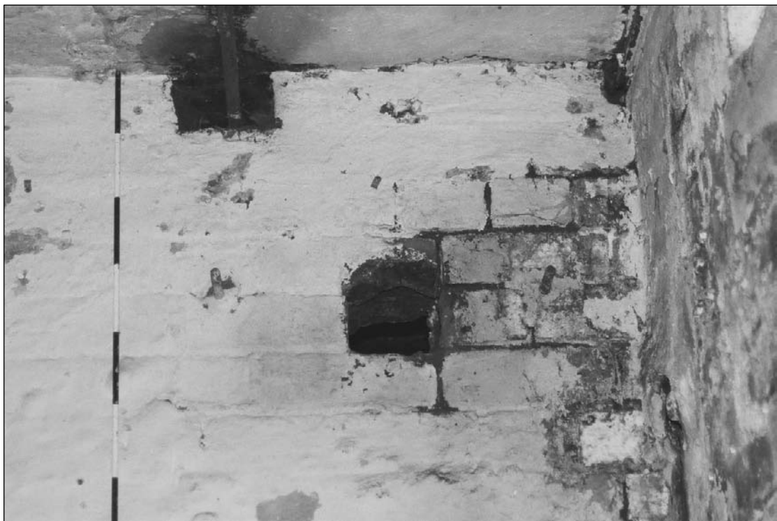
Plate 373: Detail of hole and fixings in north wall of G6 (film 42.21)
