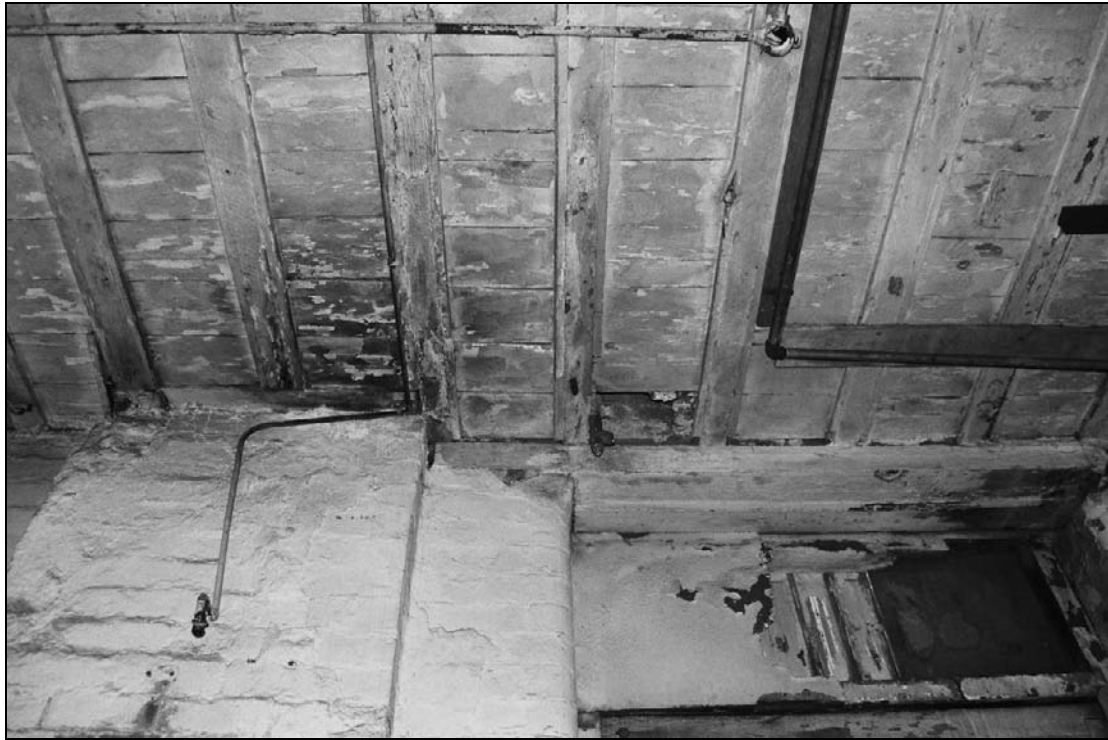
Plate 269: Detail of brick flue and ceiling of G16, south range (film 22.1)
