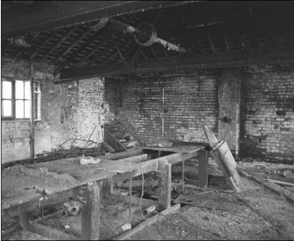
Plate 394: General view of S5, north range – note doorway from S4, workbenches and line shafting (film 45.1)
