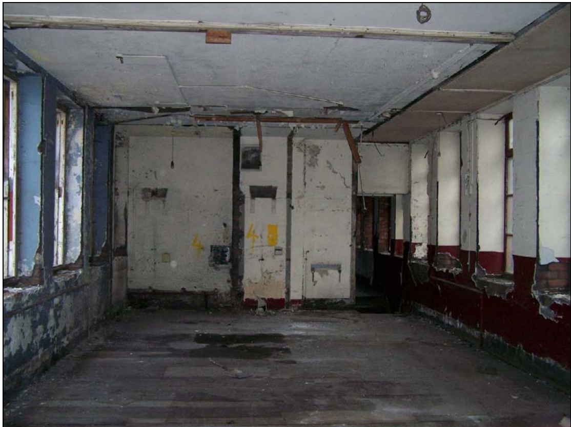
Plate 146: View of rooms F11-F16 & F18 after removal of partitions (film D.4)
