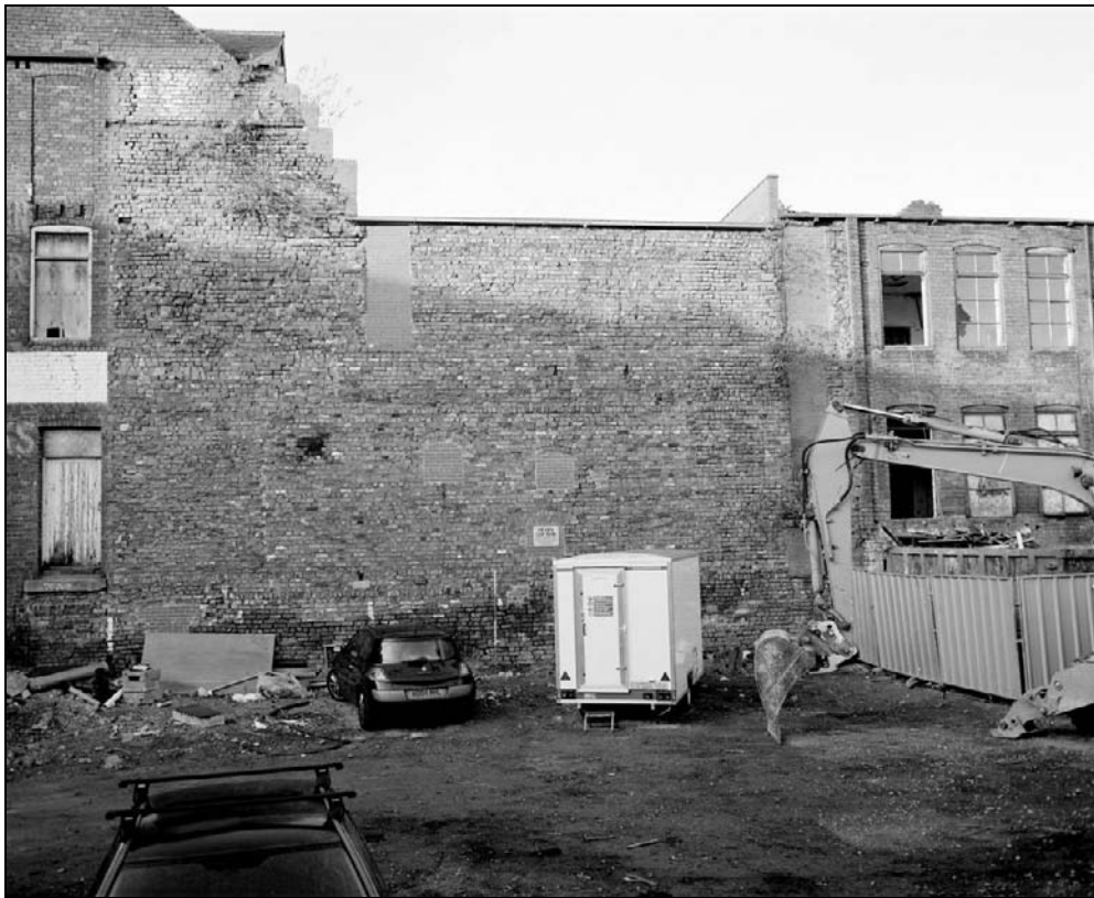
Plate 23: General view of the south elevation of the south and west ranges (film 47.6)
