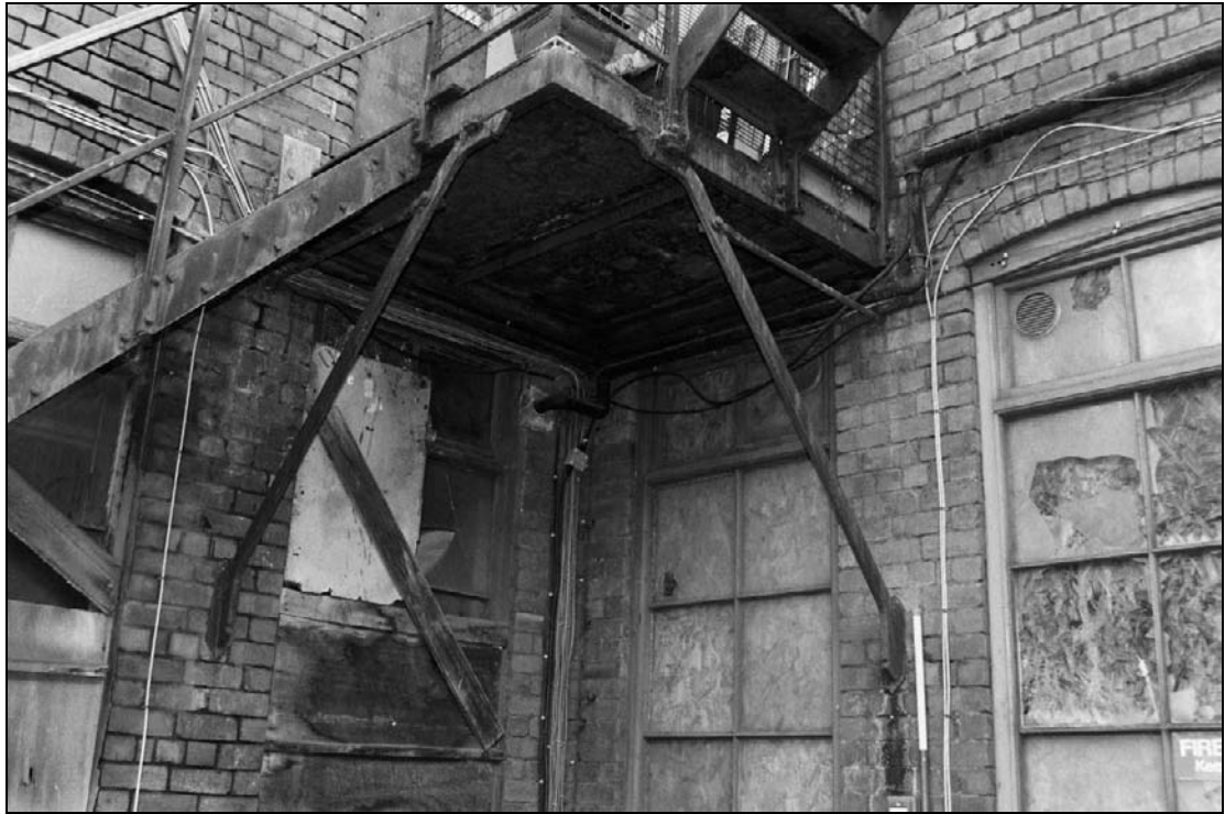
Plate 224: Detail of external staircase and supporting brackets (film 27.15)
