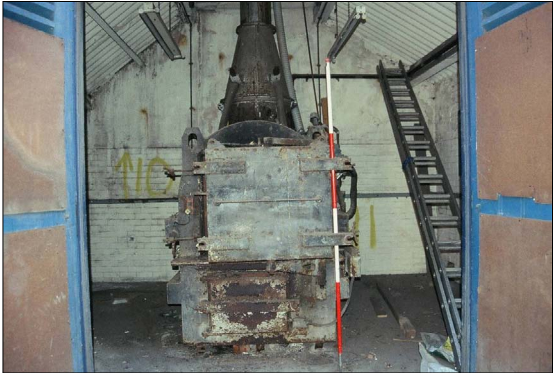
Plate 420: General view of G10, furnace house range, west building showing inserted incinerator (film C/S 3.1)
