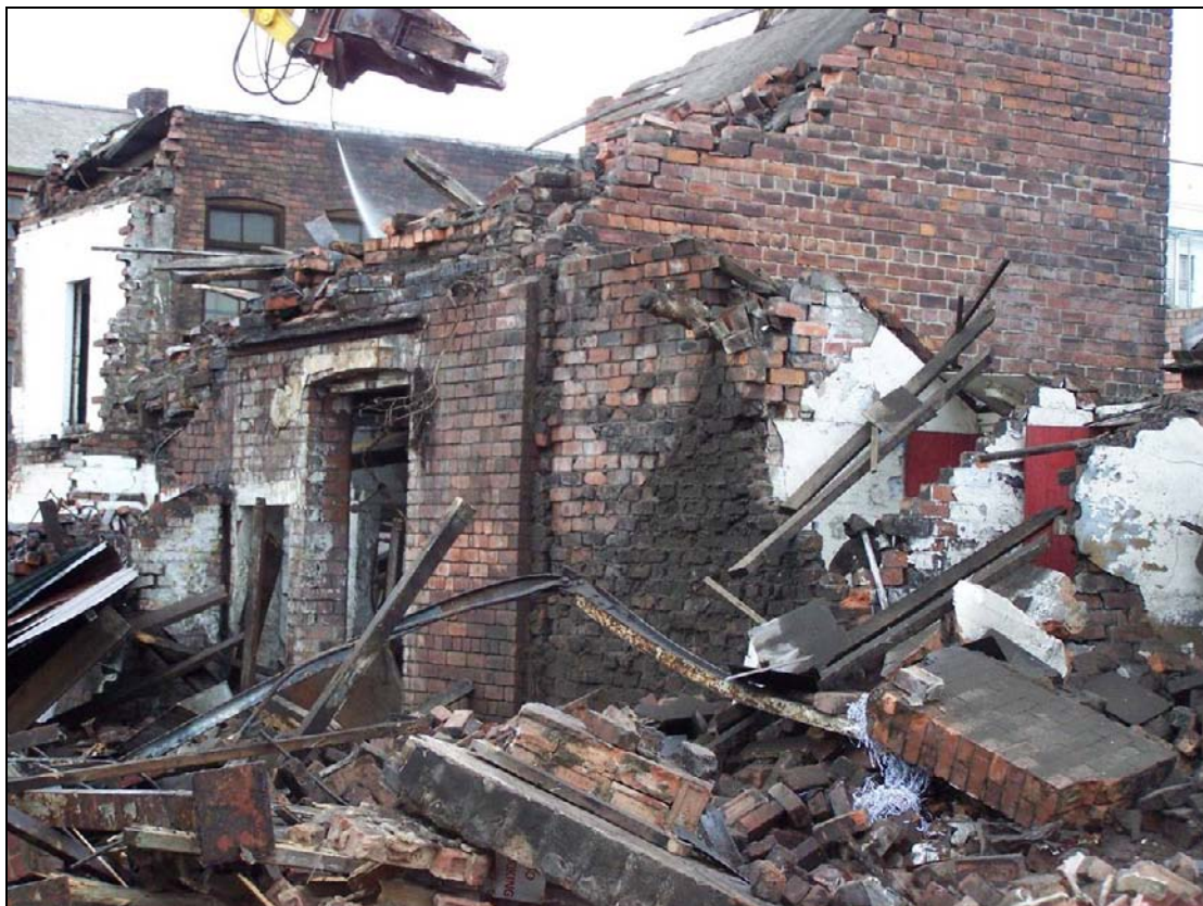
Plate 270: View depicting doorway into G16 from G15 machine shop – showing original type 9 window features, south wall of G16, south range (film D.17)
