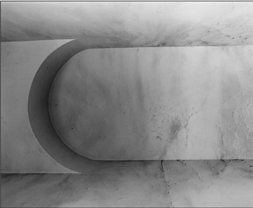
Plate 155: View of arch above stairs, F18 (film 31.3)
