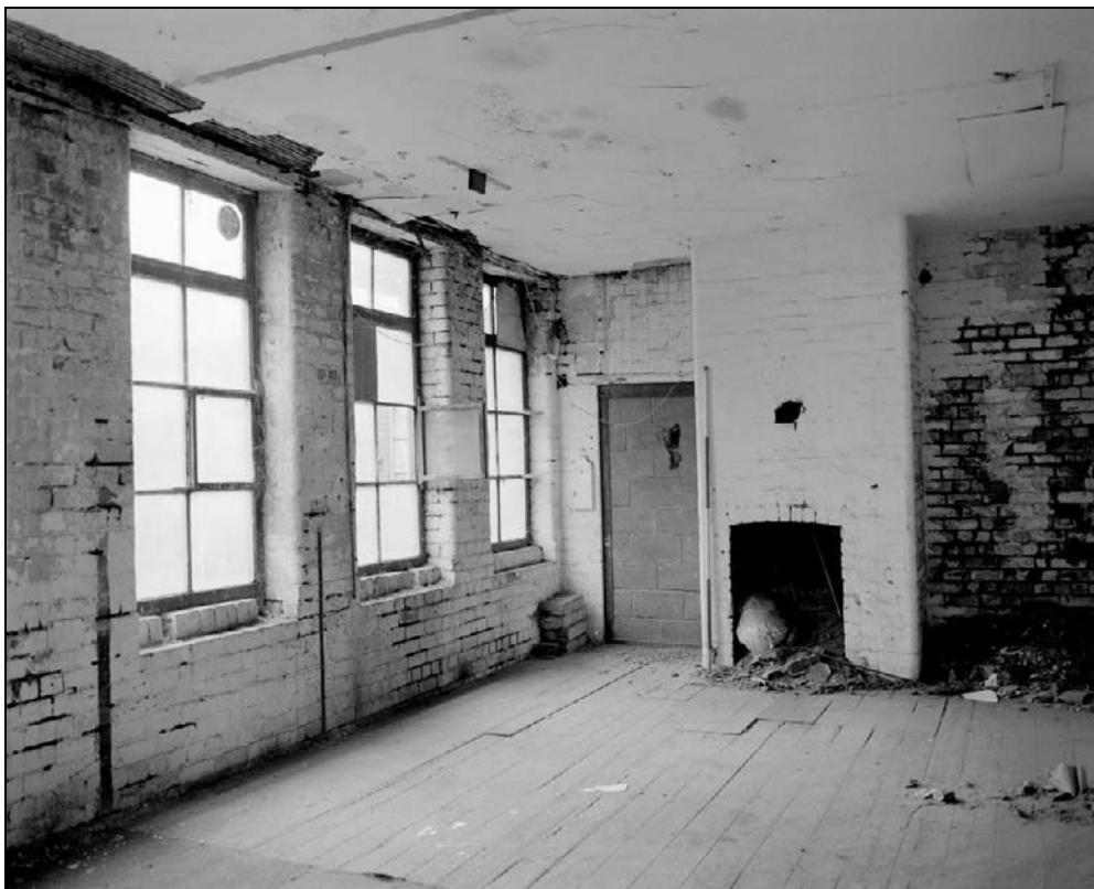
Plate 276: General view of F10, south range (west end) (film 29.2)
