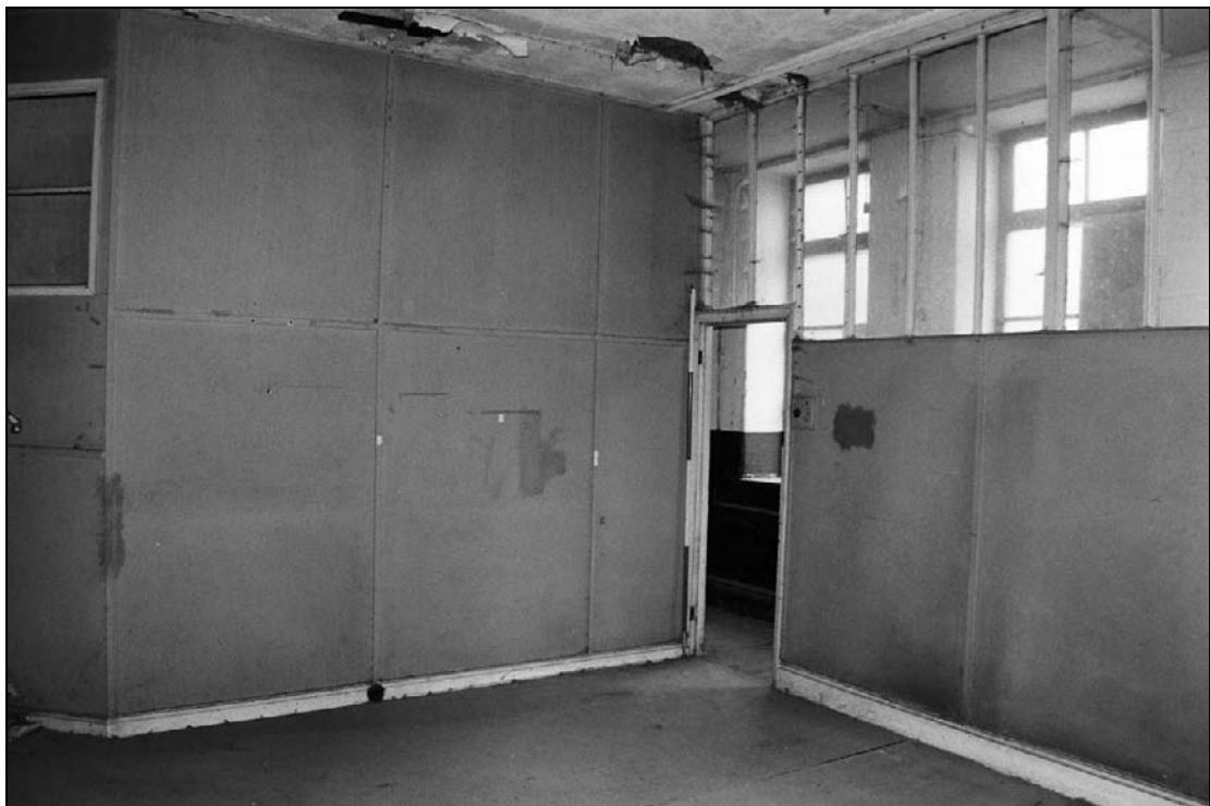
Plate 136: General view of F13 showing inserted partitioning (film 25.15)
