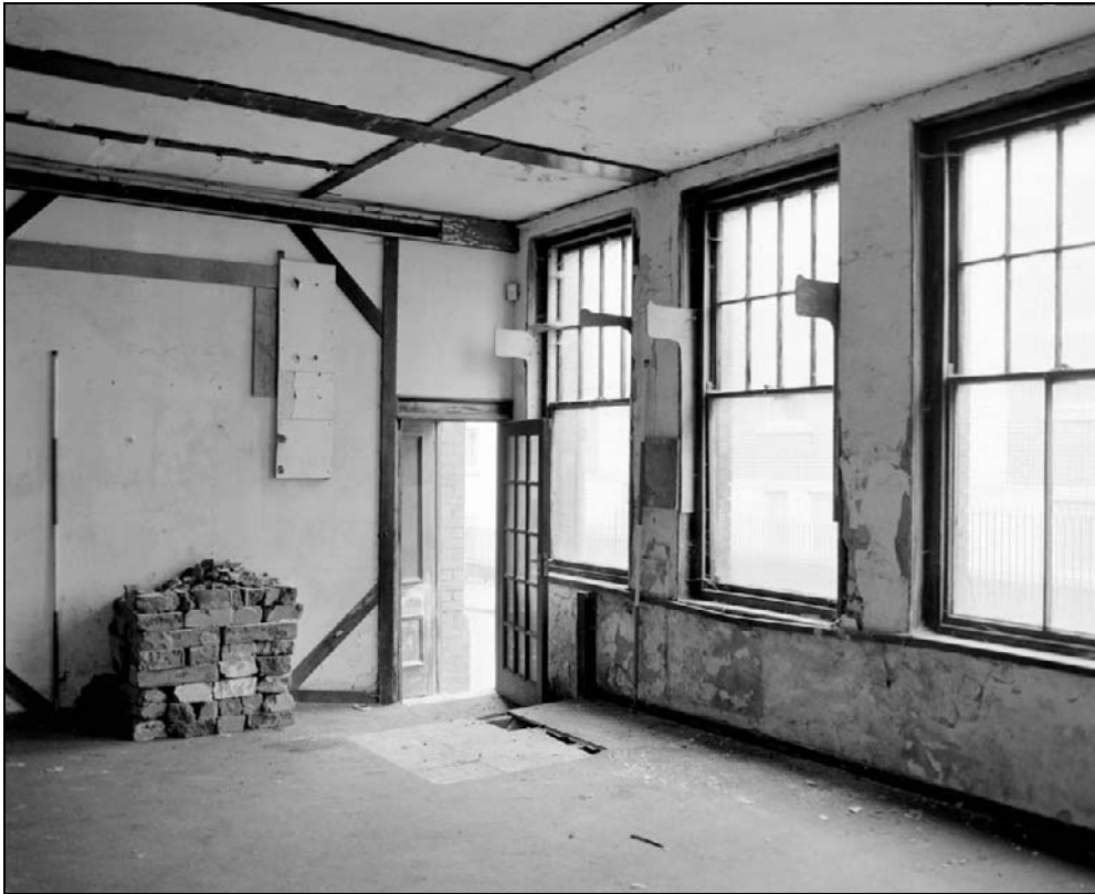
Plate 100: General view of room G2, west range, looking towards G1 (film 13.5)
