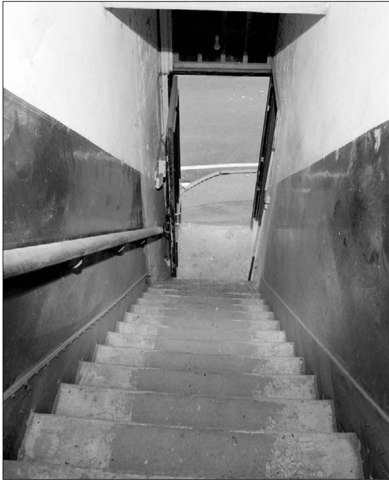
Plate 153: View from F18 down stairs to G1 (film 31.2)
