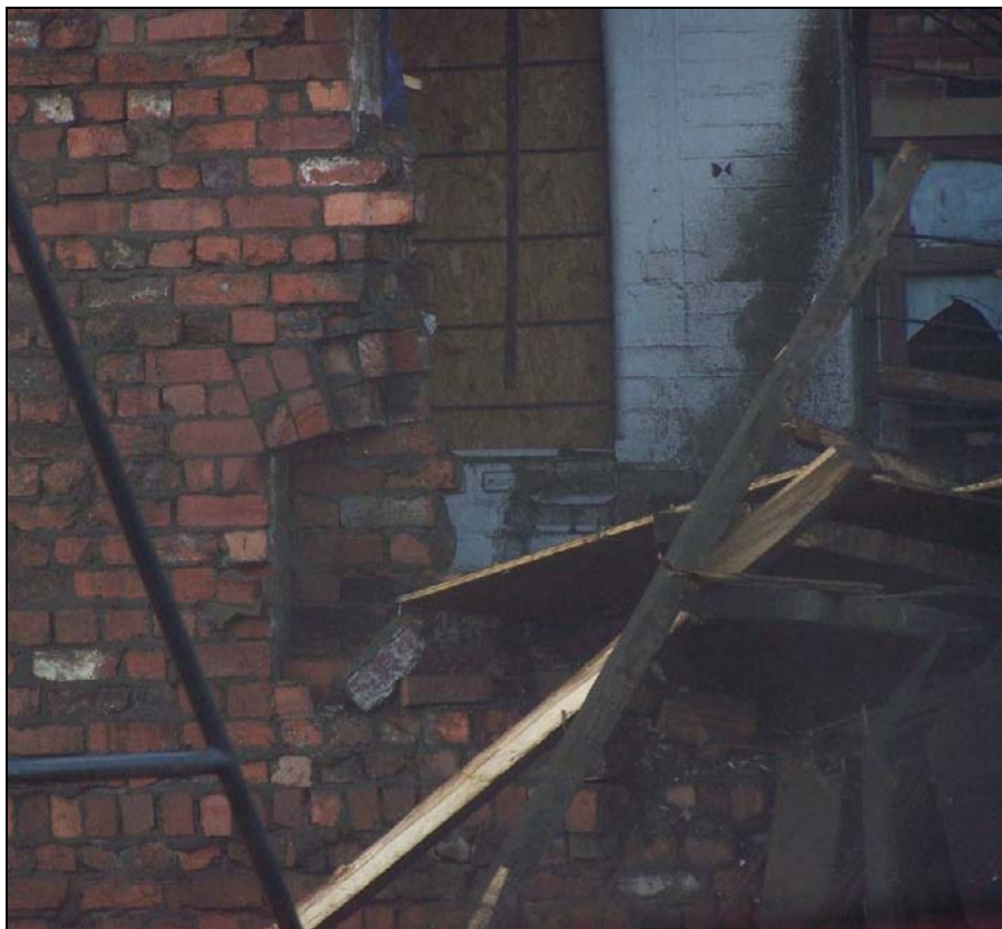
Plate 311: Detail of blocked arched opening showing painted reveals, south elevation of south range (film D.21)
