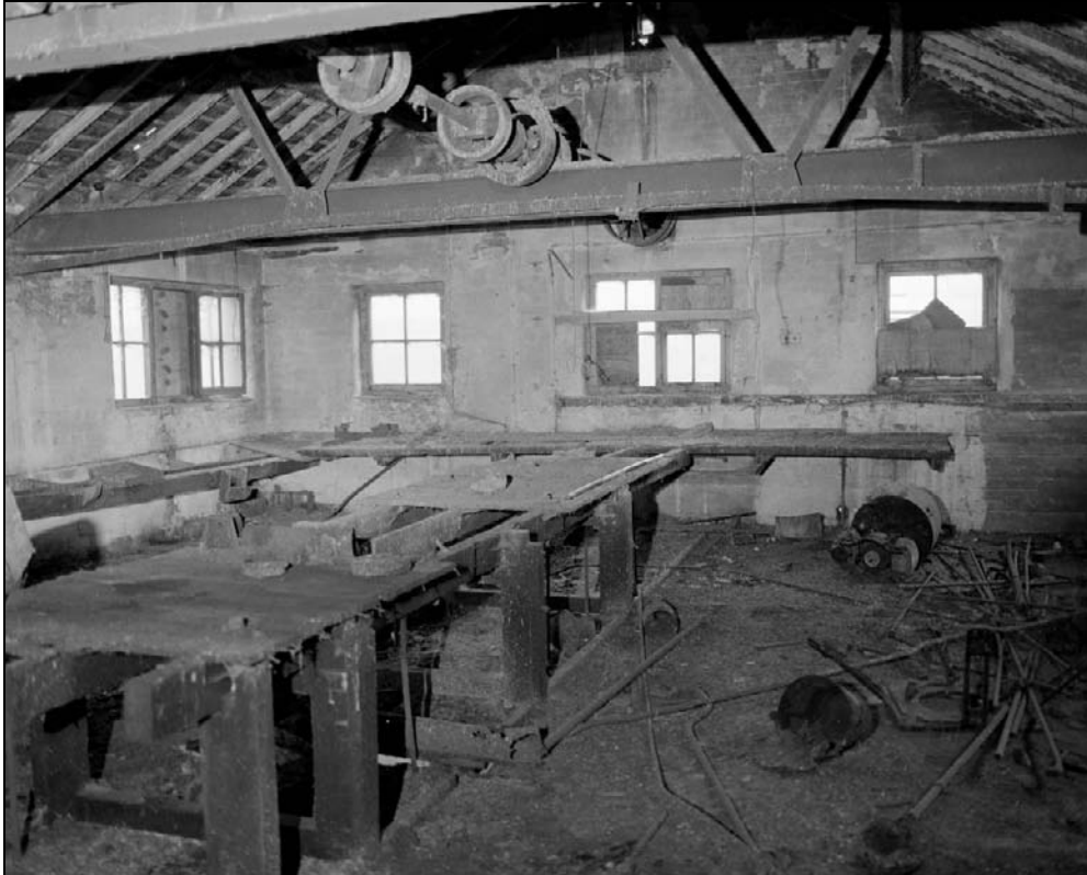
Plate 392: General view of S5, north range – note workbenches and overhead line shafting (film 45.6)
