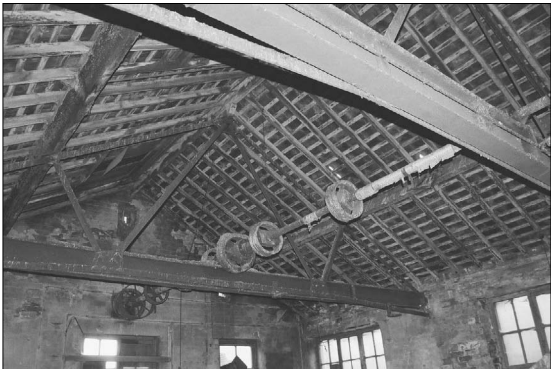
Plate 397: Detail of roof structure and line shafting, S5, north range (film 44.17)
