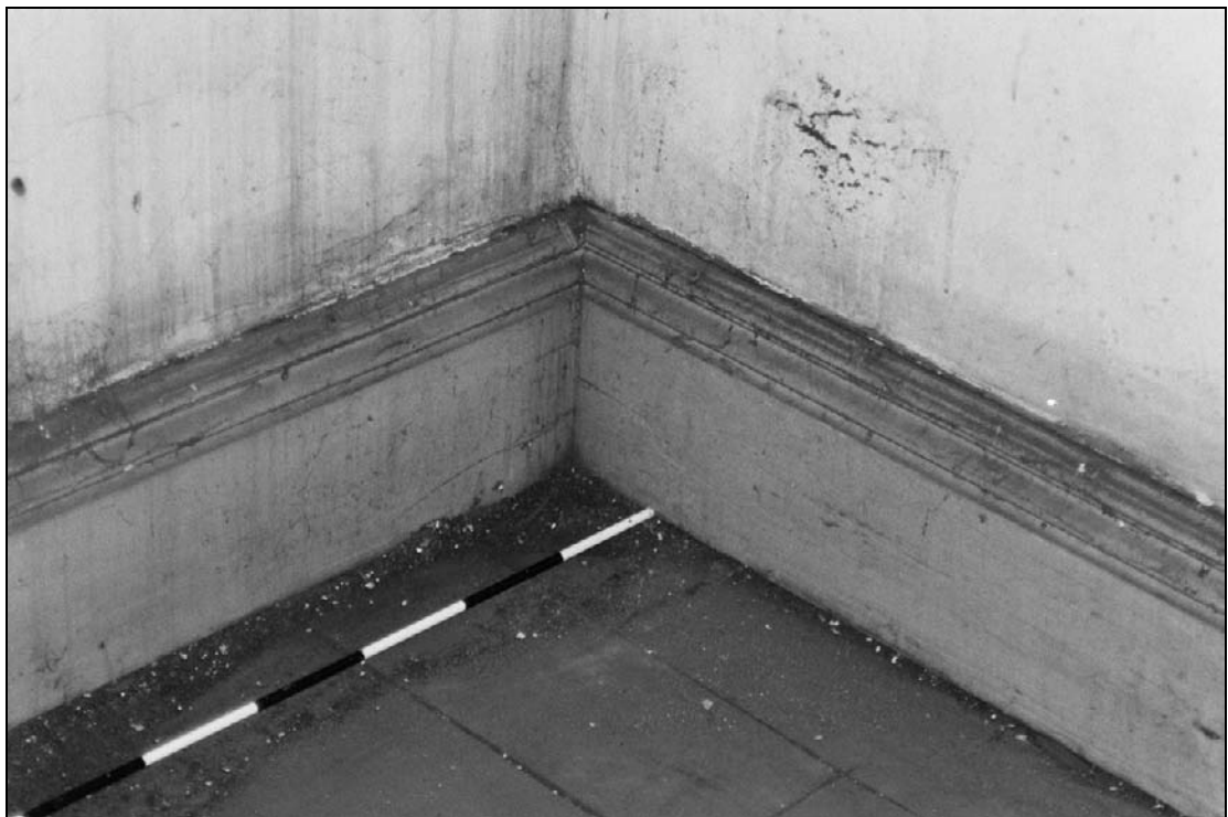
Plate 164: Detail of original skirting, room F1 (film 25.35)
