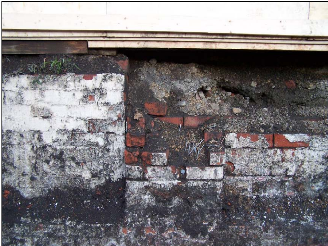
Plate 327: Detail of blocked type 4 windows within east wall of G7, east range (film D.22)
