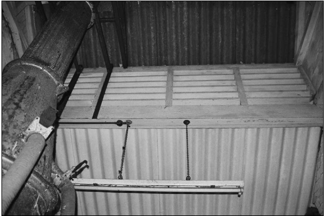
Plate 422: Detail of louvered roof of G9 and G10, furnace house range, west building (film 22.19)
