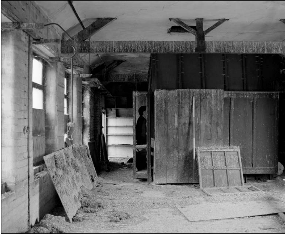
Plate 183: View of S2 showing partitioned S1 within the southwest corner (film 38.6)
