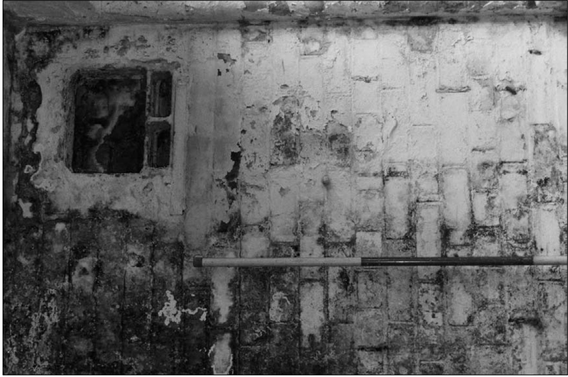
Plate 385: Detail of wall box, north wall of F4, north range (film 24.26)
