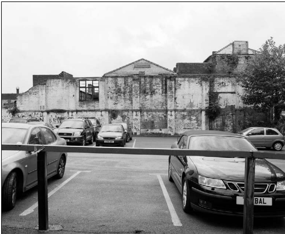
Plate 64: General view of the north elevation of the east, north and west ranges (film 4.10)
