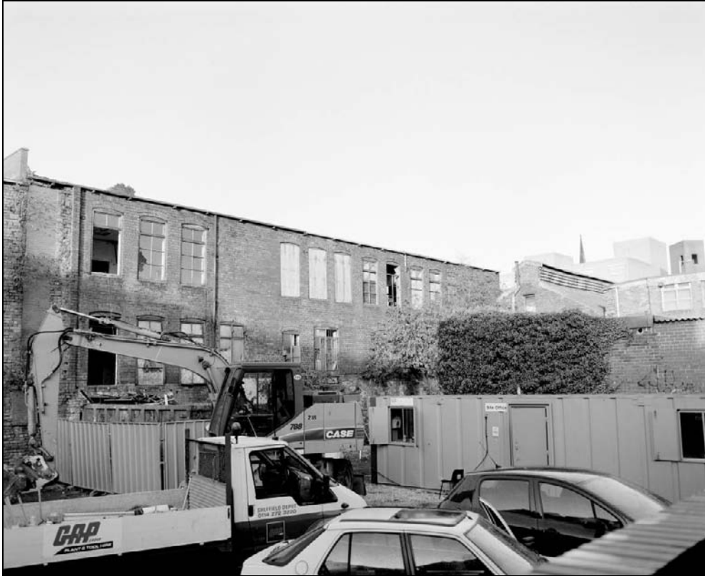
Plate 33: General view of south elevation of south range (east end) (film 47.7)
