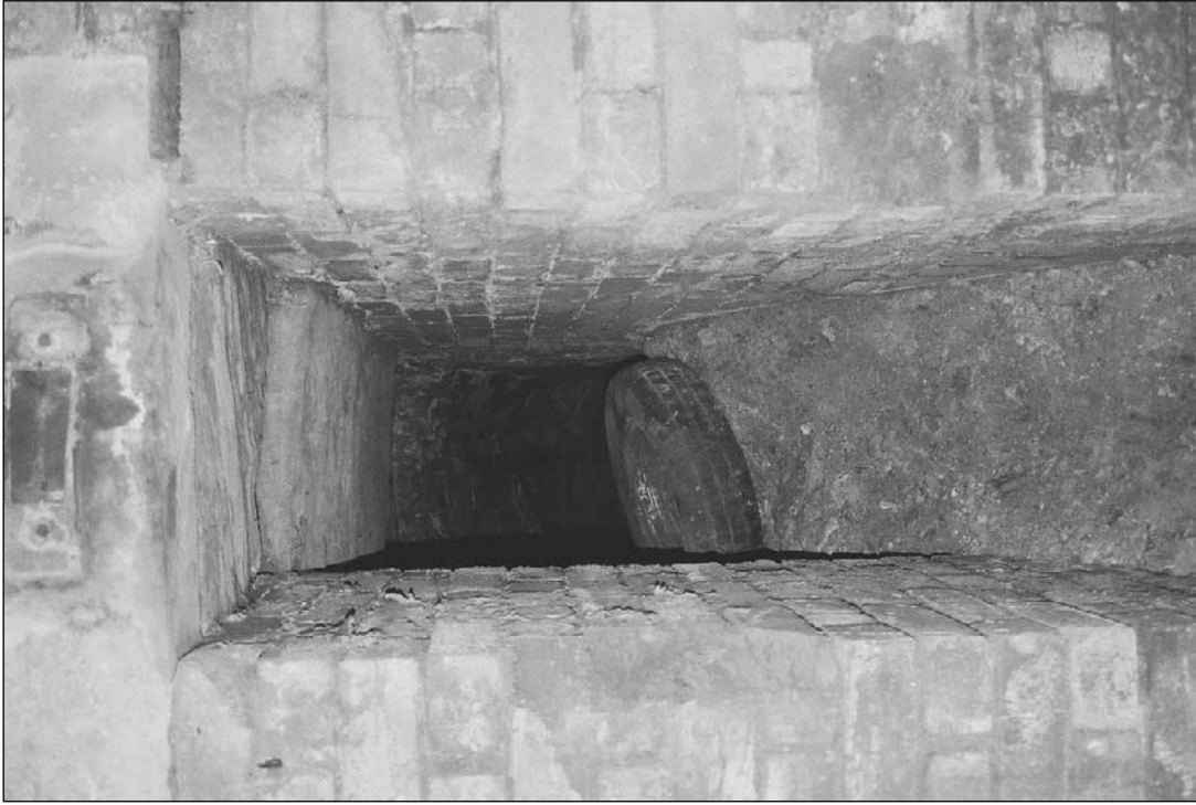
Plate 92: View along P2, northeast corner of B3, west range (film 2.4)
