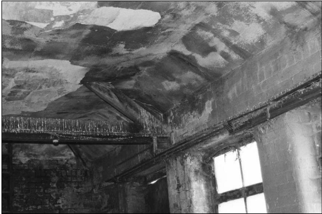
Plate 205: Detail of lath and plaster ceiling, trusses and shelves, S3 (film 41.31)
