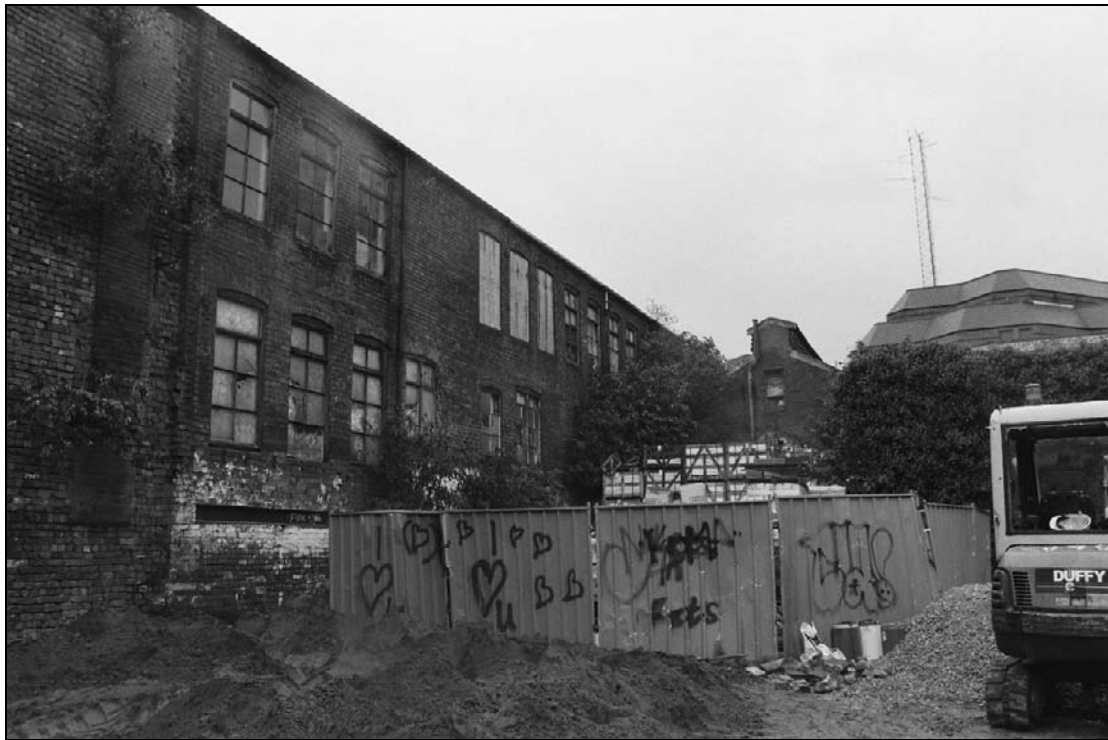
Plate 38: General view of south elevation of south range (east end) (film 1.10)
