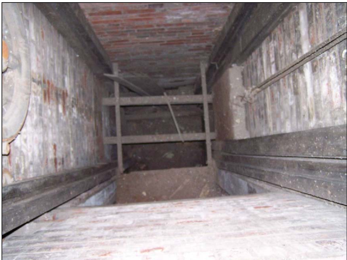
Plate 148: View of lift shaft (film D.6)
