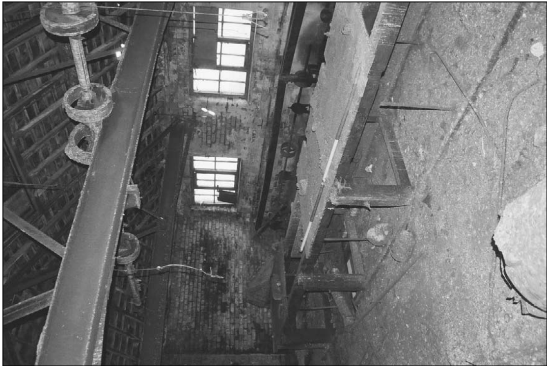
Plate 398: View showing overhead and below line shafting and central workbench (film 44.27)
