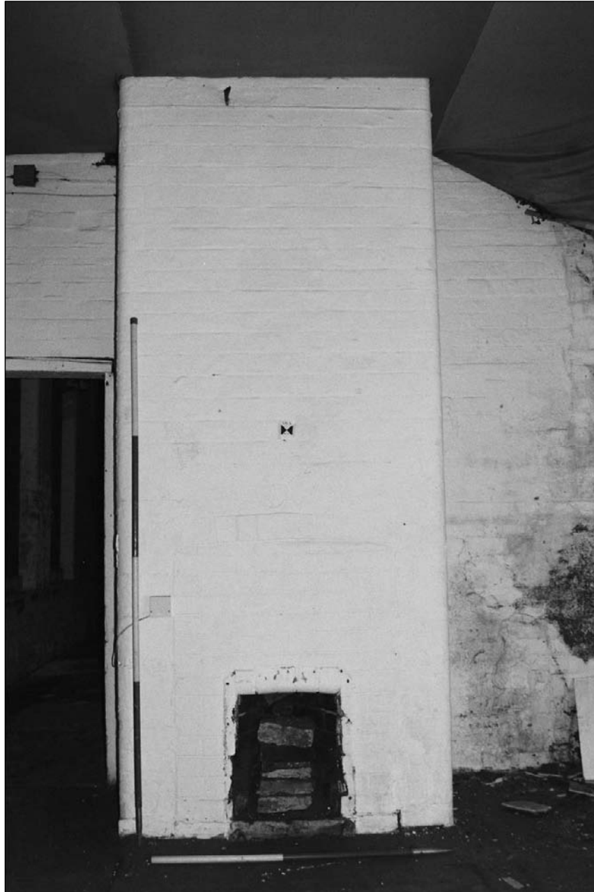
Plate 245: Detail of altered fireplace, east wall of G20, south range (film 3.2)
