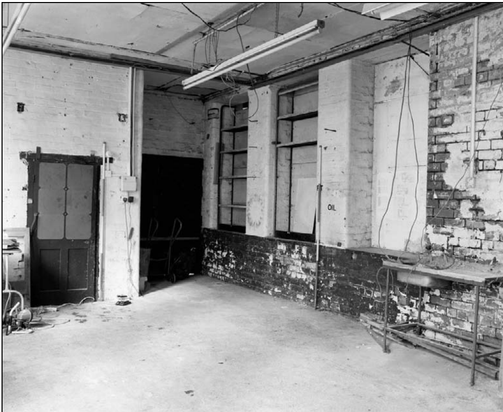
Plate 124: General view of room G21, west range (film 16.1)
