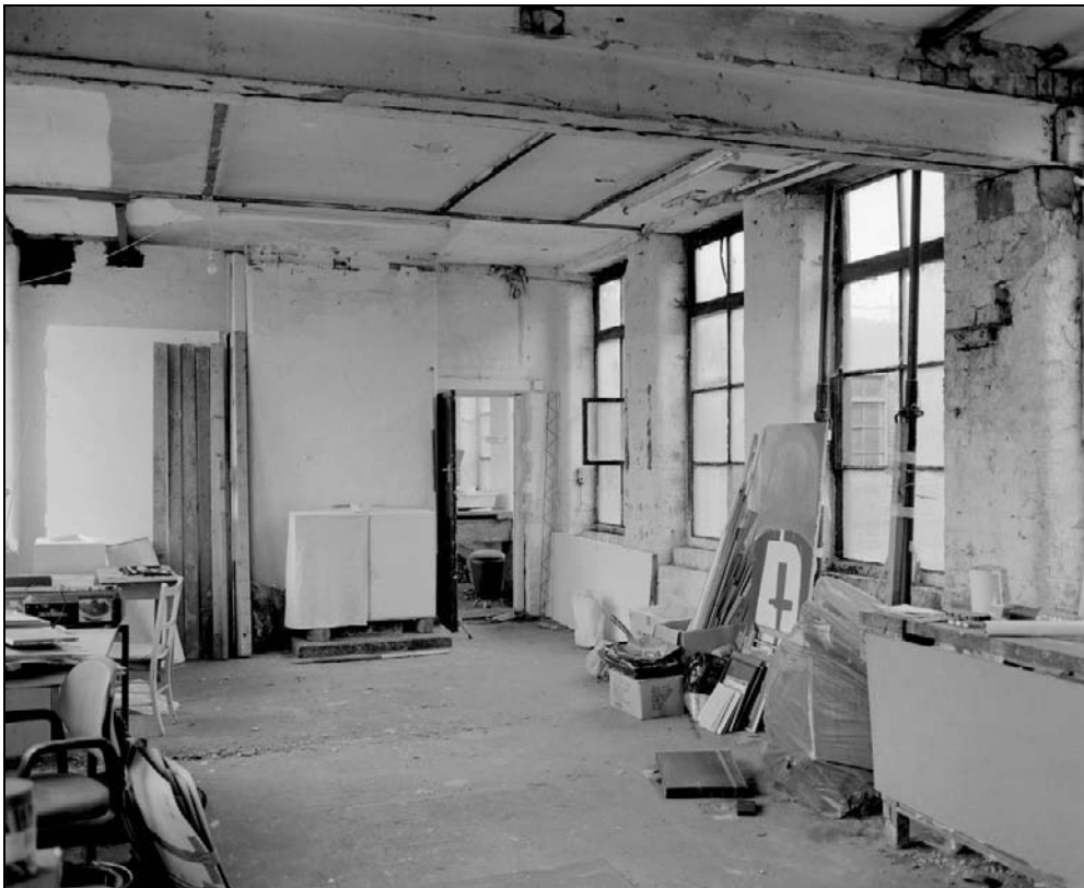
Plate 334: General view of F5, east range – note inserted doorway to F6 and blocked fireplace (film 36.6)
