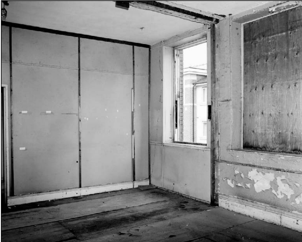
Plate 137: General view of F13, showing removed partition (film 30.7)
