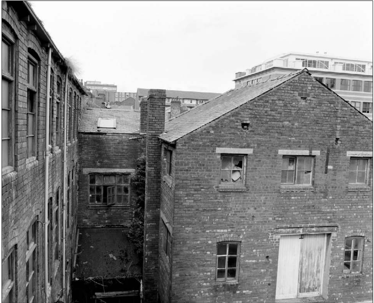
Plate 340: General view of the south and west elevation of the north range – note relationship with west range extension (film 12.5)
