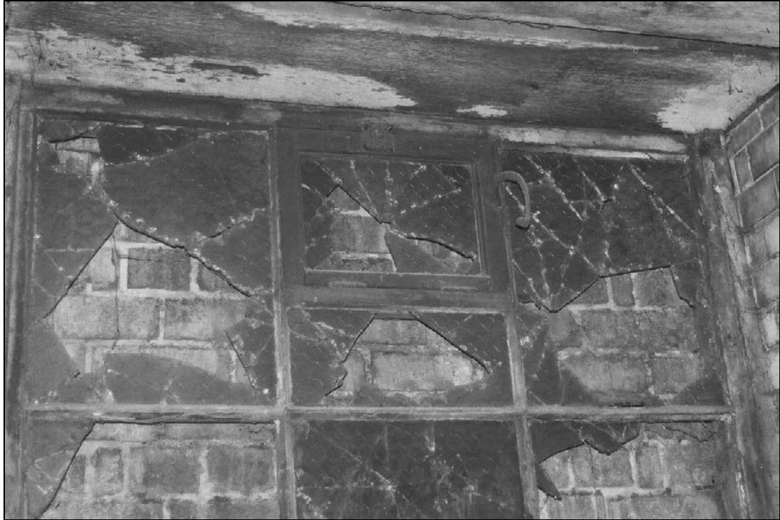
Plate 90: Detail of blocked lightwell window, B3, west range (film 2.1)
