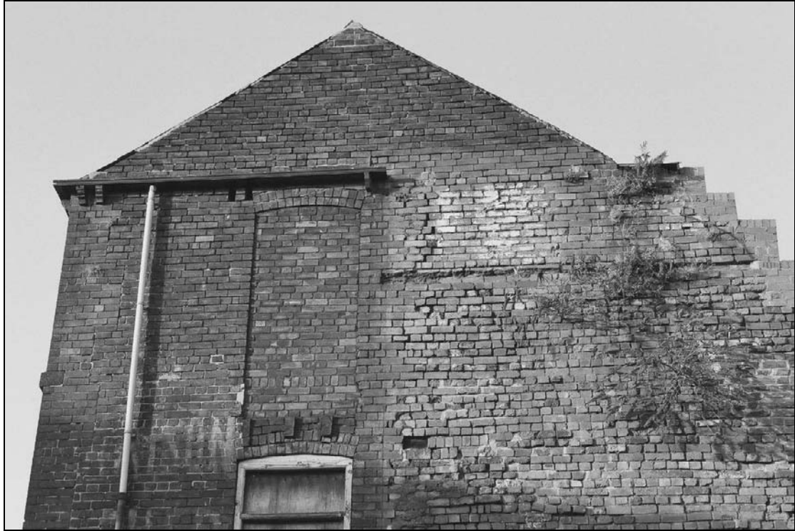
Plate 22: Detail of south gable of the west range showing 2 nd floor blocked window/door (film 46.31)
