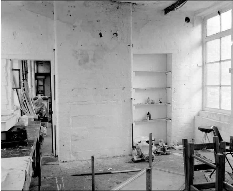
Plate 331: View of north wall of F6, east range, showing blocked primary door, inserted door and central blocked fireplace (film 36.1)
