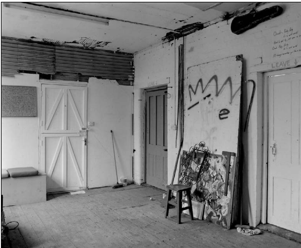
Plate 286: General view of east end of F9, south range, showing inserted partition and doorways leading to external staircase and F6, east range (film 34.8)
