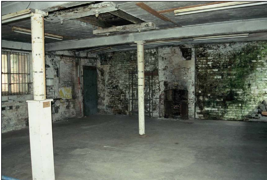
Plate 379: General view of F4, north range – note blocked window, stair scar and fireplace (film C/S 2.10)
