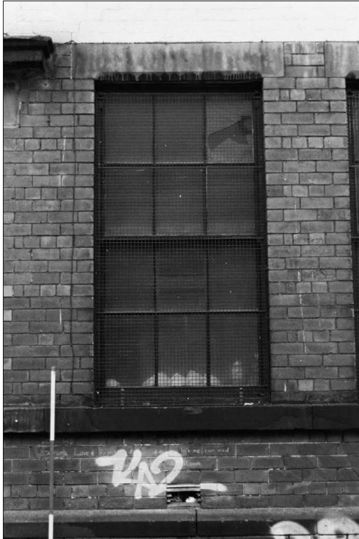
Plate 12: Detail of type 1 window, west elevation of west range (film 1.21)
