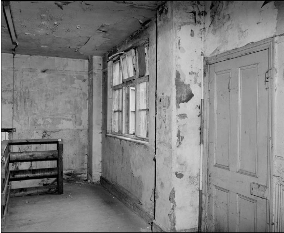
Plate 172: General view of F3 showing original doorway from F1, extension with type 25 window and inserted staircase (film 32.8)
