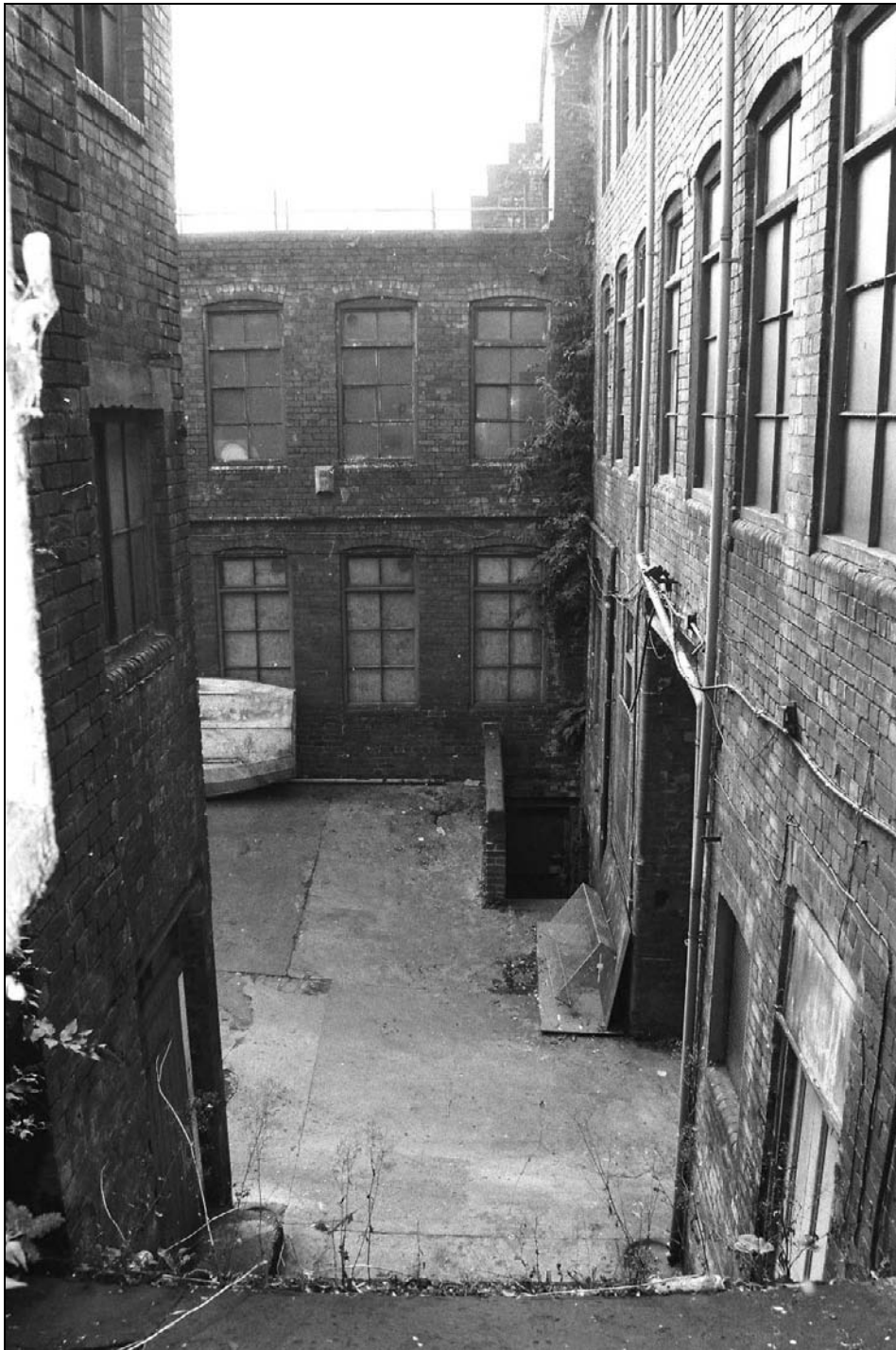
Plate 221: View across central yard from F3 towards north elevation of south range (west end) – note external staircase leading to basement (film 24.12)
