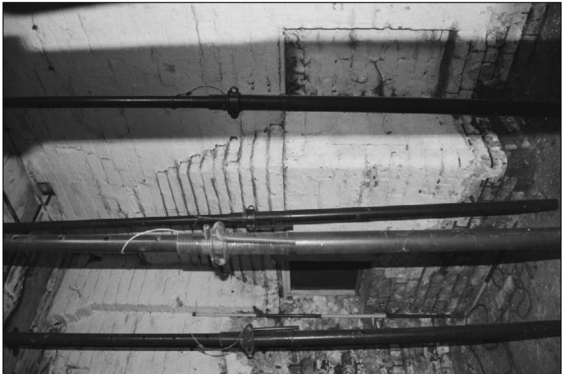
Plate 259: Detail of hand forge and adjacent blocked opening, west wall of G17 south range (film 22.9)
