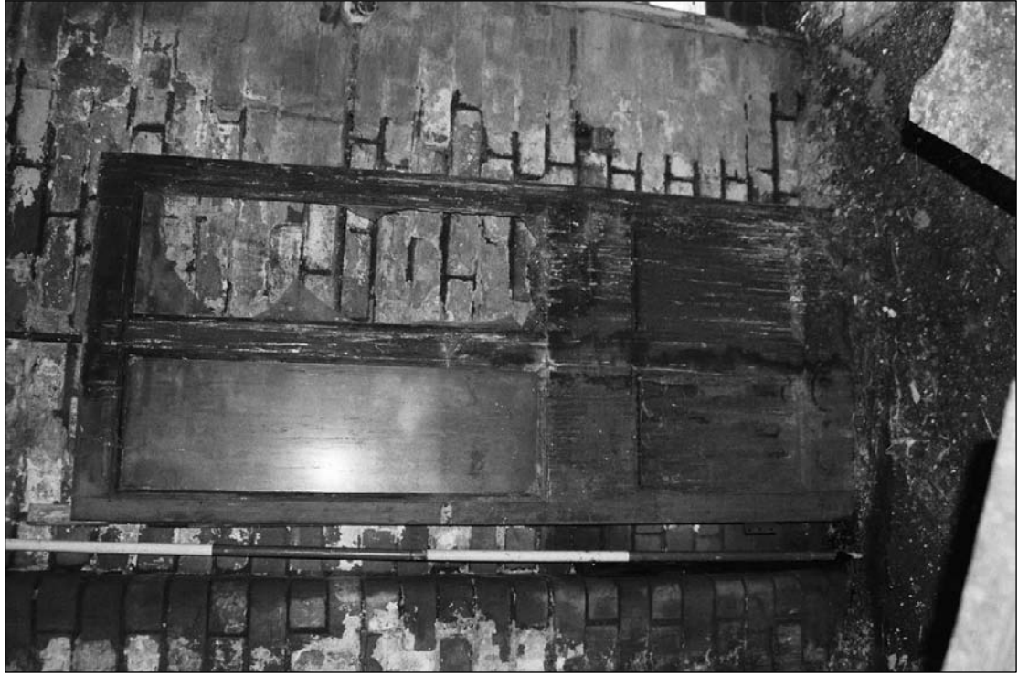
Plate 194: Detail of removed door, S2 (film 41.5)
