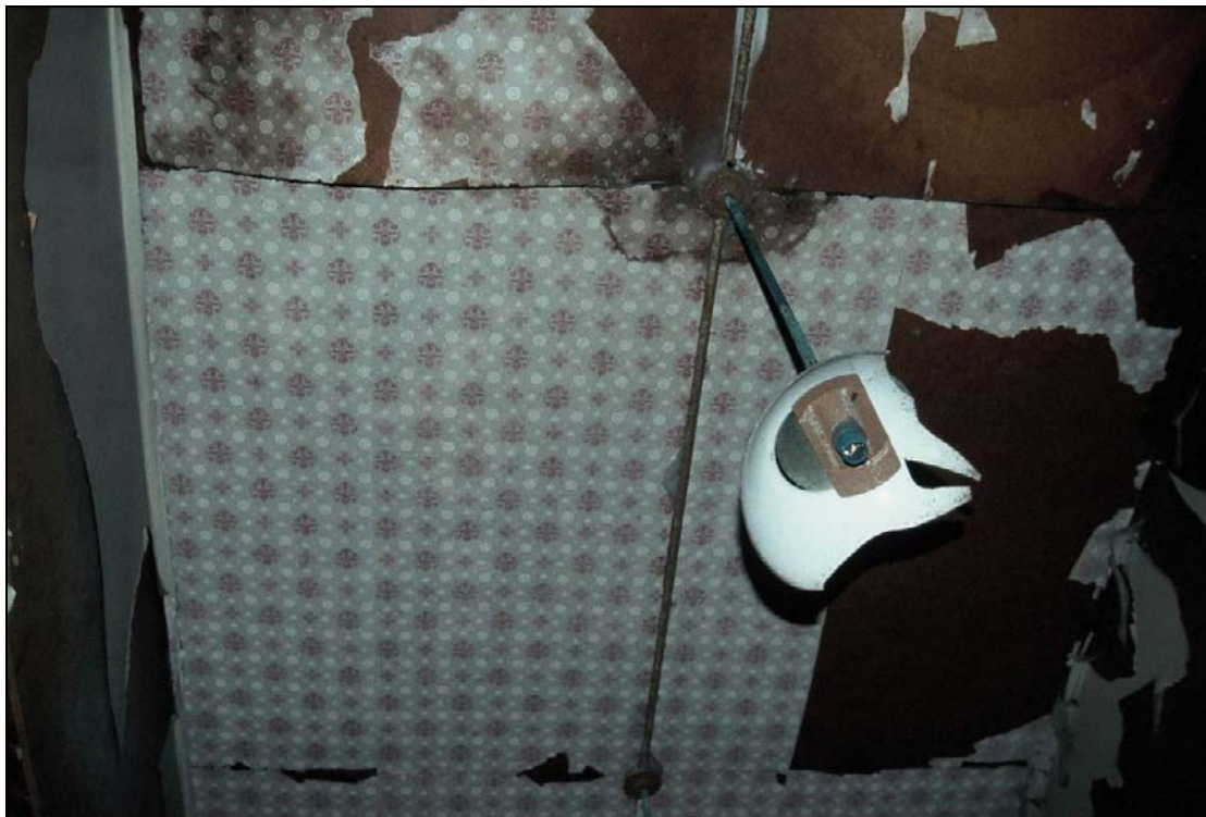
Plate 190: Detail of lighting within S1 and papered ceiling (film C/S 1.21)
