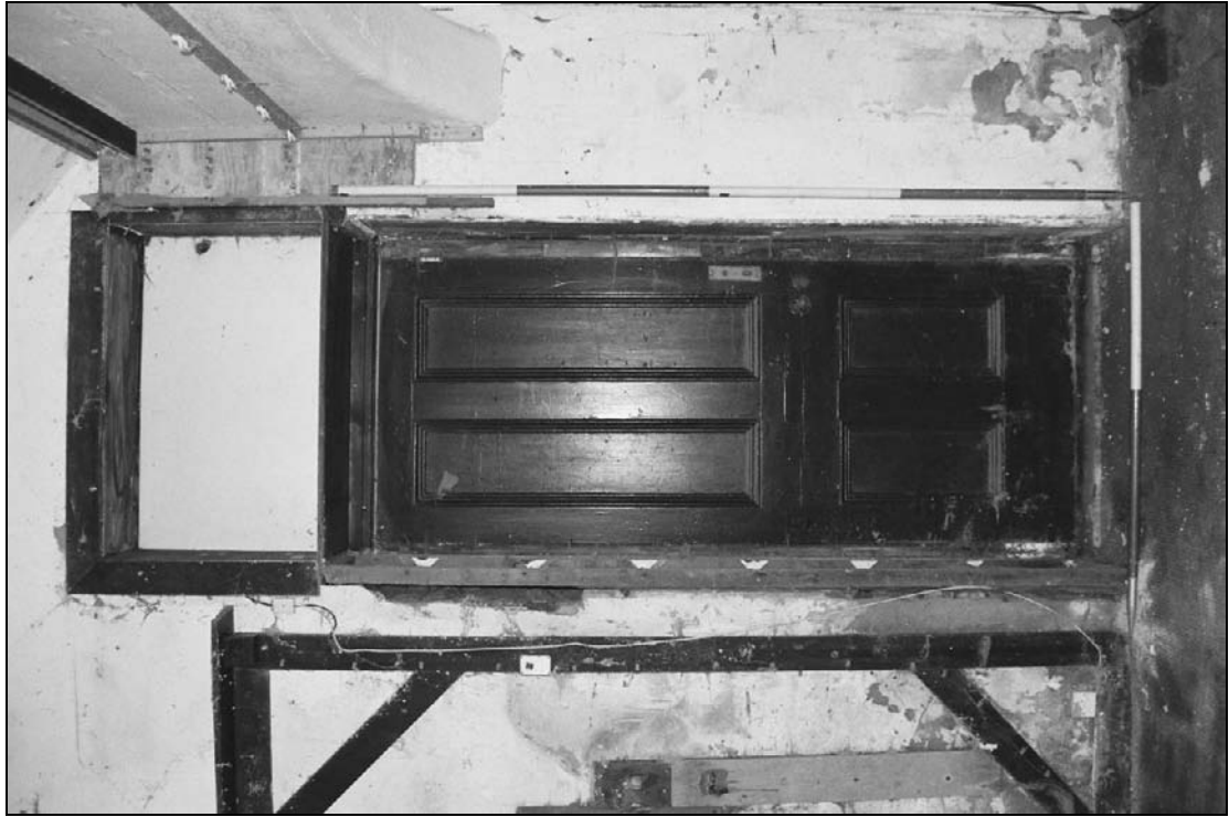
Plate 105: Detail of inserted doorway within former window opening, east wall of G2, west range (film 22.33)
