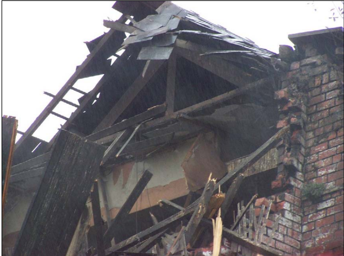
Plate 218: Detail of roof structure of king-post without diagonal braces, west range (film D.16)
