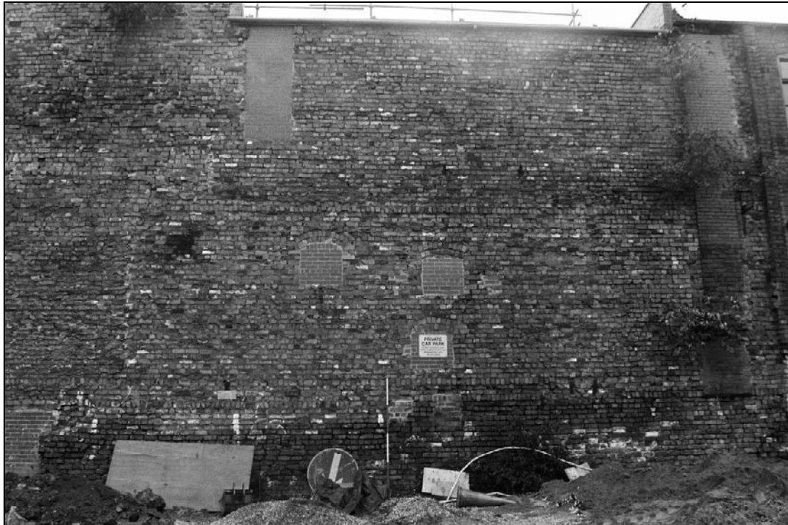
Plate 27: View of south elevation of the south range (west end) (film 1.13)
