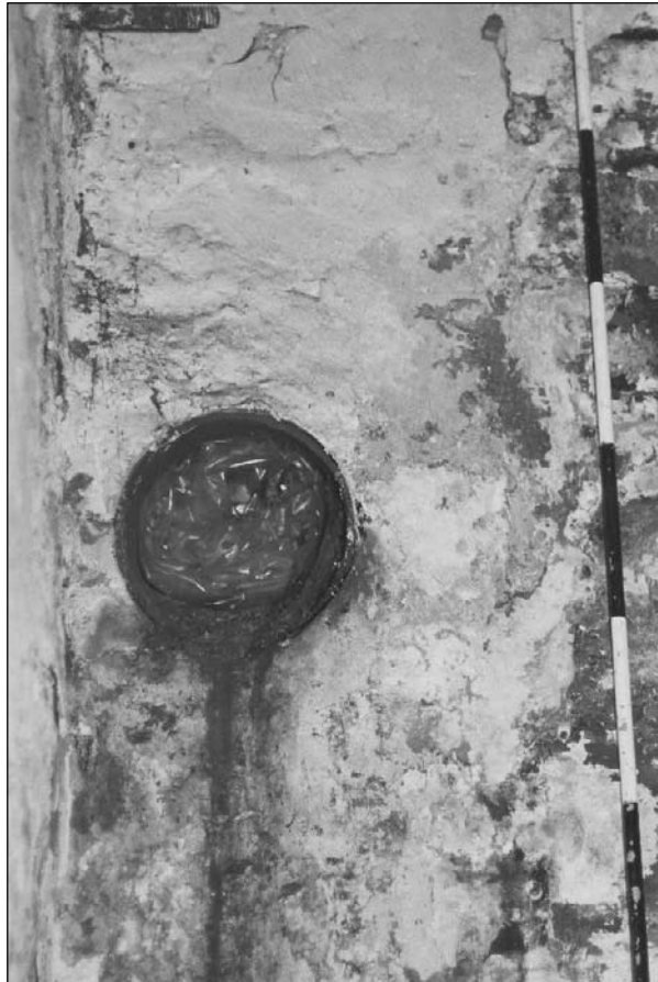
Plate 372: Detail of flue, northeast corner of G6, north range (film 42.27)
