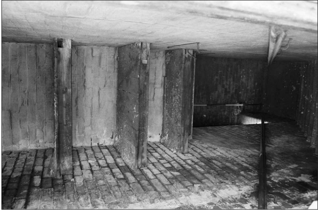
Plate 179: View down staircase to F11 from S6/roof of south range (film 28.26)
