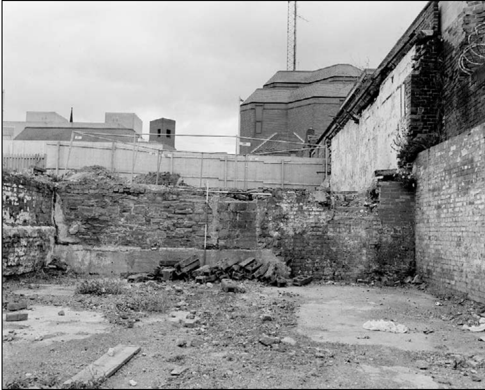
Plate 48: View of lower section of west elevation of machine shop showing height of internal floor level (film 49.7)
