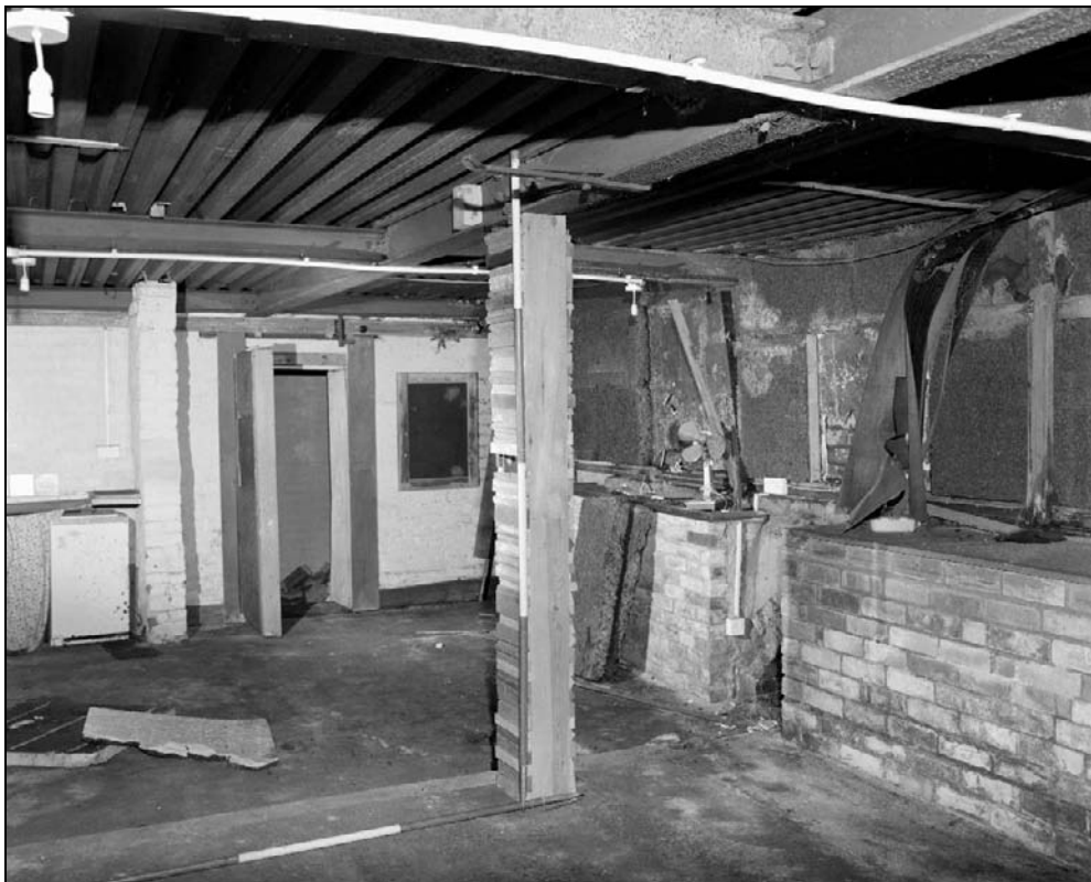
Plate 229: General view of room B5, south range (film 7.7)
