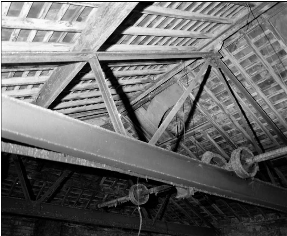
Plate 395: Detail of roof structure and line shafting, S5, north range (film 45.10)
