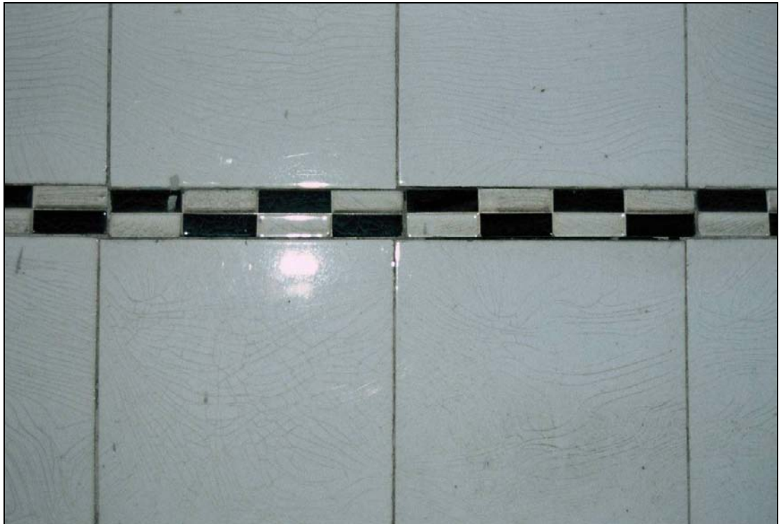
Plate 451: Detail of black and white tiles, G13, wash house (film C/S 4.6)
