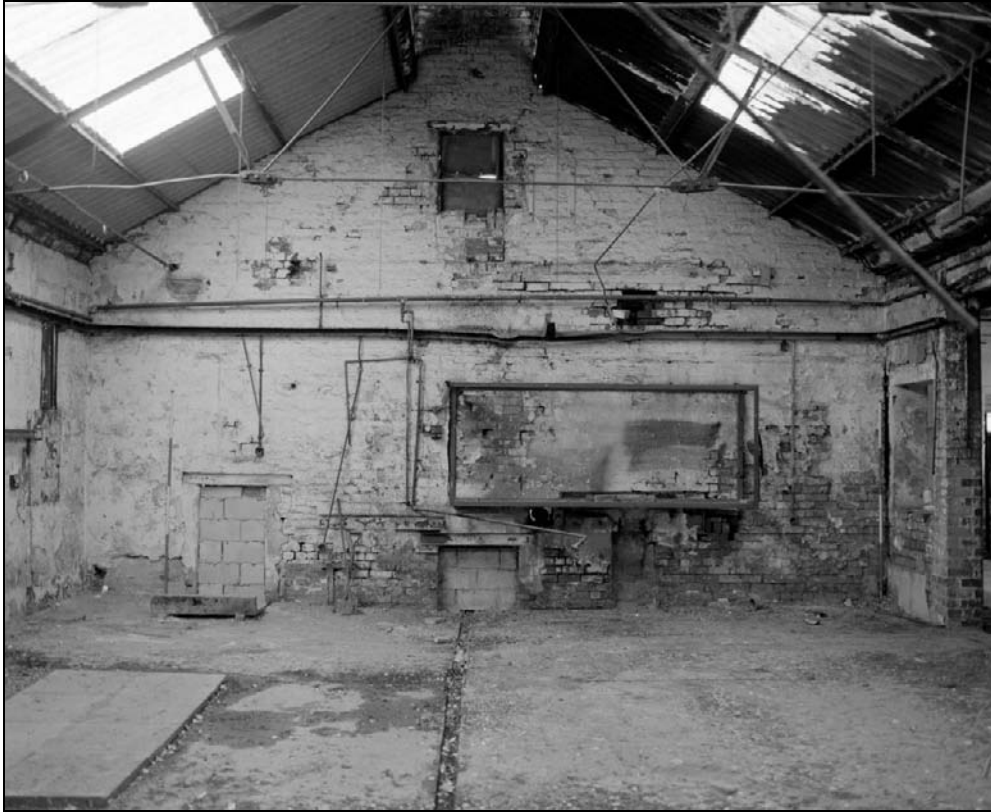
Plate 409: Detail of west wall of G15, machine shop, showing blocked openings and upper gable boarded window (film 19.6)
