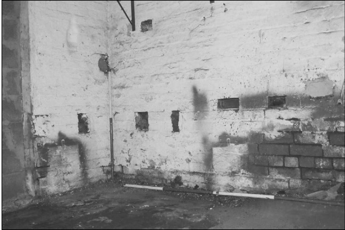
Plate 370: Detail of sockets in north wall of G6, north range (film 42.29)
