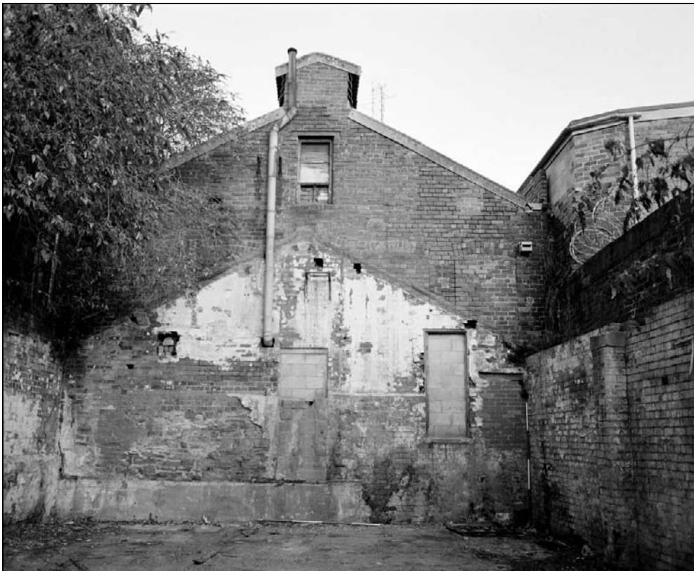
Plate 47: General view of west elevation of machine shop (film 48.9)
