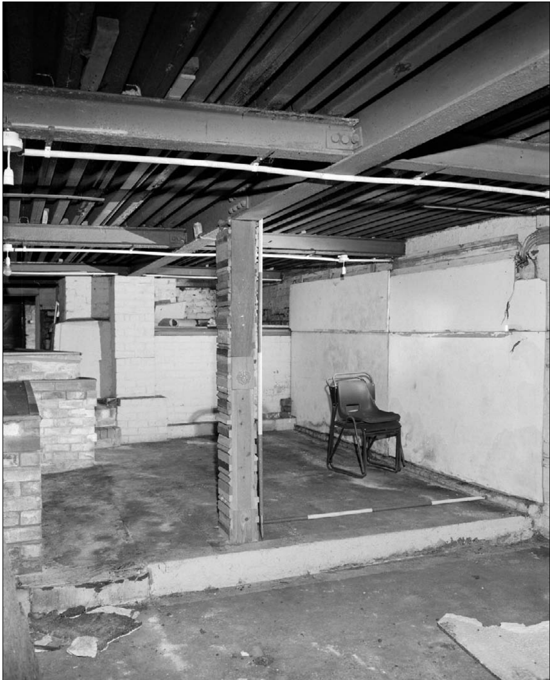
Plate 230: General view of B5 – note inserted ceiling (film 7.6)
