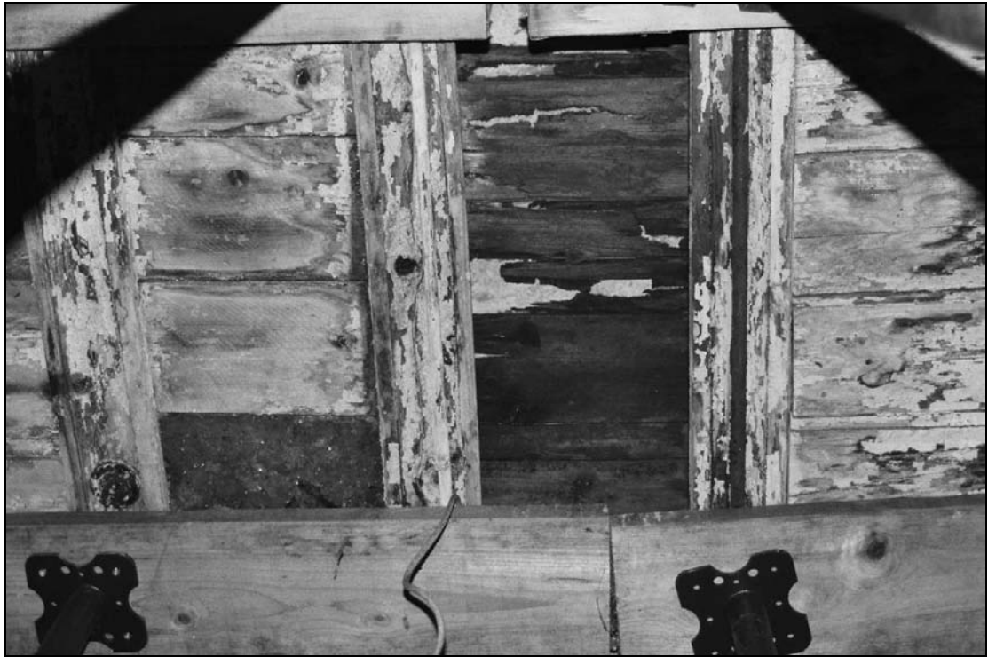
Plate 263: Detail of ceiling construction, G17 south range (film 22.5)
