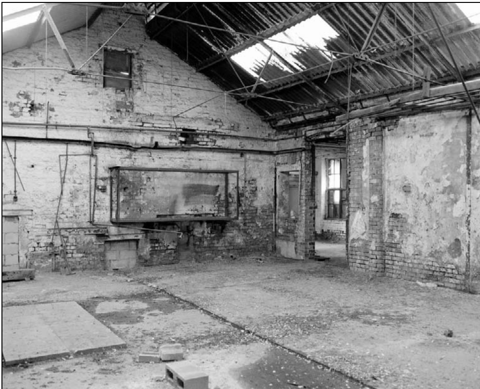
Plate 408: General view of G15, machine shop – note inserted doorway from G16, south range (film 19.7)
