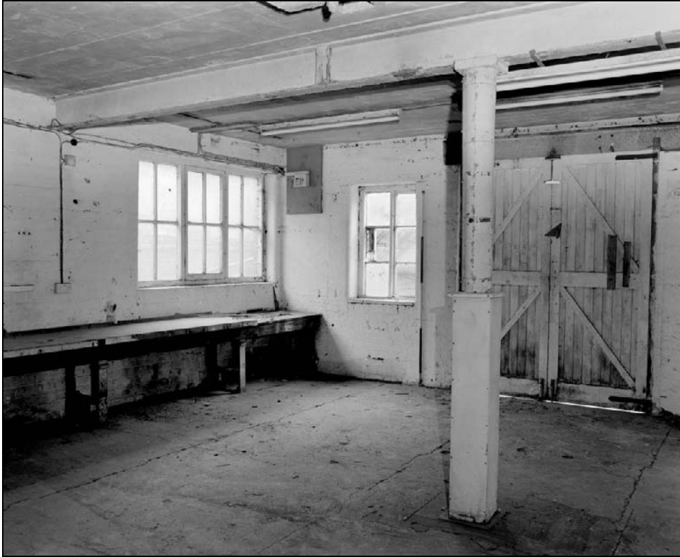
Plate 376: General view of F4, north range – note workbench, column and loading door (film 33.2)
