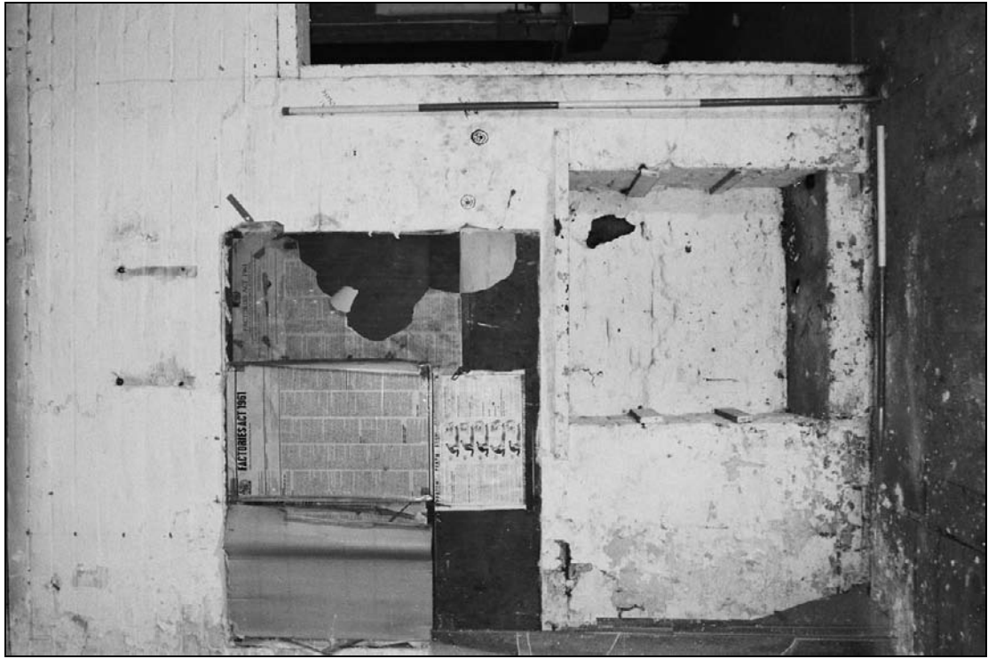
Plate 252: Detail of altered fireplace, west wall of G19, south range (film 21.33)
