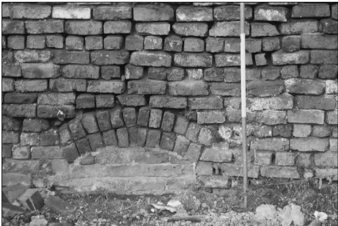
Plate 30: Detail of blocked primary opening within early section of wall, south elevation of south range (film 46.29)
