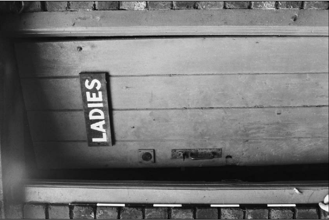
Plate 454: Detail of timber planked door, G14 privies, wash house range (film 23.19)
