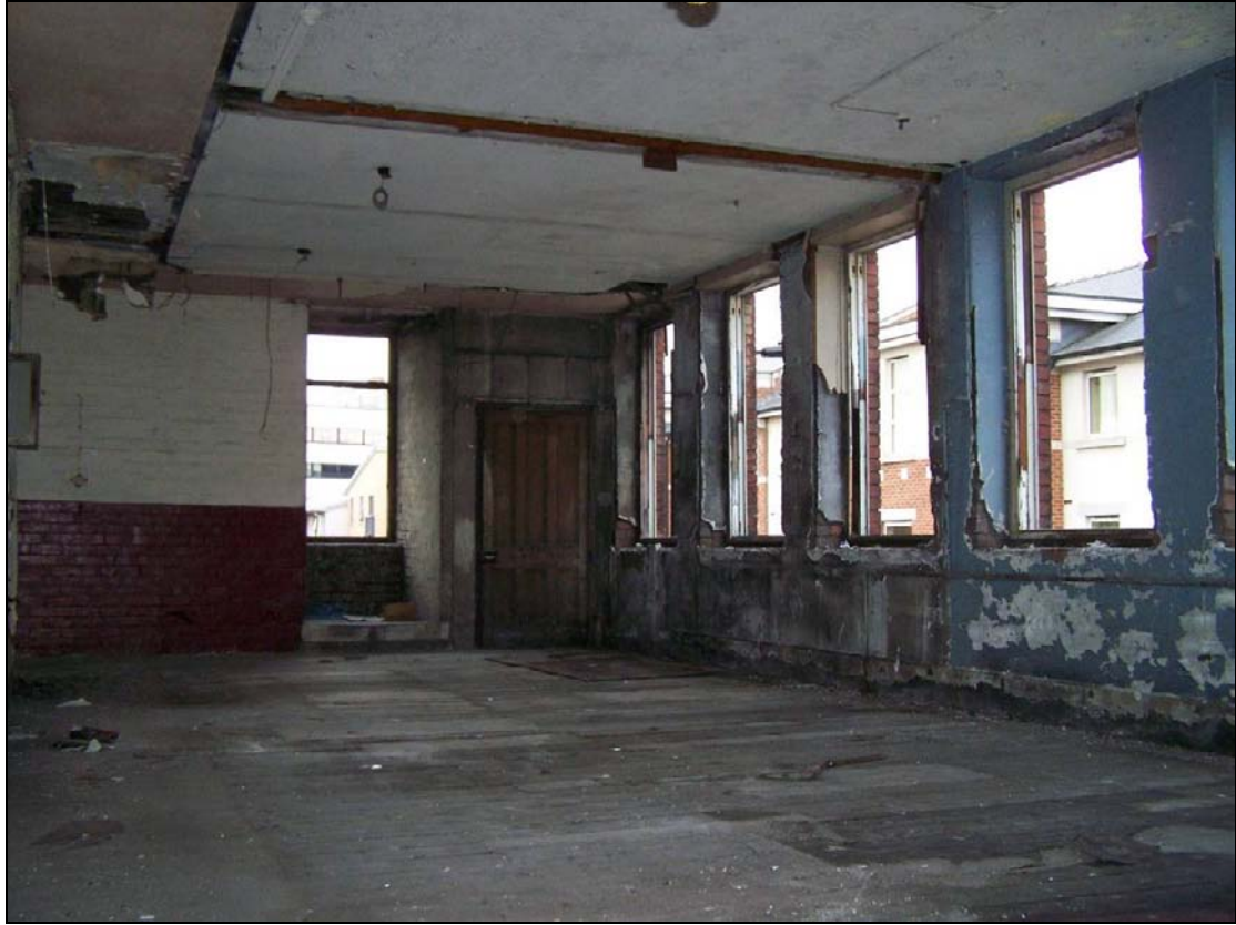
Plate 145: View of rooms F11-F16 & F18 after removal of partitions (film D.3)
