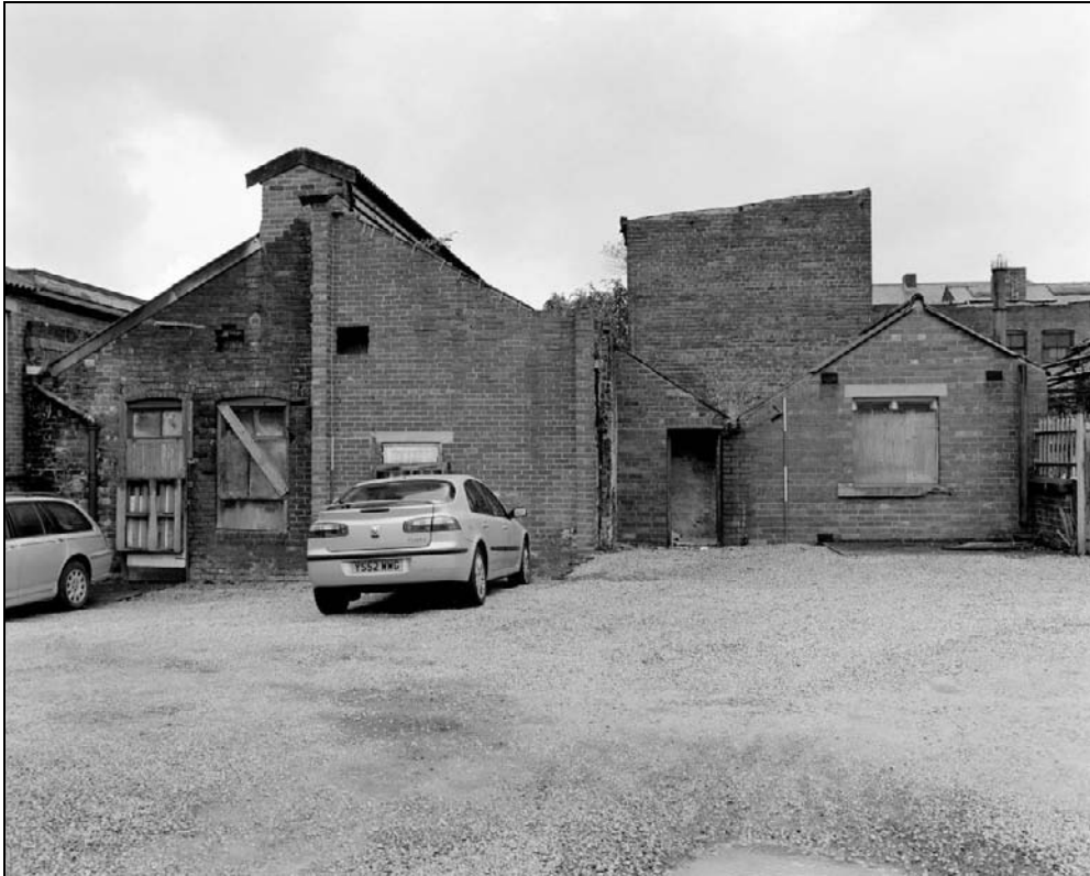
Plate 53: General view of the east elevations of the machine shop and wash house range (film 5.7)
