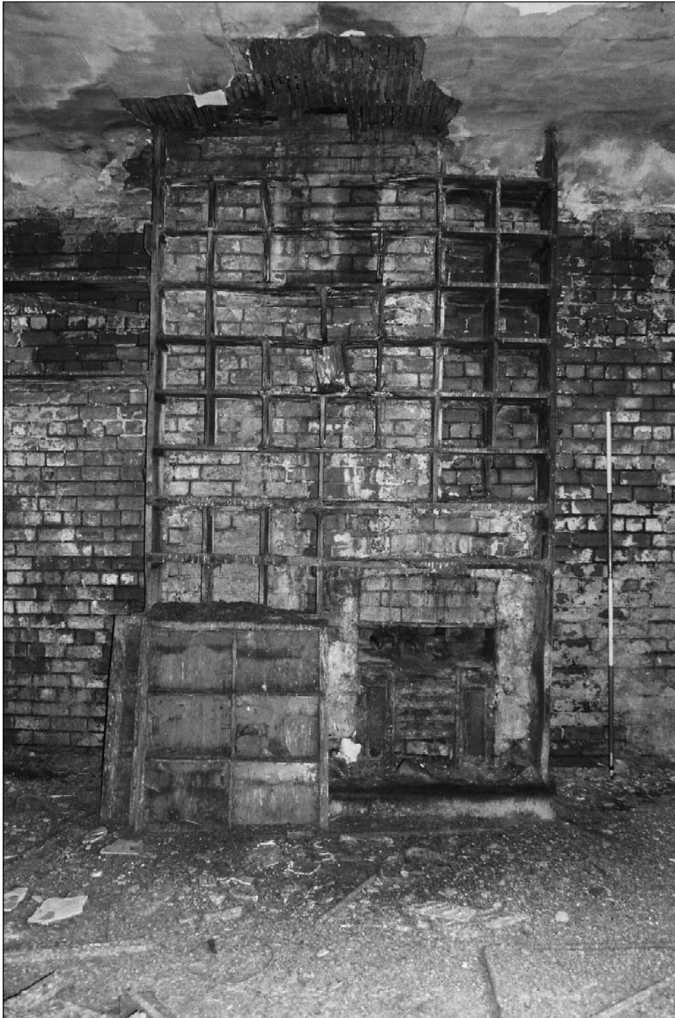
Plate 203: Detail of fireplace and timber shelving (film 41.33)
