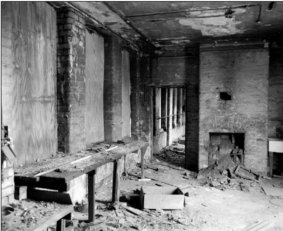
Plate 299: General view of F8, south range (east end) – note workbenches and fireplace (film 35.6)
