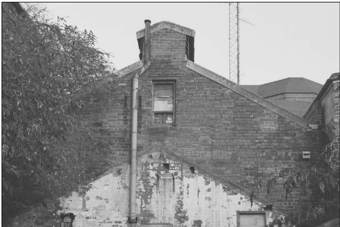
Plate 52: Detail of raised ridge louvered roof and upper window, west elevation of machine shop (film 46.8)
