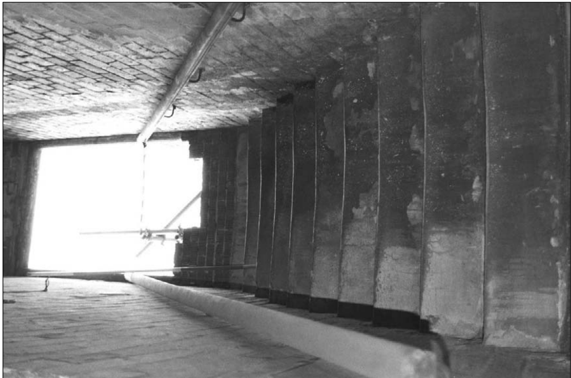
Plate 178: View up staircase from F11 to S6/roof of south range (film 26.25)
