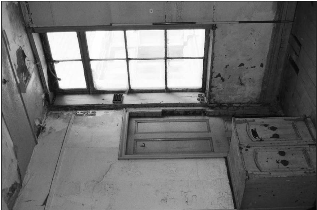
Plate 165: Detail of northeast corner of room F1, showing type 5 window (film 25.27)
