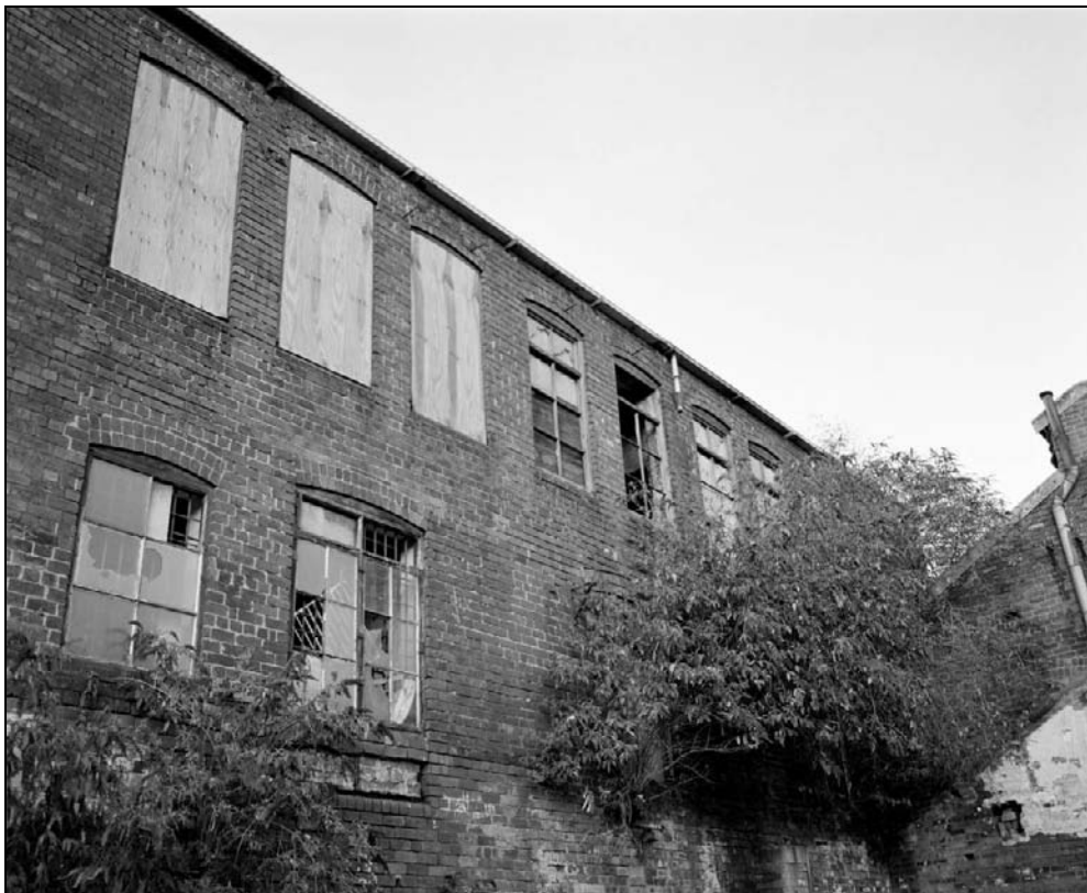
Plate 39: Detail of windows, south elevation of south range (east end) (film 48.7)
