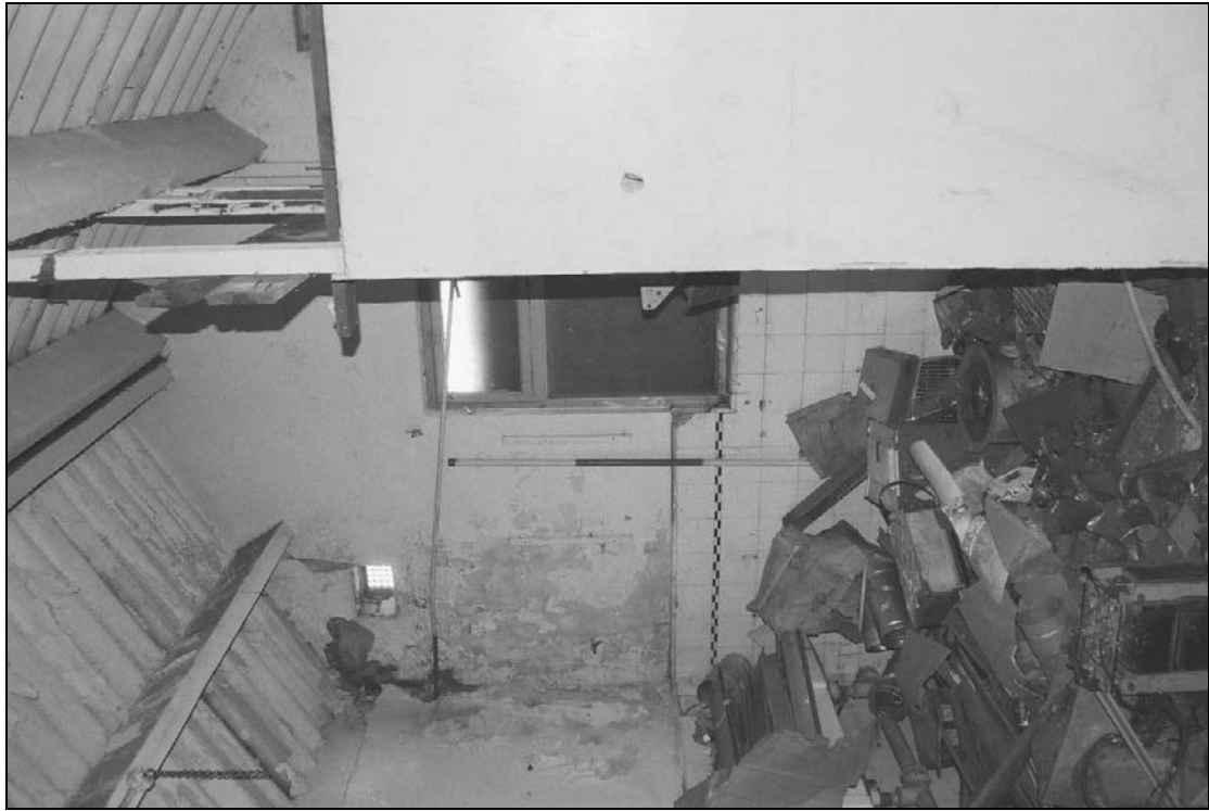
Plate 446: General view of G13, wash house (film 44.4)
