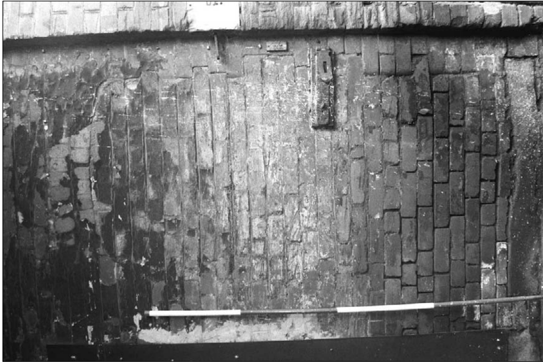
Plate 76: Detail of blocked door, south side of cart passage, west range (film 1.2)
