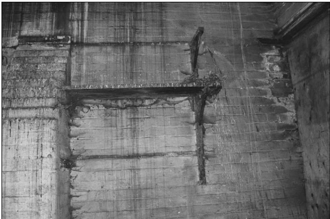
Plate 206: Detail of flue and shelves, south wall of S3 (film 41.26)
