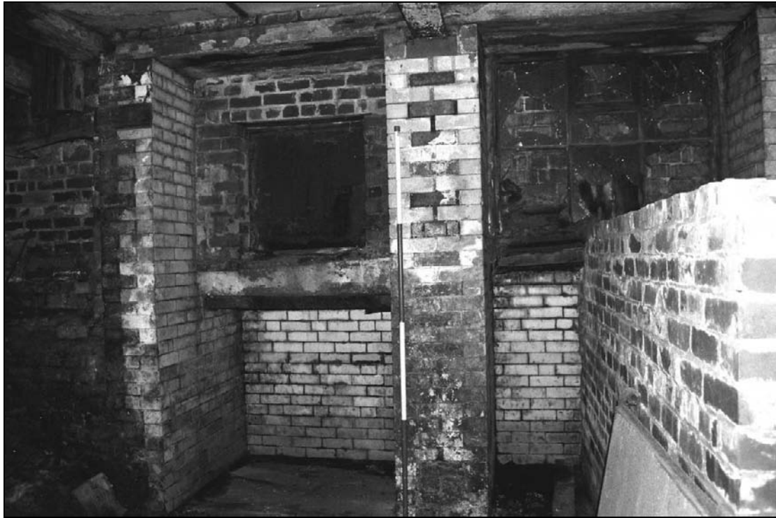
Plate 86: Detail of glazed brickwork and coal chute and blocked lightwell, B3 west range (film 3.35)
