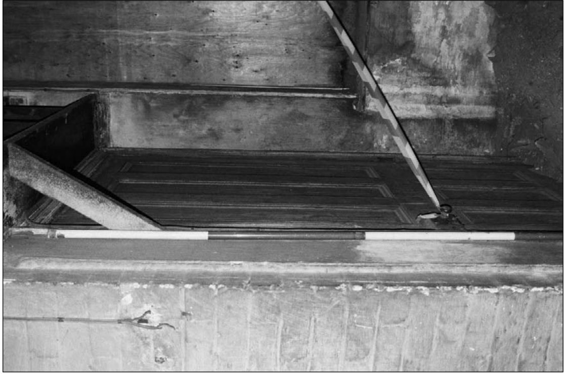
Plate 132: Detail of lift door, F11, west range (film 26.26)
