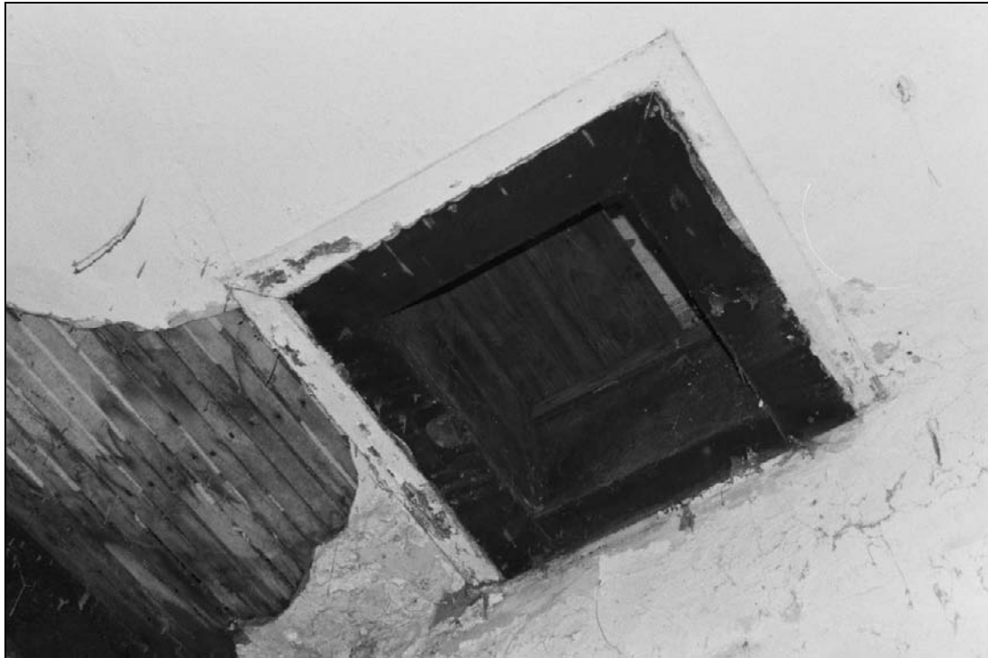
Plate 109: Detail of inserted hatch within ceiling of room G2, west range (film 22.27)
