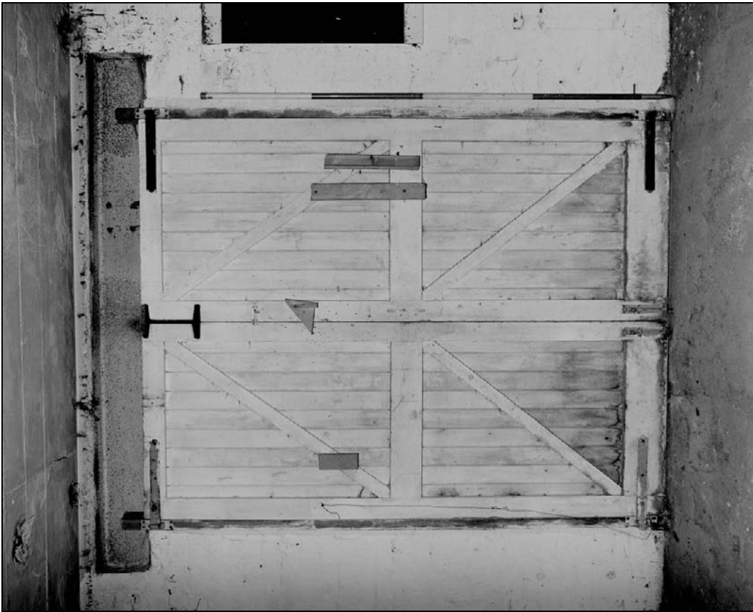
Plate 382: Detail of inserted loading door, south wall of F4, north range (film 33.7)
