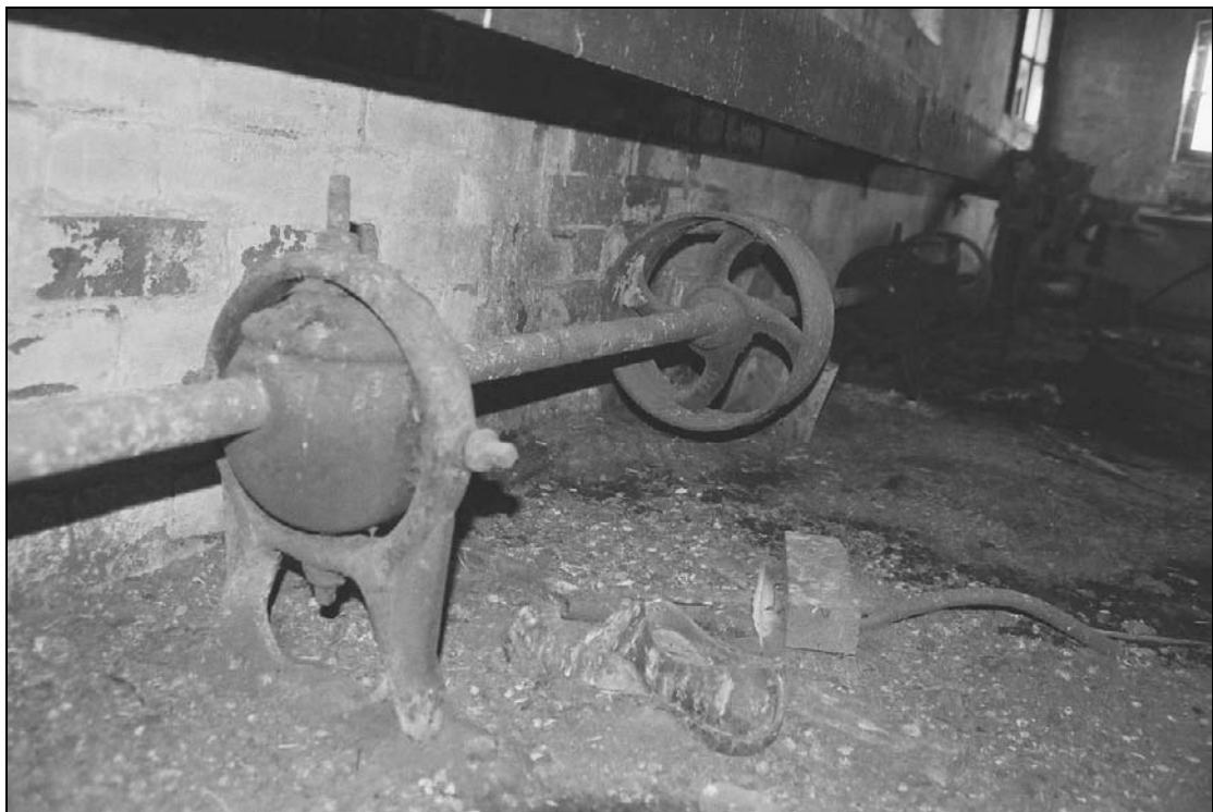
Plate 401: Detail of line shafting, S5 (film 44.13)
