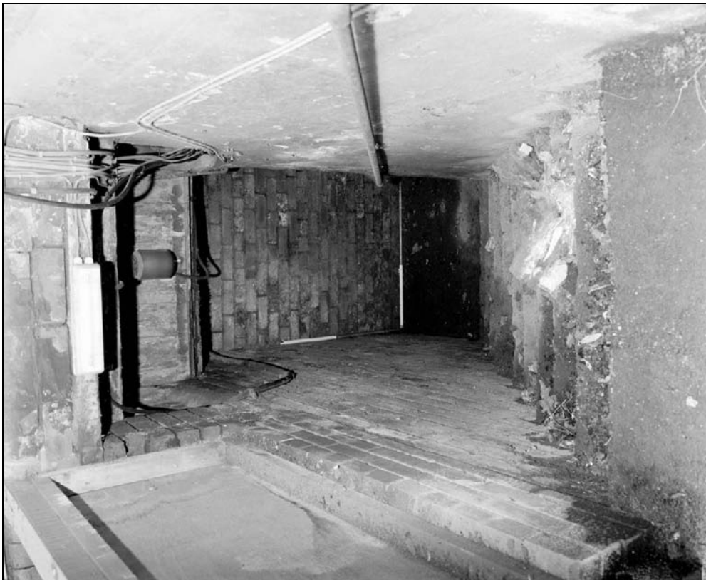
Plate 239: View down external staircase from central yard to B7 (film 8.6)
