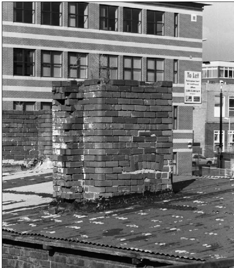
Plate 316: Detail of truncated chimney breast from removed second floor, east range (film 28.32)
