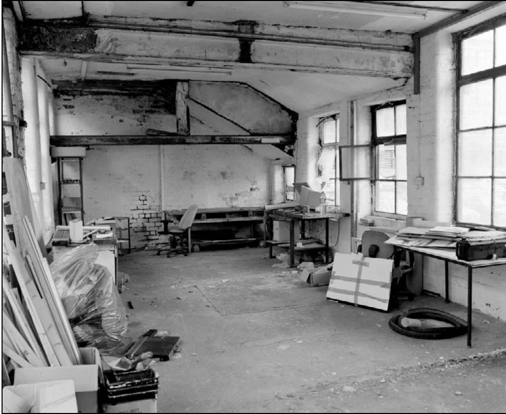
Plate 333: General view of F5, east range, showing changes in roof level (film 36.3)
