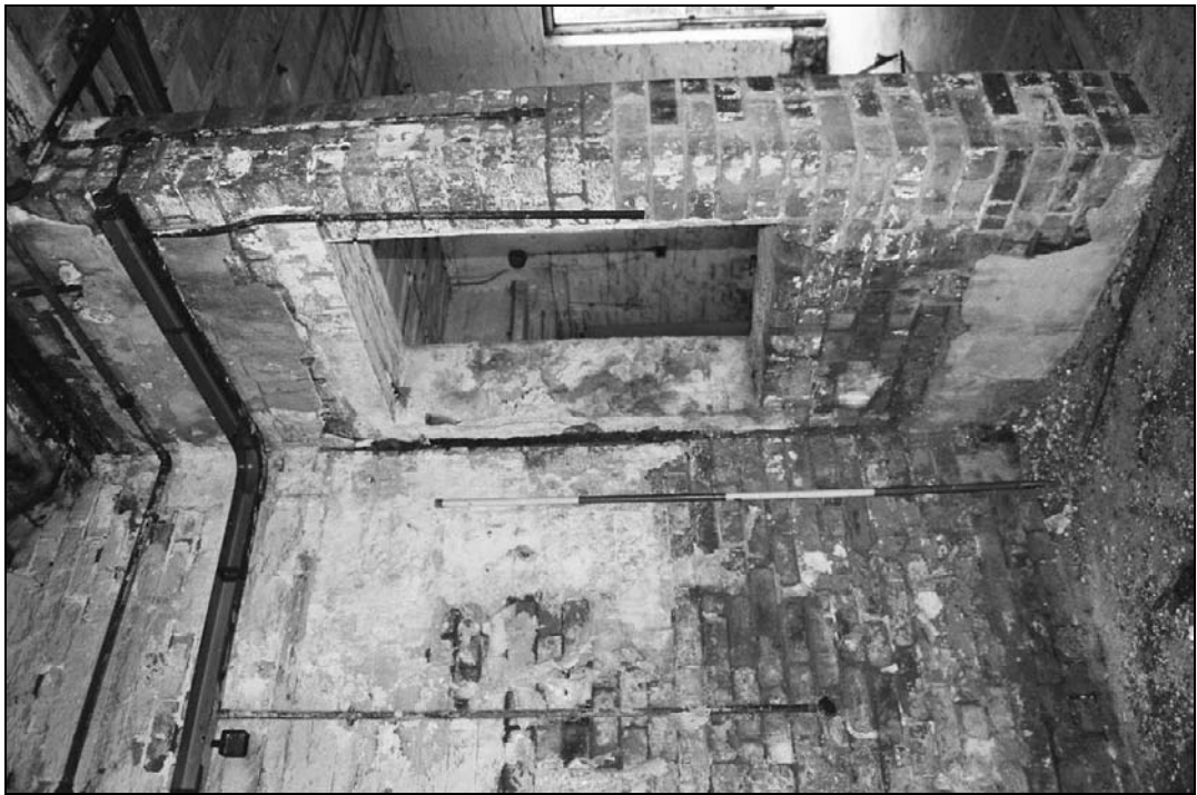
Plate 412: Detail of inserted window, northwest corner of G15, machine shop (film 23.33)
