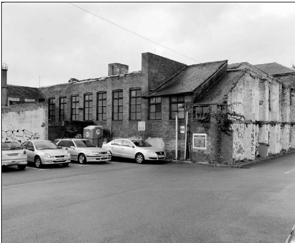
Plate 62: General view of the east and north elevation of the east range (film 5.1)
