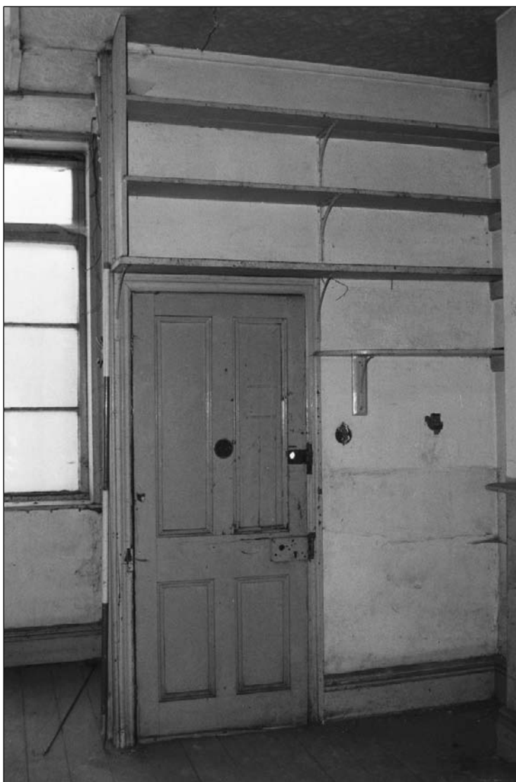
Plate 167: Detail of door and shelving, room F1 (film 25.27)
