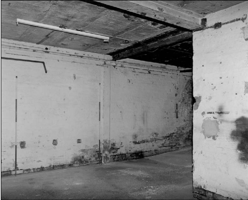
Plate 362: General view of G5, north range, showing removed wall scars (film 14.9)
