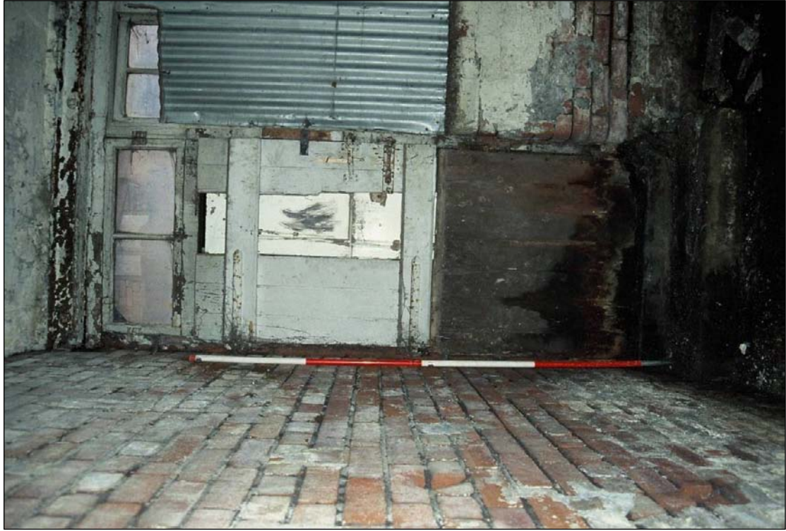
Plate 357: Detail of doorway, east wall of G4, north range (film C/S 4.24)
