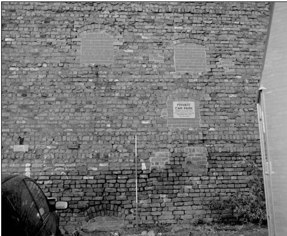
Plate 28: Detail of join between older lower section of wall and later upper section of wall and blocked arched openings, south elevation of south range (west end) (film 47.9)
