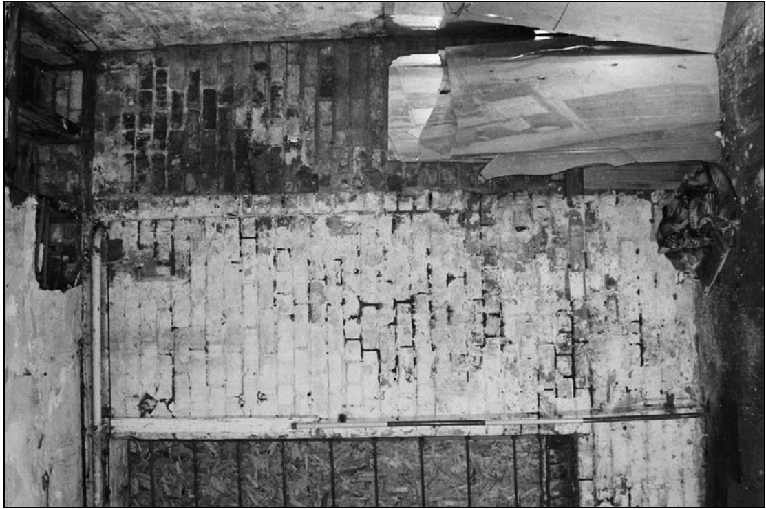
Plate 251: Detail of blocked opening southwest corner of G19, south range (film 21.31)
