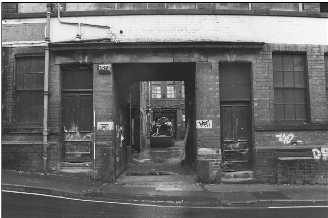
Plate 5: Detail of cart passage and flanking pedestrian doors, west elevation of west range (film 1.27)
