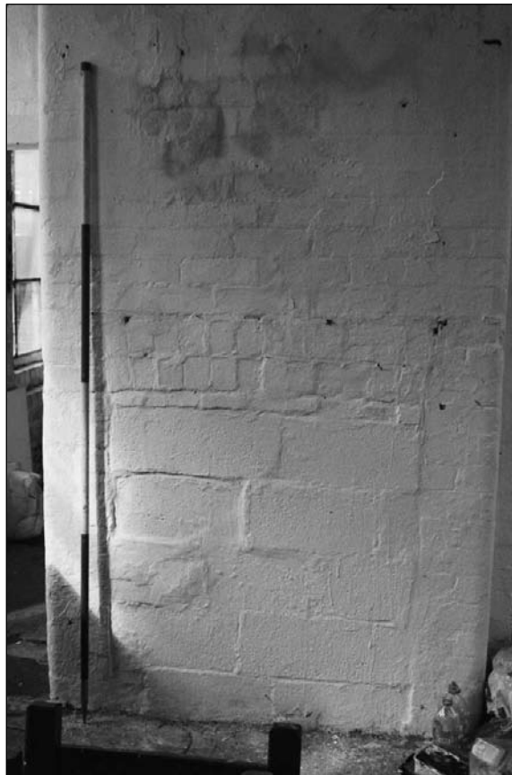
Plate 332: Detail of blocked fireplace, north wall of F6, east range (film 26.9)
