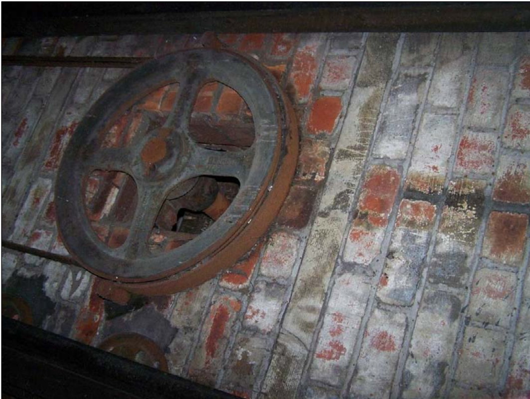
Plate 151: Detail of inserted lift mechanism within lift shaft (film D.9)
