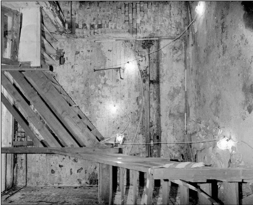
Plate 112: General view of G3, west range extension – note inserted staircase (film 13.9)
