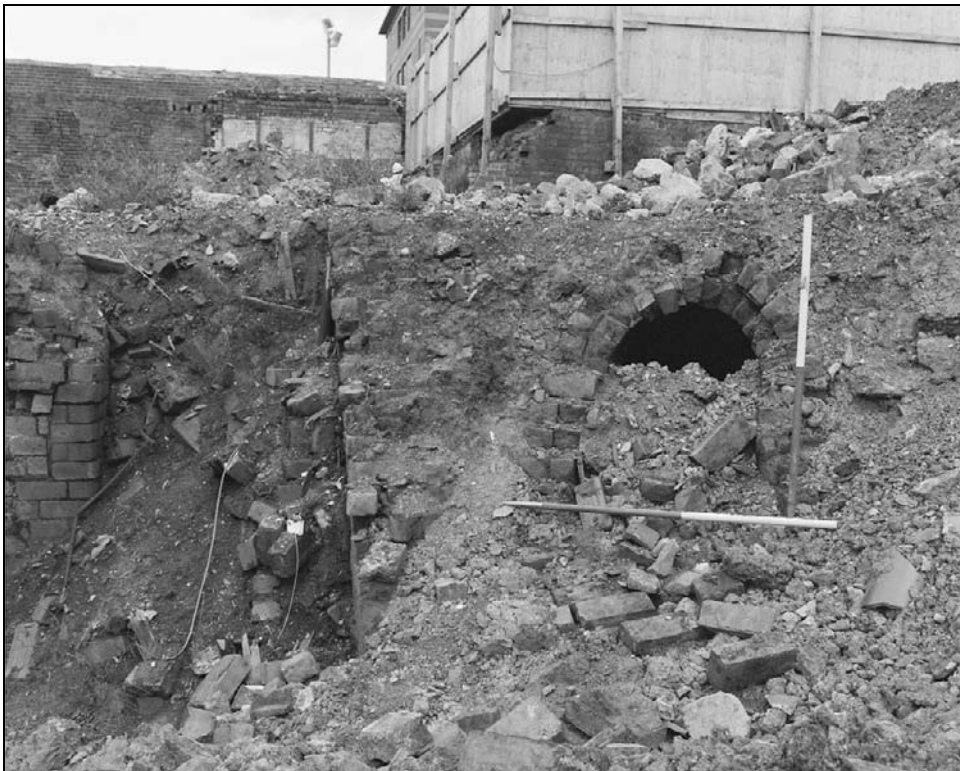
Plate 37: Detail of former passage B7 to the left and earlier flue to the right, south range (east end) (film 49.10)
