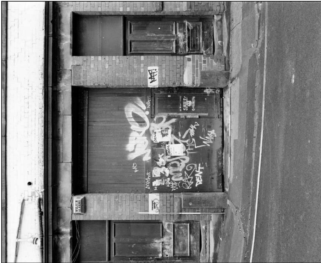
Plate 6: Detail of cart passage and flanking pedestrian doors, west elevation of west range (film 4.3)
