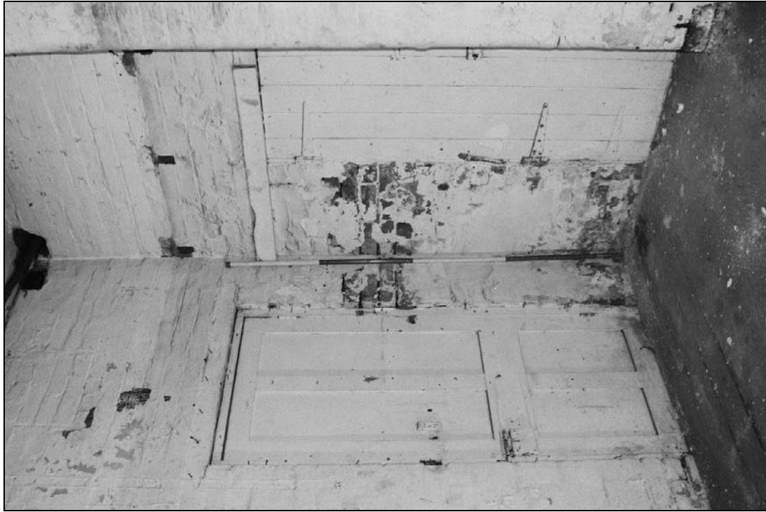
Plate 249: Detail of doorways, northeast corner of G19, south range – left door is primary leading to G8 (east range) right door is inserted (film 21.27)
