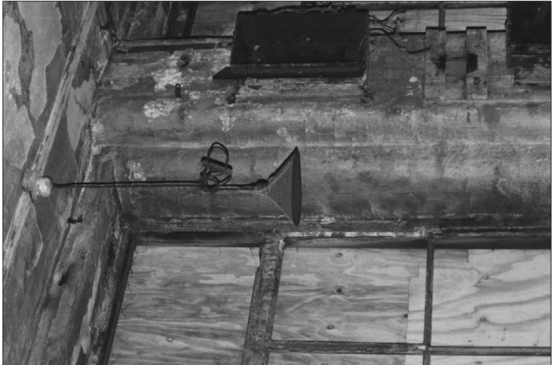
Plate 296: Detail of lamp, F7 south range (east end) (film 26.1)
