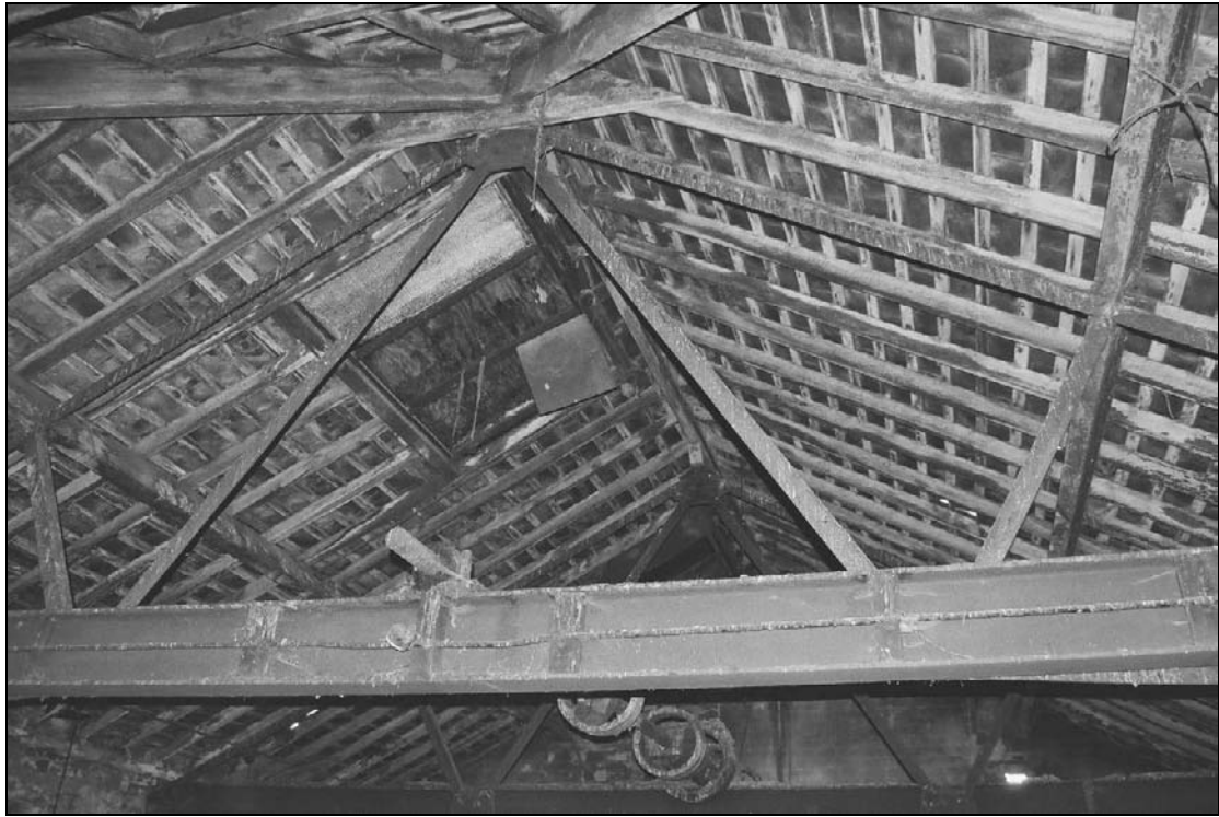
Plate 396: Detail of roof structure and line shafting, S5, north range (film 44.11)
