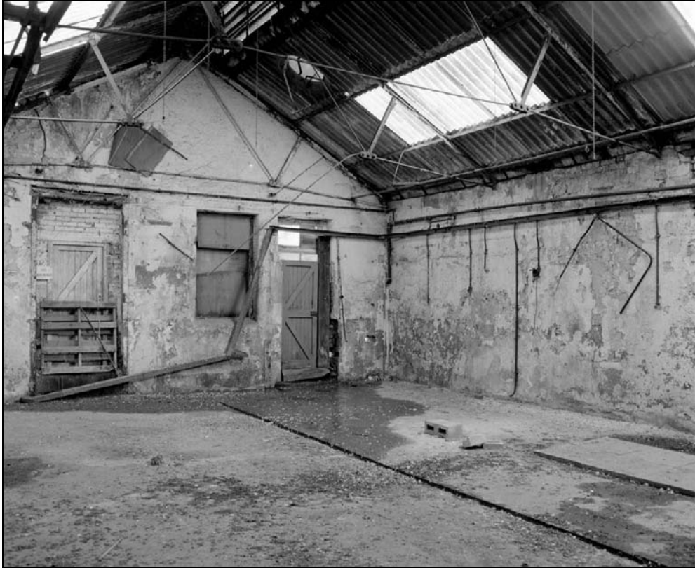
Plate 407: General view of room G15, machine shop – note inserted doorways (film 19.2)
