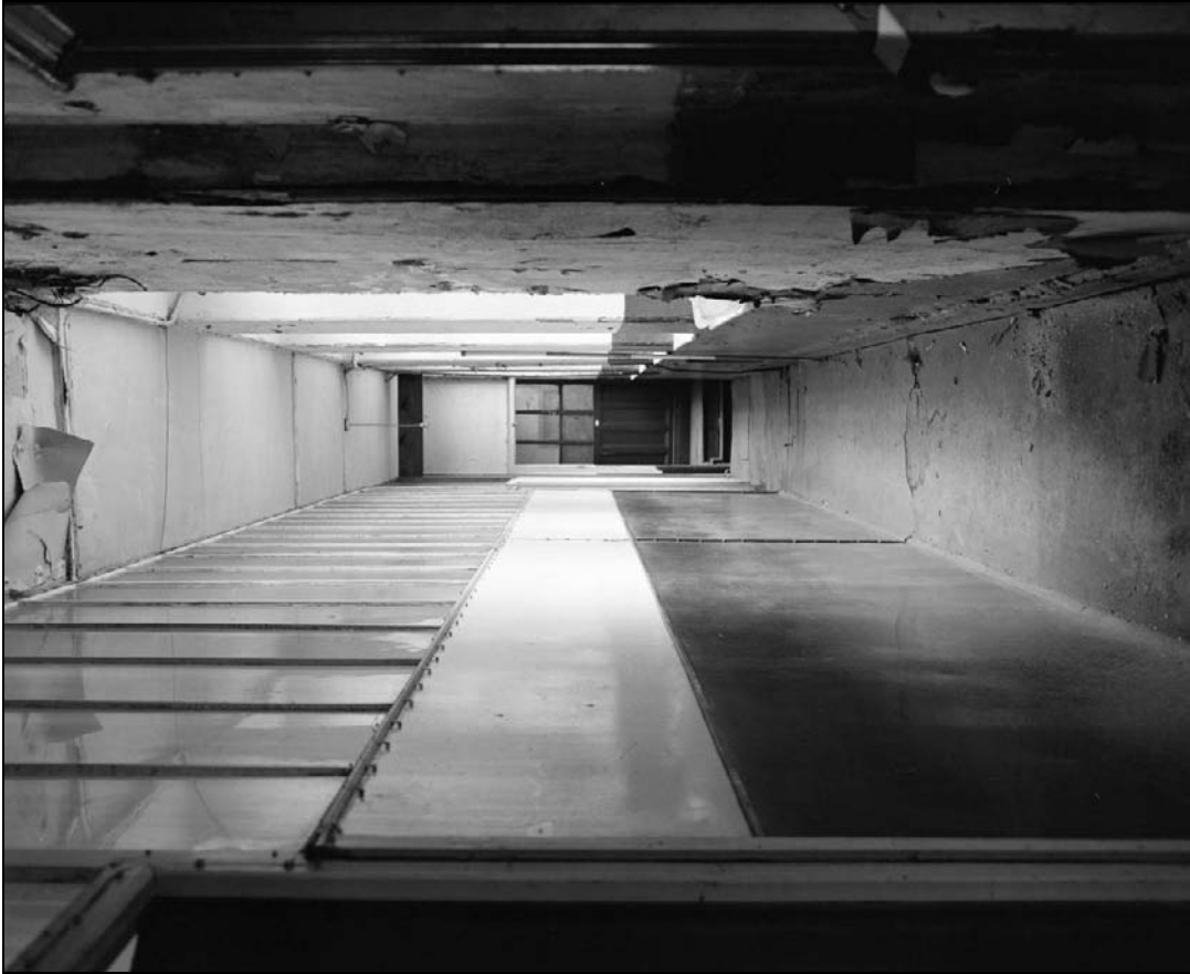
Plate 143: General view along corridor F18 (film 30.4)
