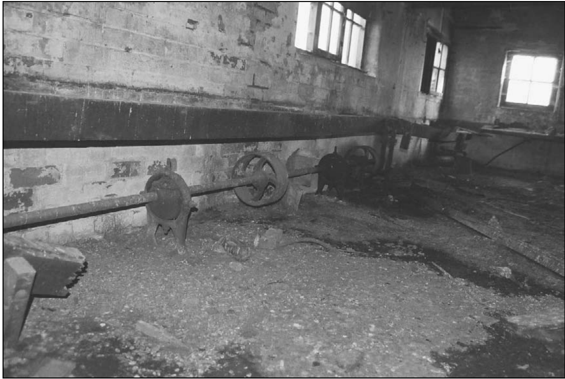
Plate 400: Detail of below line shafting, along east wall of S5 (film 44.15)
