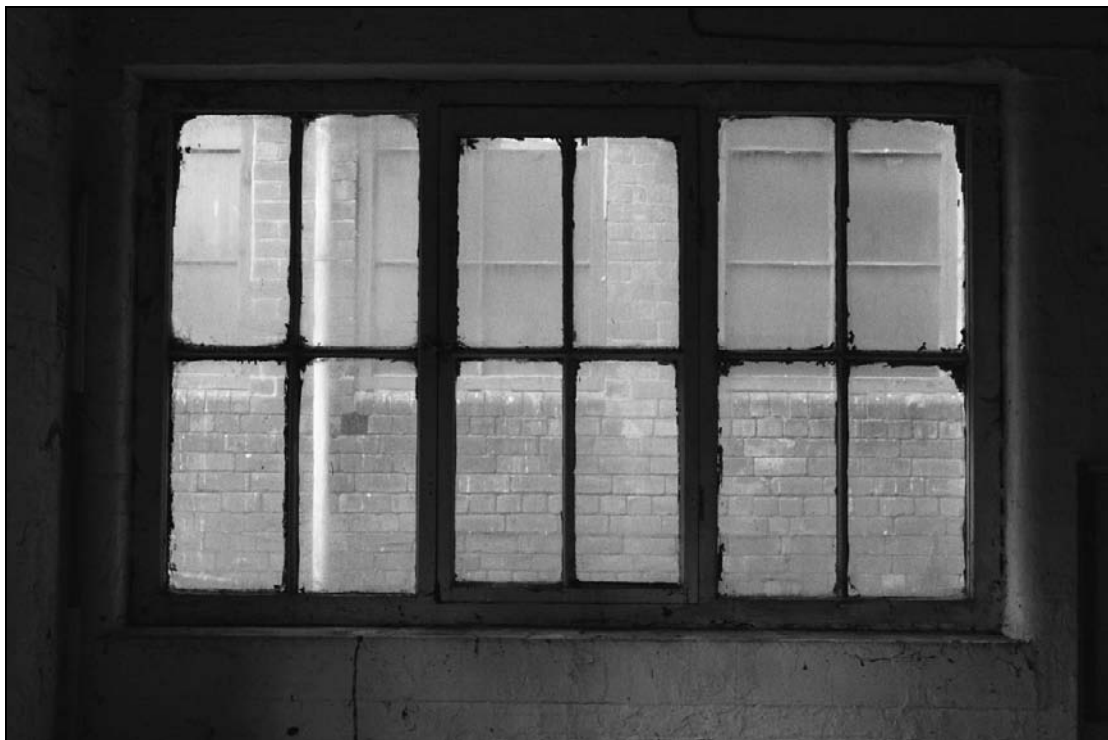
Plate 387: Detail of type 14 window, F4, north range (film 24.22)
