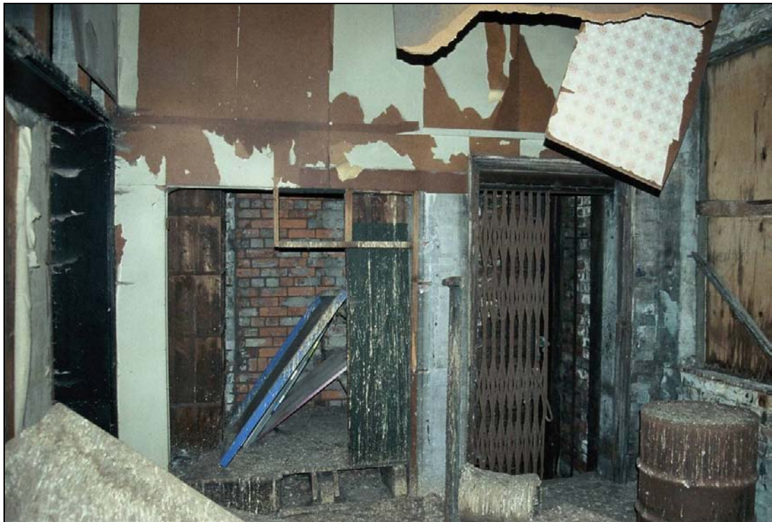
Plate 188: View of lift shaft and storage area at south end of S1 (film C/S 1.23)
