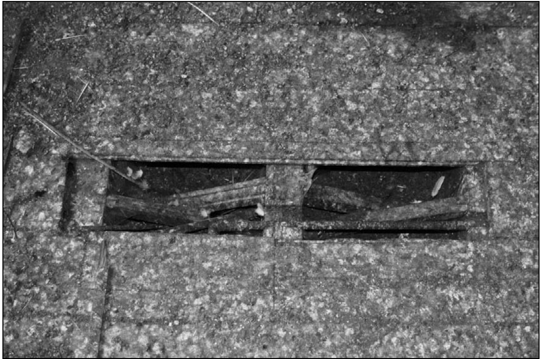
Plate 197: Detail of noggins between timber floor joists, S2 (film 41.24)
