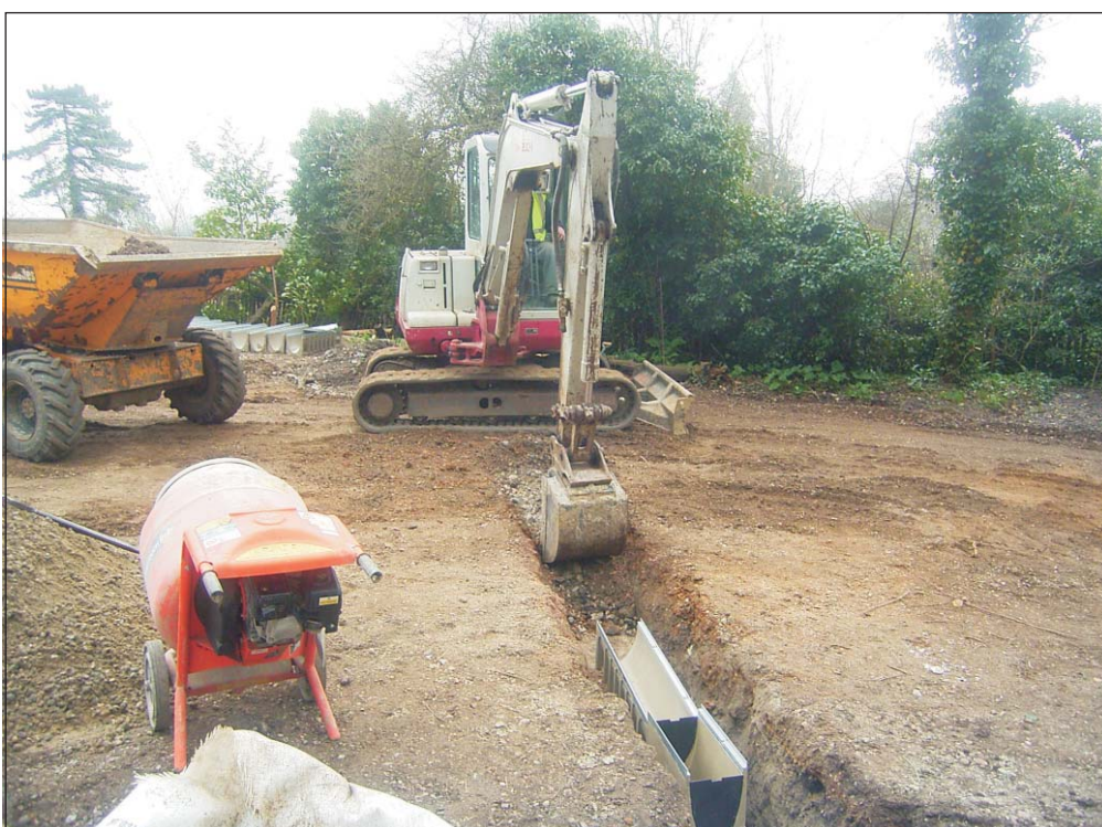
Plate 2: Machine excavation of the drainage trench, view from north-east
