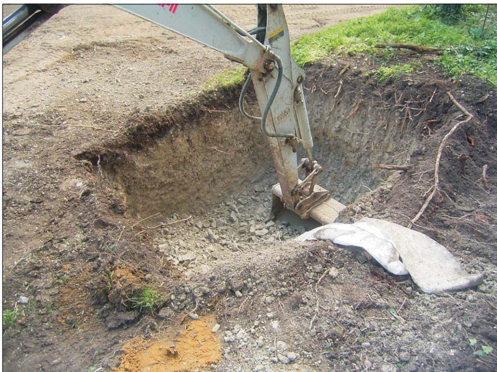
Plate 1: Machine excavation of the soakaway trench, view from north-east
