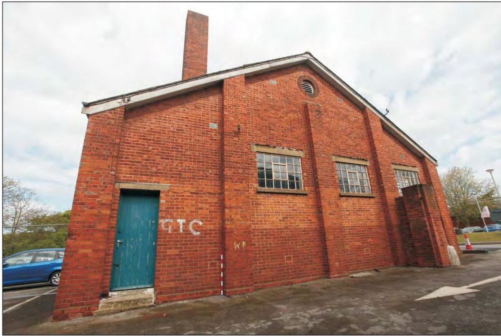
Plate 35: Building WA 0 211 viewed from the south-east
