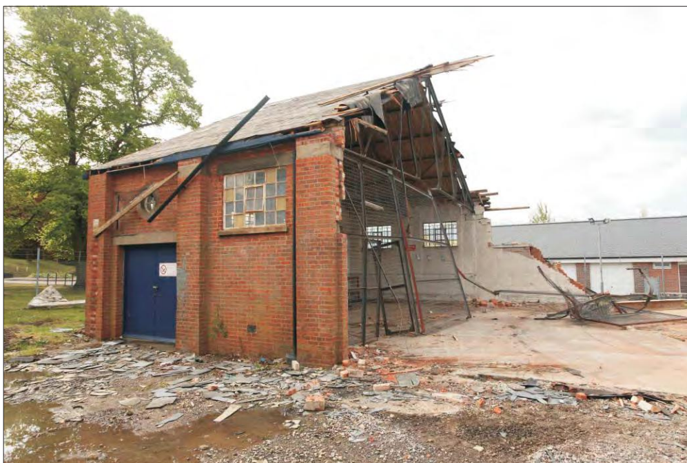
Plate 38: Building WAA 218 viewed from the north-east during demolition
