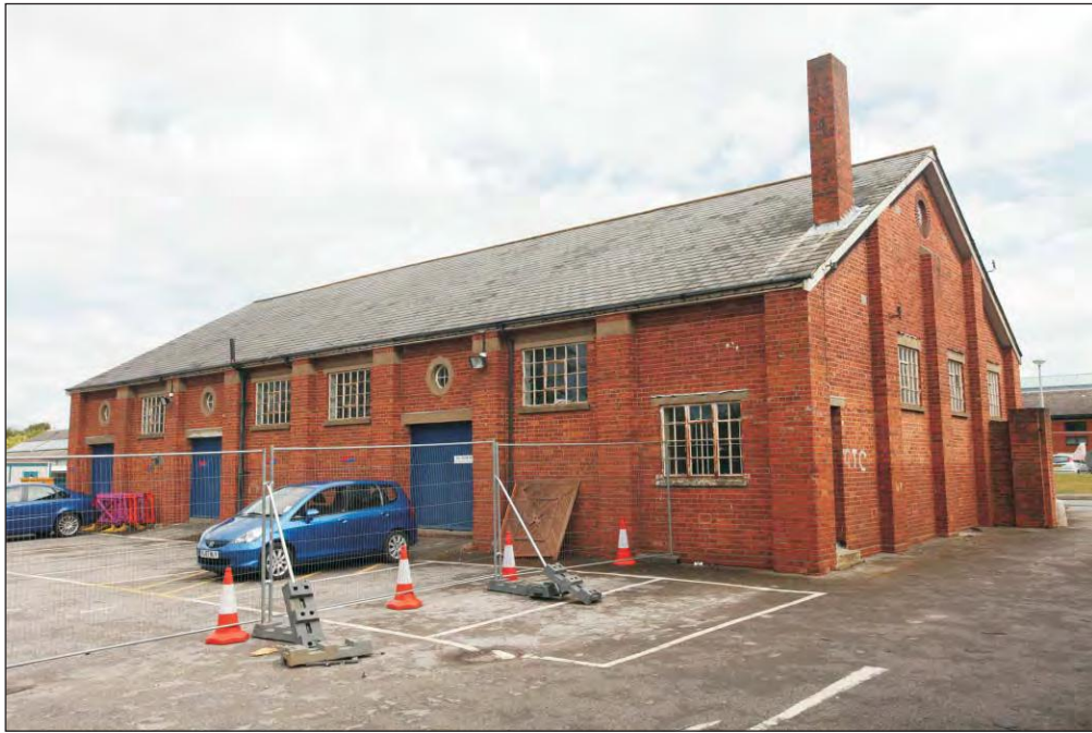
Plate 33: Building WA 0 211 viewed from the south
