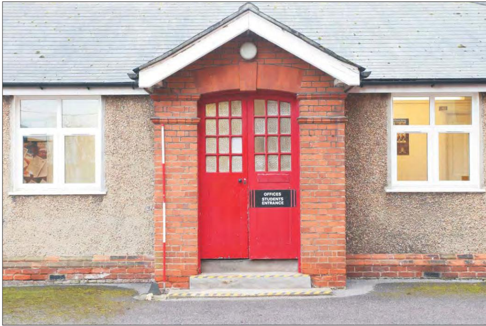
Plate 21: Building PT0 127 Entrance porch viewed from the north-west
