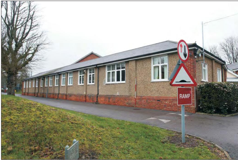
Plate 19: Building PT0 127 viewed from the east
