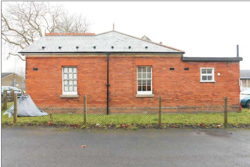
Plate 3: Building PVA 071 viewed from the south-east
