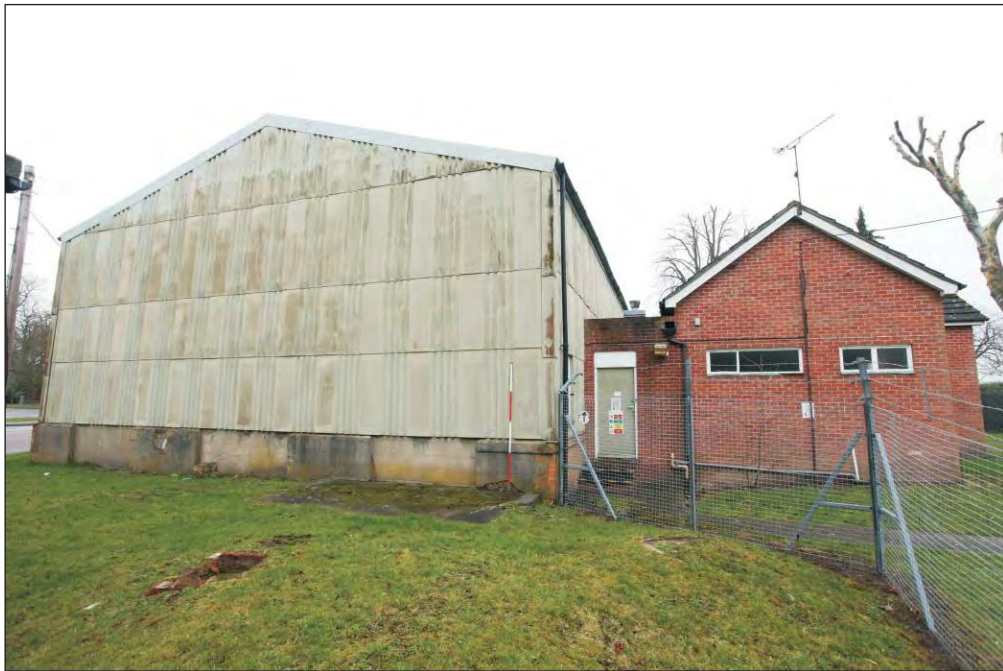
Plate 26: Building PT0 123 viewed from the south-east
