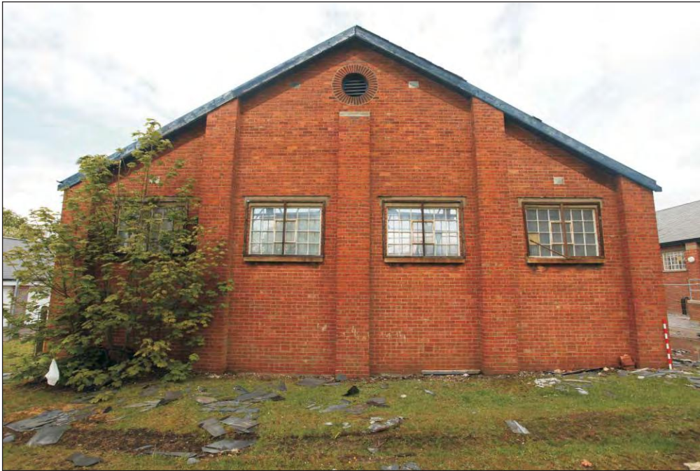
Plate 39: Building WAA 218 viewed from the south-east during demolition
