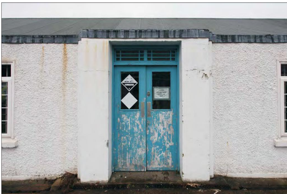
Plate 14: Building PVA 078 entrance viewed from the south-west
