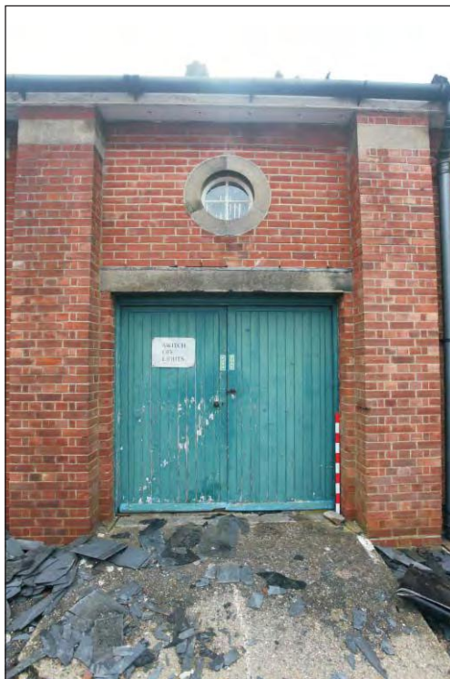
Plate 28: Building WA 0 217 - one of three identical doors on the north-west elevation
