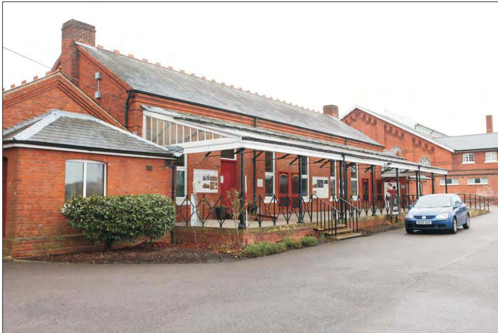
Plate 17: Building PT0 133 Verandah viewed from the east
