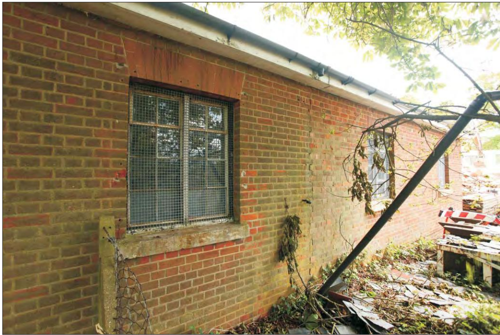
Plate 45: Building WA O 215 - Store viewed from the west
