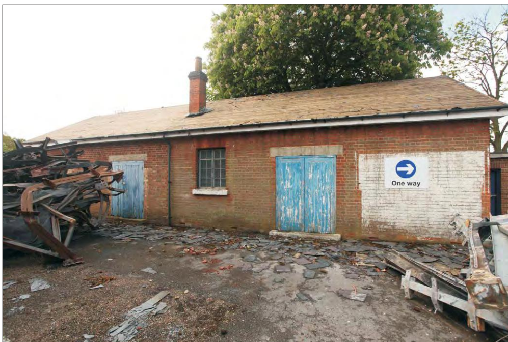
Plate 44: Building WA O 215 - Store viewed from the north
