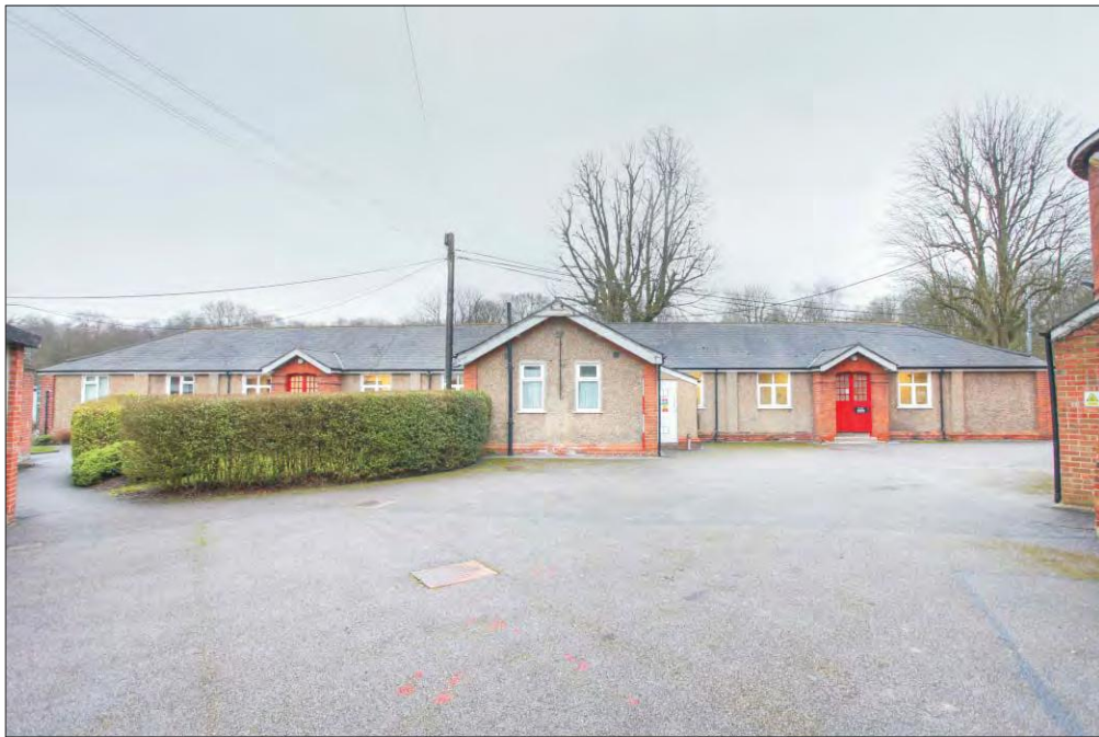
Plate 20: Building PT0 127 viewed from the north-west
