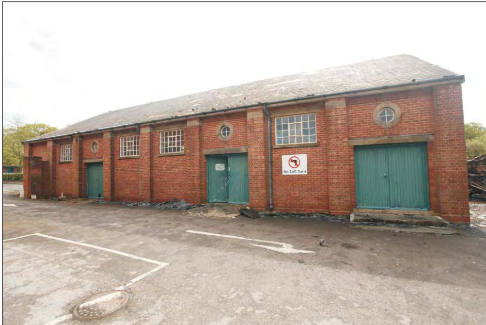
Plate 27: Building WA 0 217 viewed from the west
