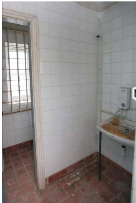
Plate 16: Building PVA 078 interior - toilet block viewed from the west
