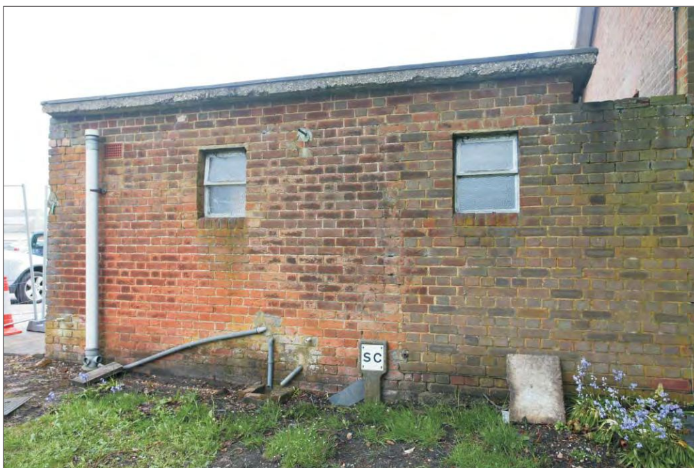
Plate 42: Building WA O 215 - Toilet Block viewed from the south-west
