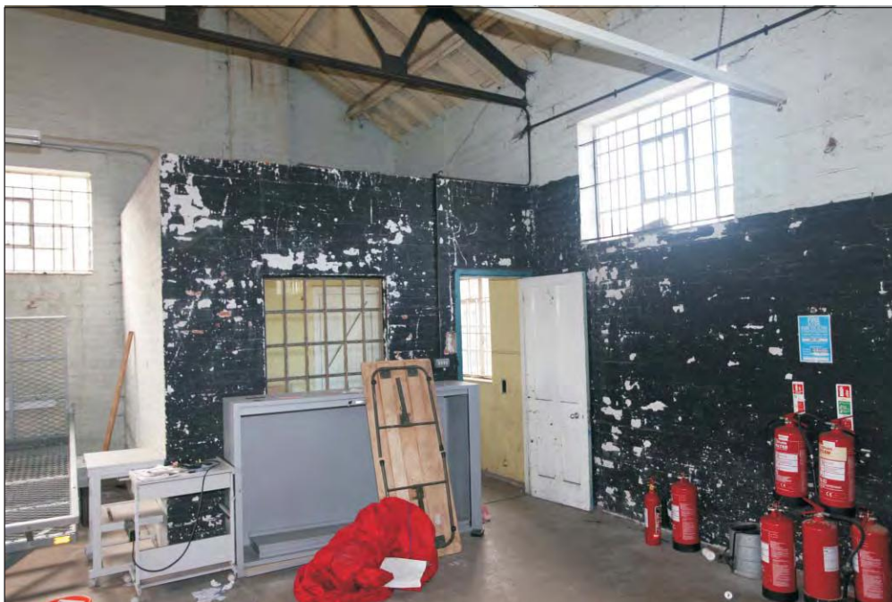
Plate 37: Building WA 0 211 interior – office viewed from the north
