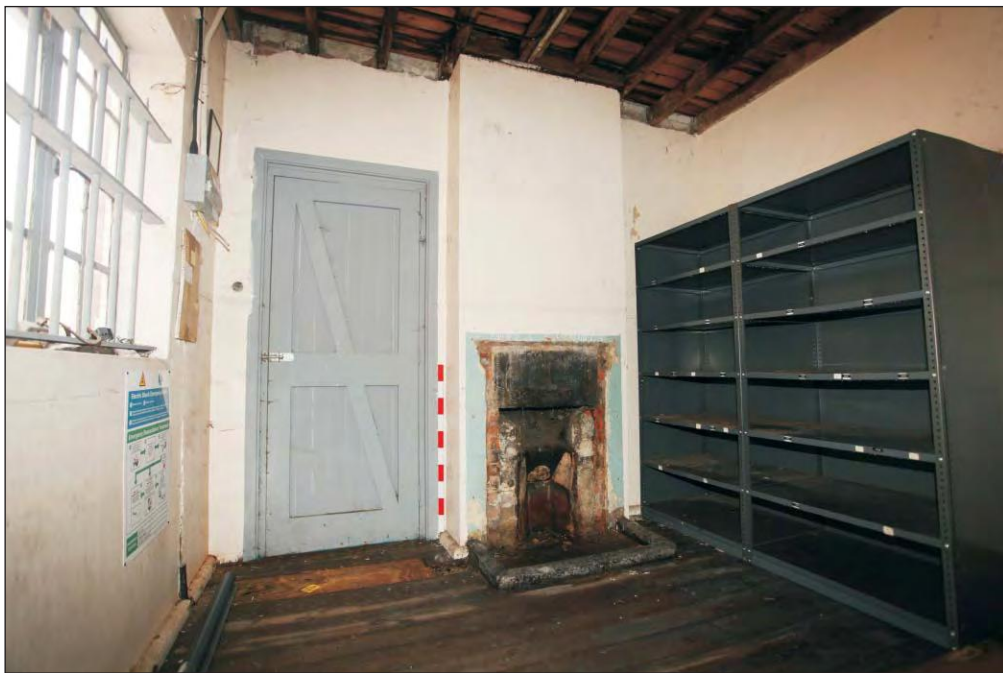
Plate 32: Building WA 0 211 viewed from the south
