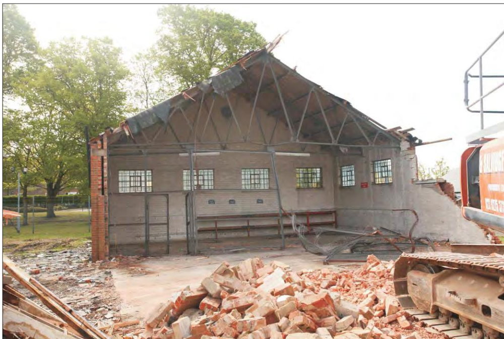
Plate 40: Building WAA 218 interior - viewed from the north-west during demolition
