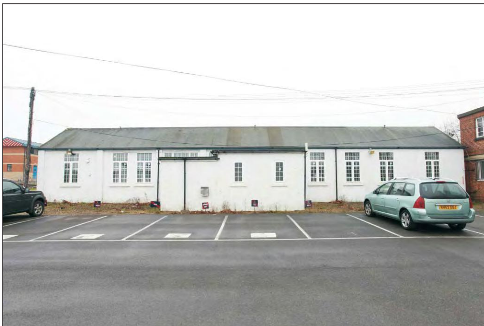
Plate 13: Building PVA 078 viewed from the north-east
