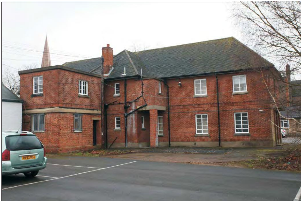
Plate 8: Building PVA 073 viewed from the north-east
