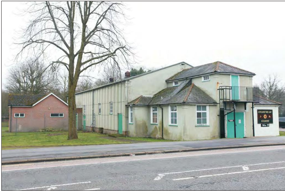
Plate 25: Building PT0 123 viewed from the north-west
