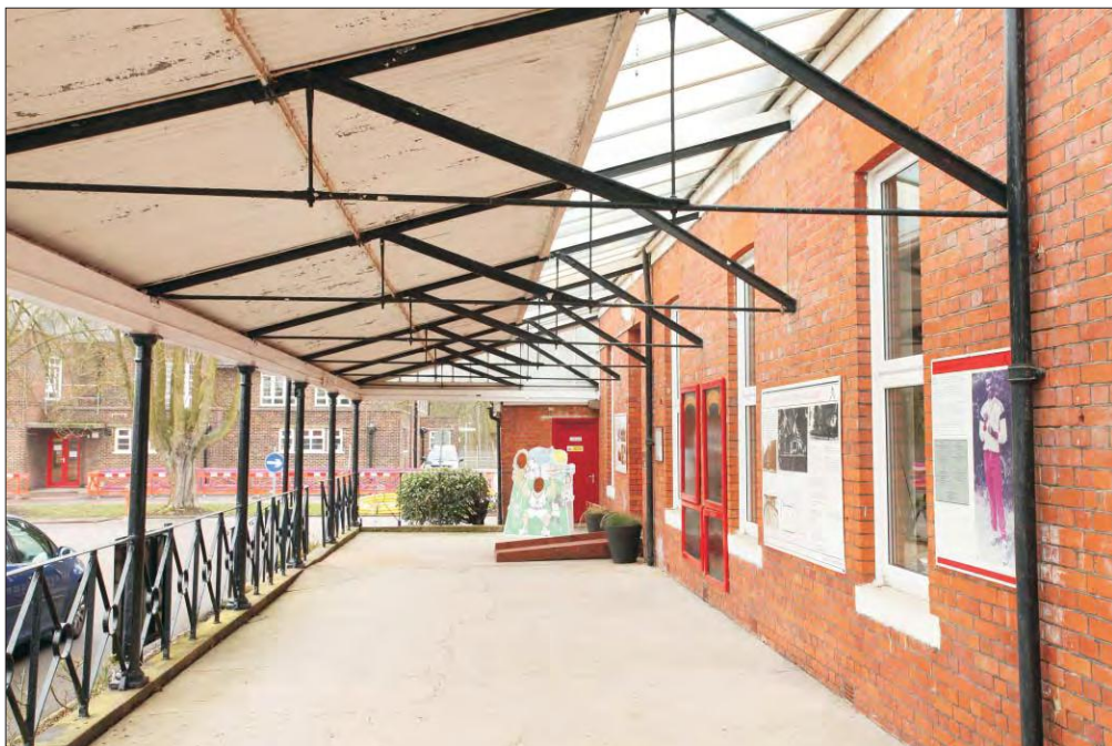
Plate 18: Building PT0 133 Verandah viewed from the north-west
