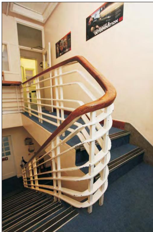
Plate 10: Building PVA 073 interior - staircase viewed from the north-west
