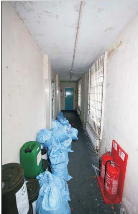
Plate 15: Building PVA 078 interior - long corridor viewed from the north-west
