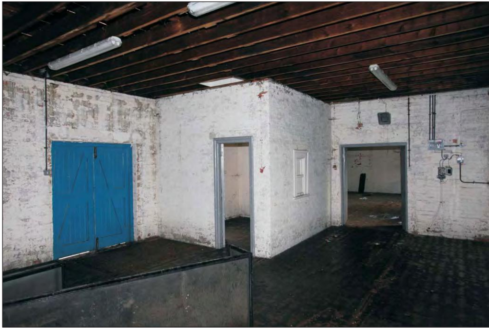
Plate 47: Building WA O 215 - Store - interior viewed from the west
