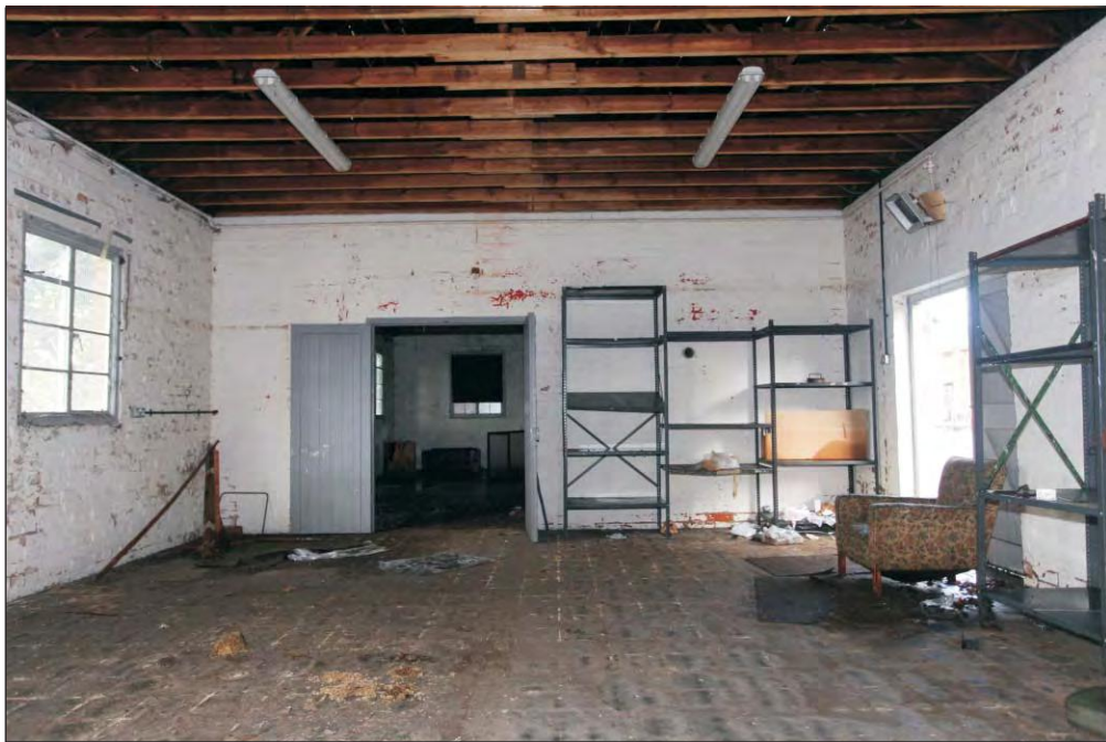
Plate 46: Building WA O 215 - Store – interior viewed from the south-east
