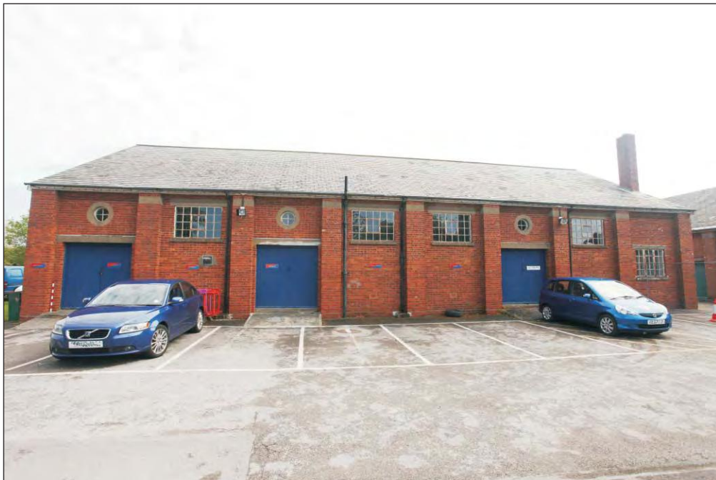
Plate 34: Building WA 0 211 viewed from the south-west
