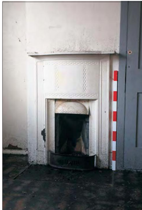
Plate 48: Building WA O 215 - Store – interior fireplace viewed from the south-west
