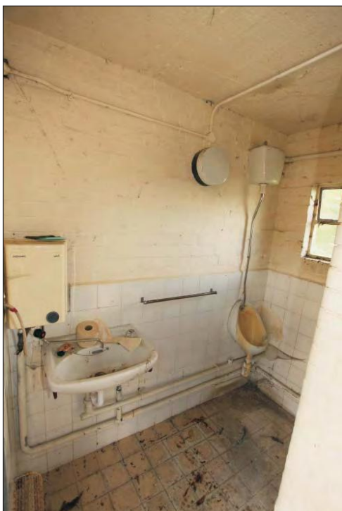
Plate 43: Building WA O 215 - Toilet Block – interior viewed from the north
