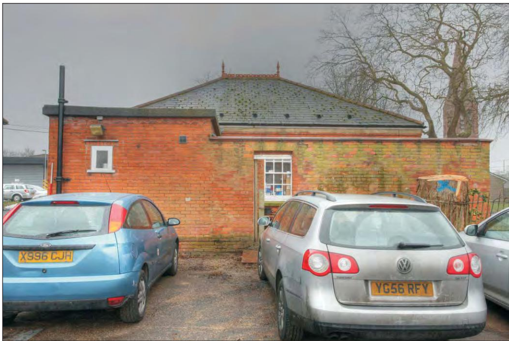
Plate 2: Building PVA 071 viewed from the north-east
