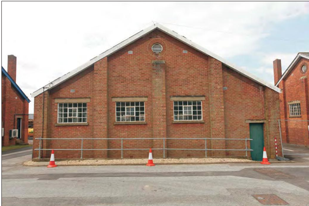
Plate 29: Building WA 0 217 viewed from the north-east
