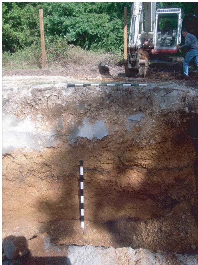
Plate 2: Garage foundation trench section
