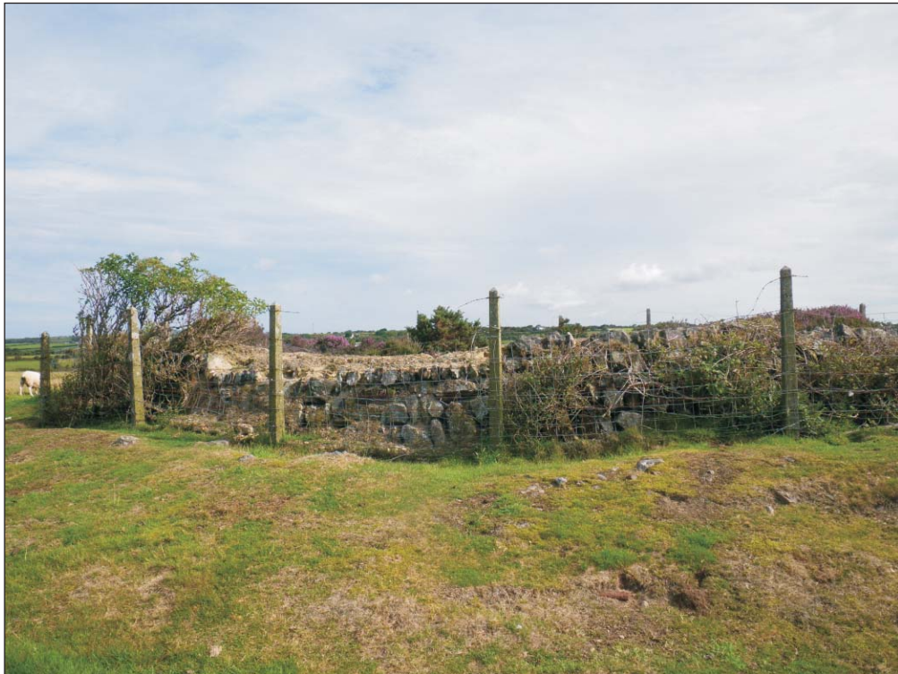
Plate 1: Wall collar at the summit of Shaft 12, view from west
