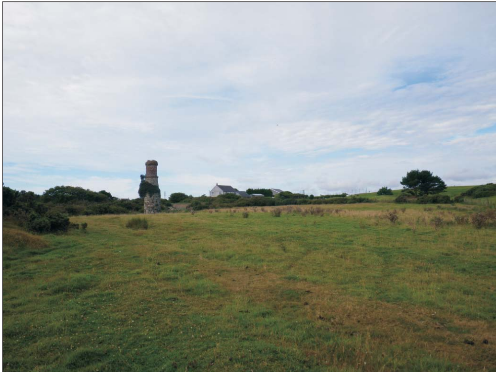
Plate 2: Chimney Stack Listed Building in its present setting, view from north-east
