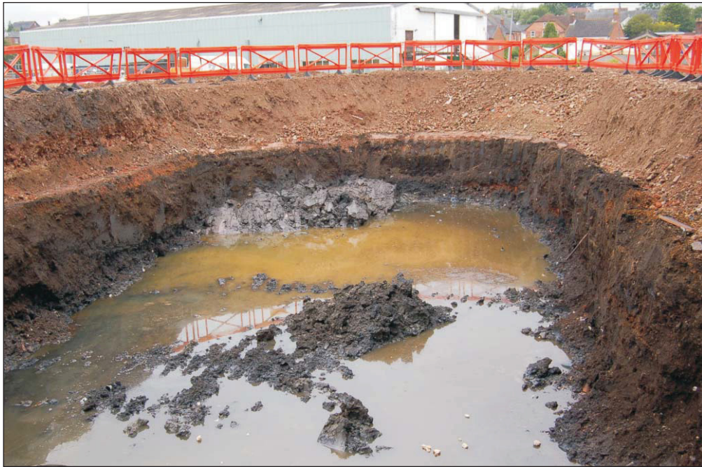
Plate 1: West facing photograph of Trench 1
