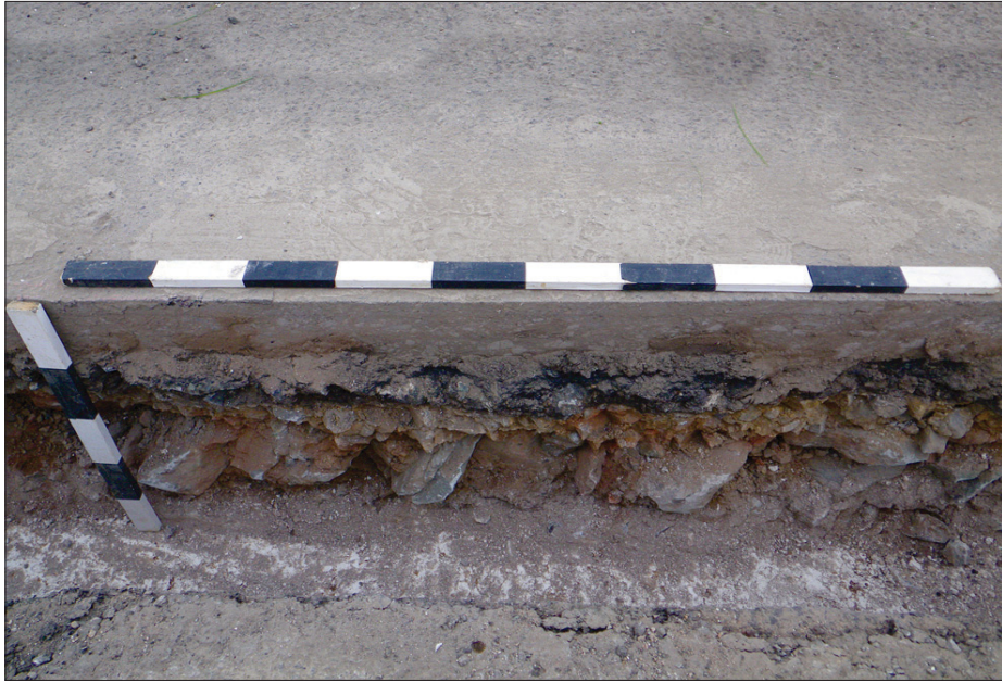
Plate 1: Section through road surface showing road construction down to chalk natural
