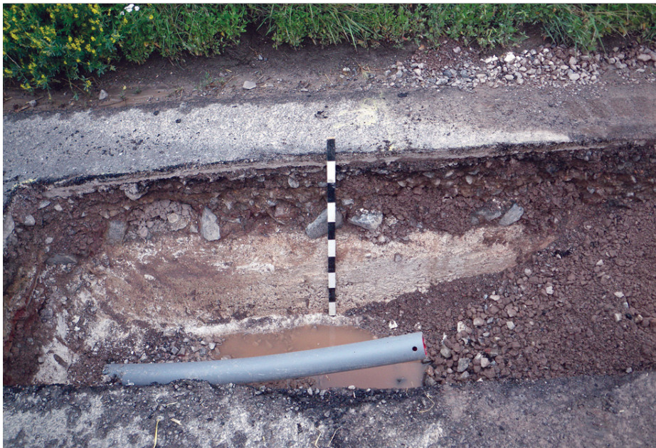
Plate 2: Fully excavated launch pit at east end of trench
