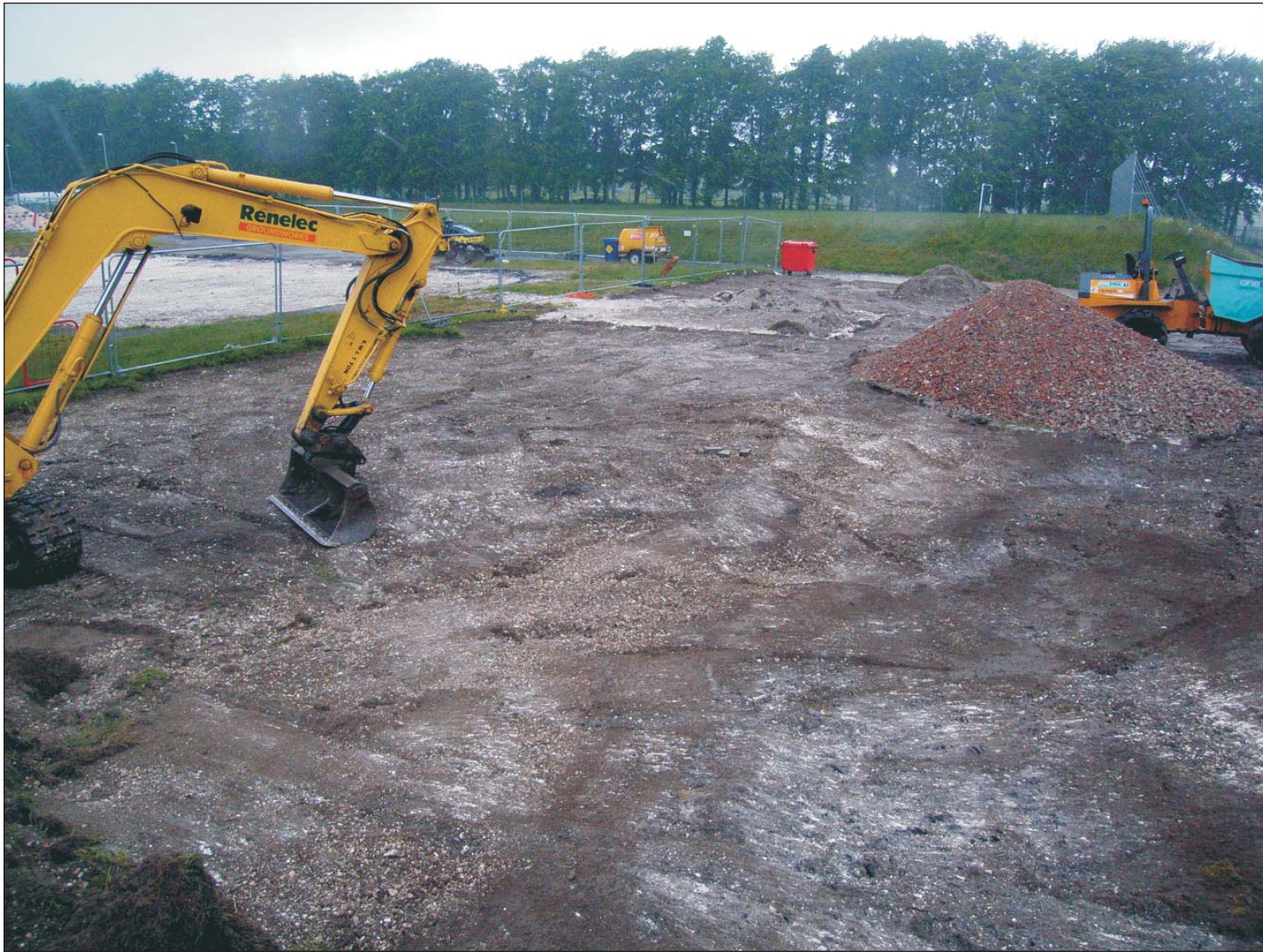
Plate 1: Area stripped to construction level. View from the south
