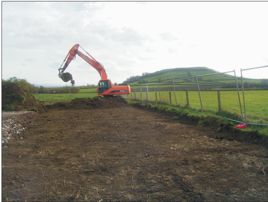
Plate 1: General working view of Area 1, view from west
