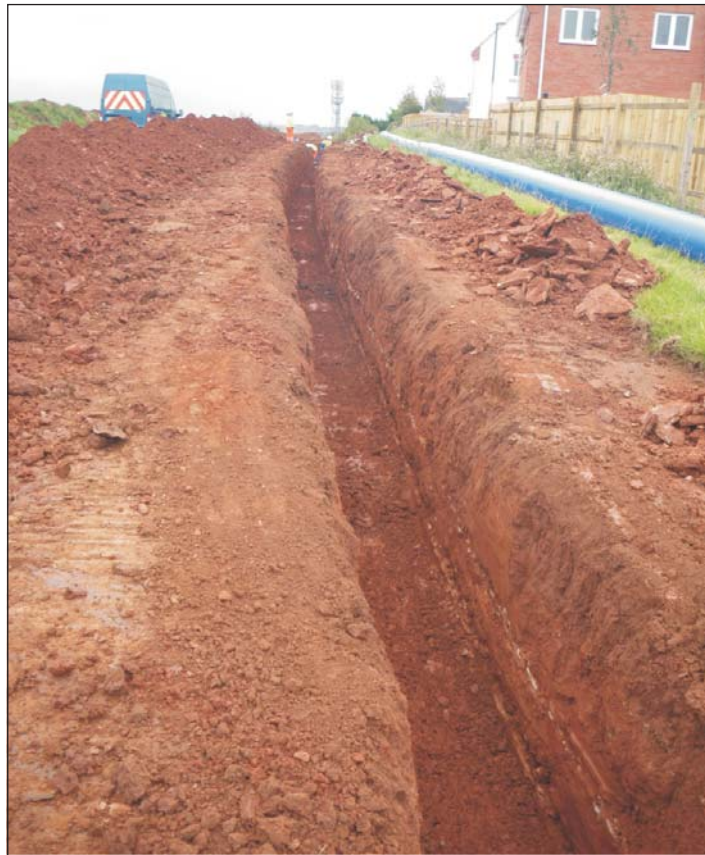
Plate 3: Pipe trench in Area 1
