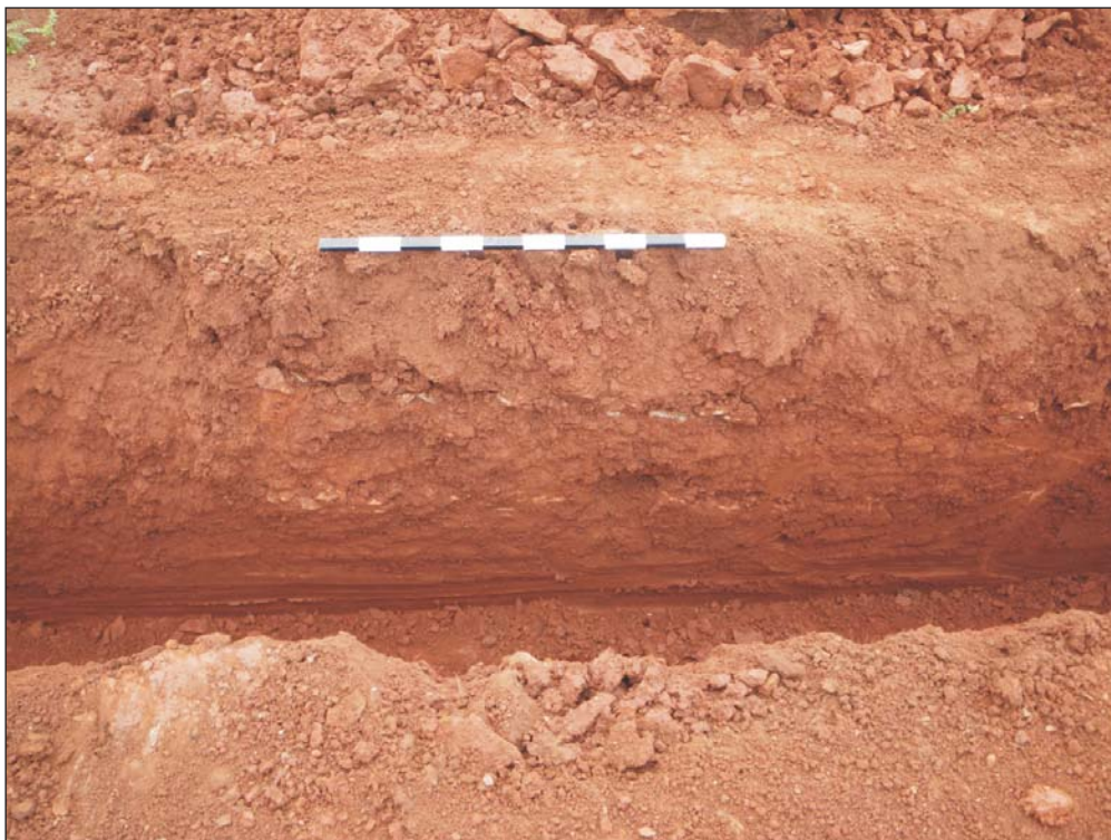
Plate 4: East facing representative section of pipe trench in Area 2
