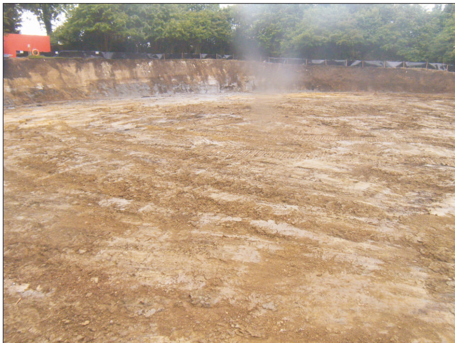
Plate 2: Area 3 following machine excavation
