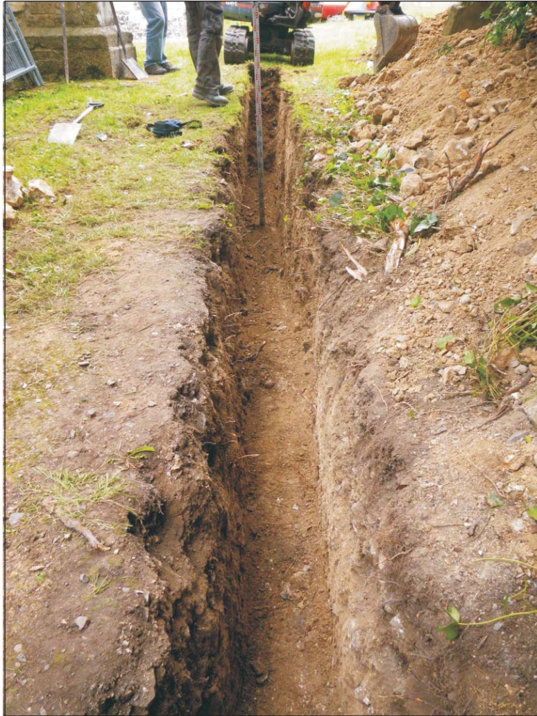
Plate 1: South-east facing trench following excavation
