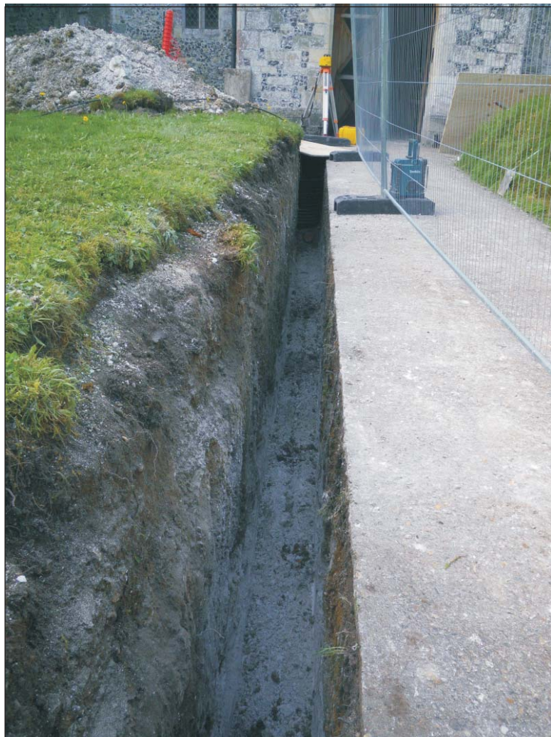
Plate 3: North facing photograph of pipe trench
