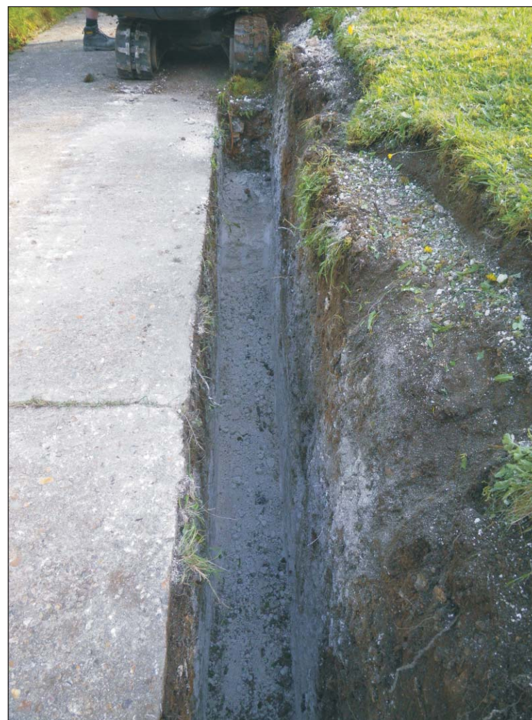
Plate 4: South facing trench following excavation
