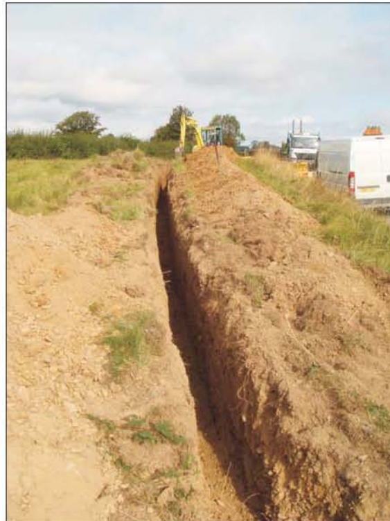
Plate 2: Trench 8 , view from south
