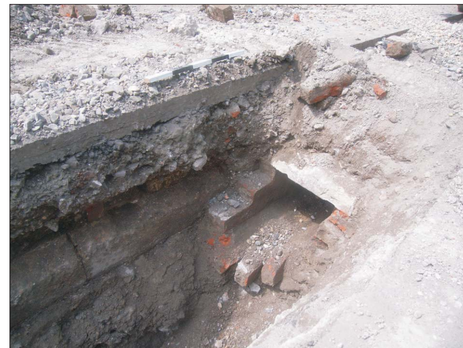
Plate 2: Relationship between kerb stones and later brick built utility
