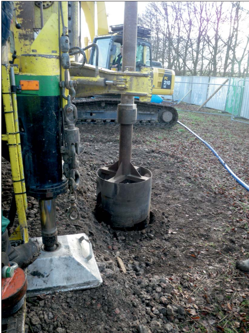
Plate 3: Borehole 1 within watching brief area
