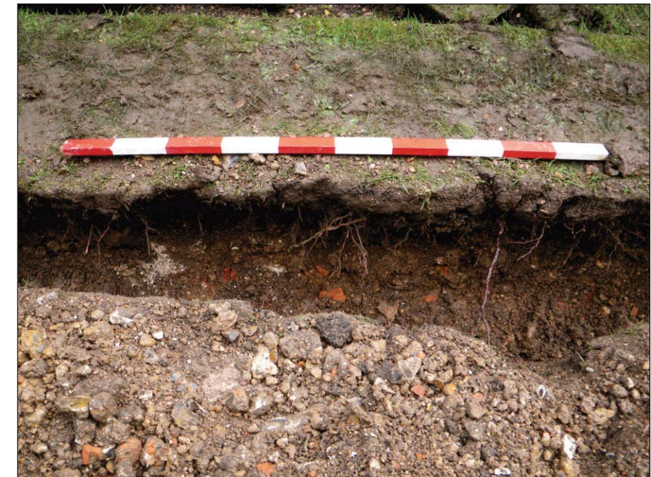
Plate 6: West facing section of BT Data cable trench
