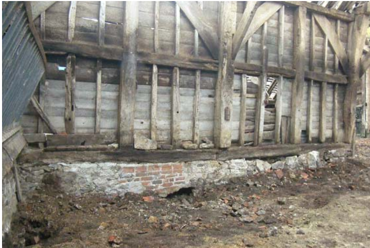
Plate 1: North wall of Main Barn, deposit 1702
