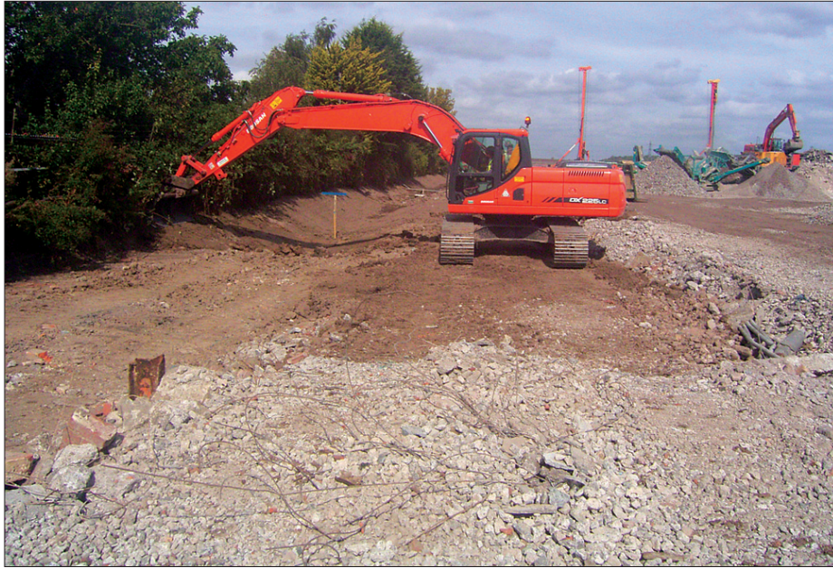
Plate 5: Cutting the culvert
