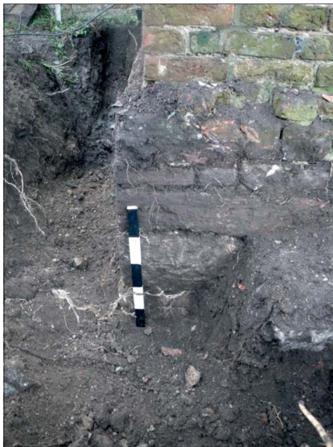
Plate 4: North-west facing elevation of stone foundations at north-western corner of Cottage 609 in the French Drain
