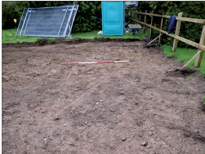
Plate 1: Footprint of building following topsoil strip, looking south
