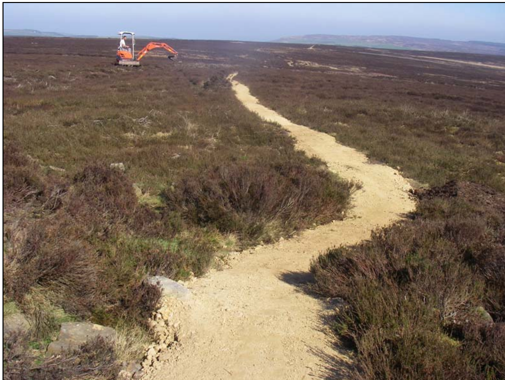
Plate 3: New path, view from southwest
