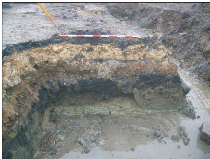
Plate 2: North facing section of strip footing
