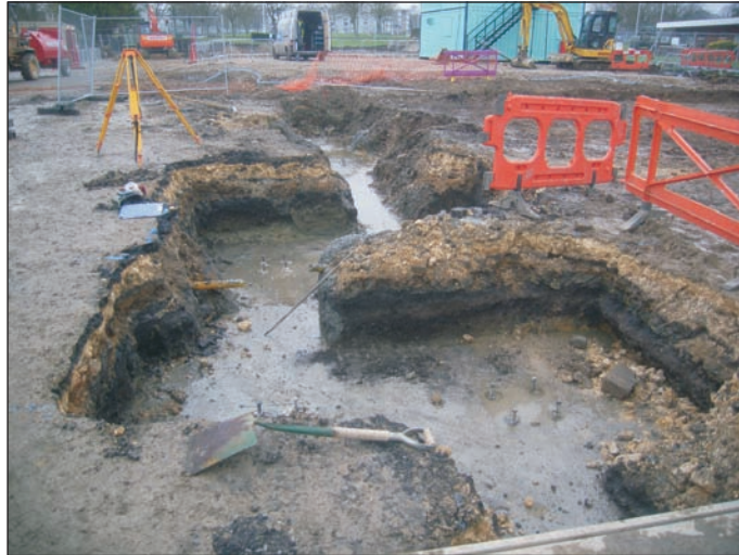
Plate 1: View of strip footings from the north
