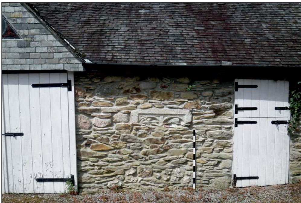
Plate 1: Location of the tracery window fragment
