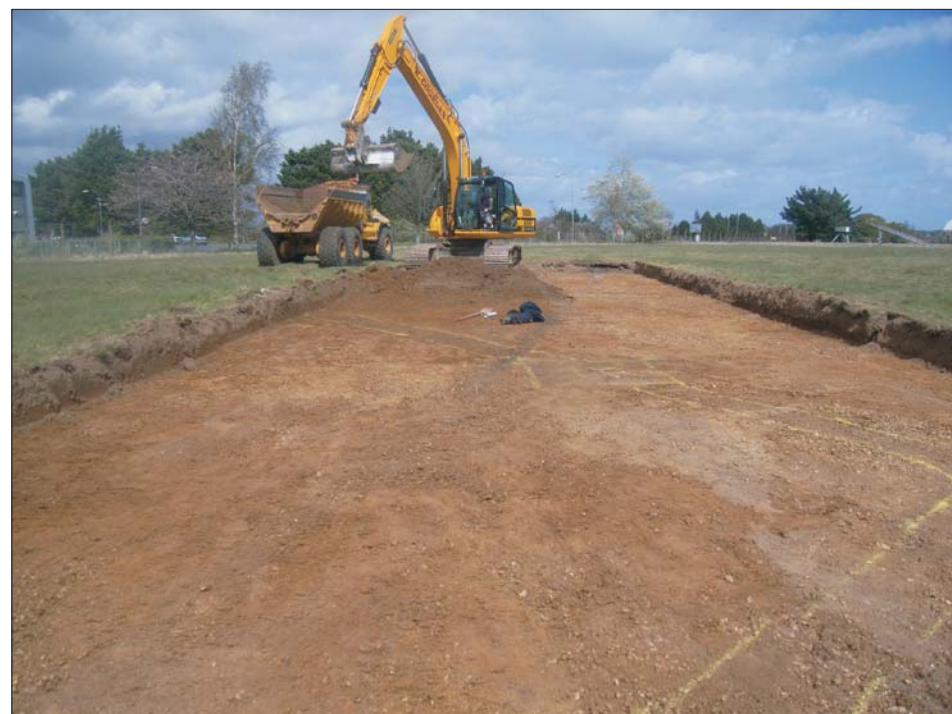
Plate 1: General view of machine excavation of Area 16
