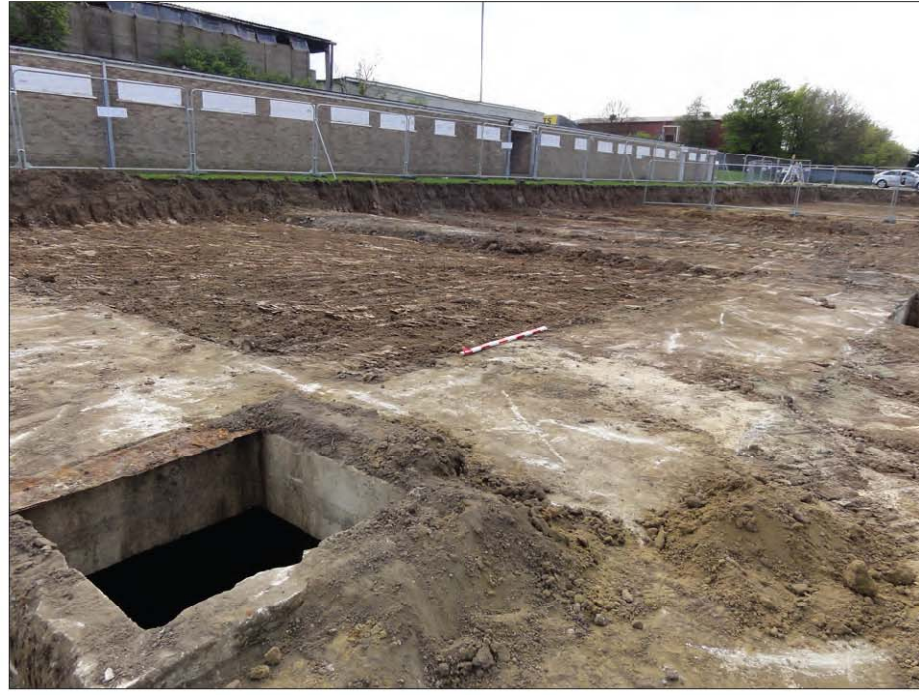
Plate 2: View across exposed roof of air raid shelter. Looking south-west.
