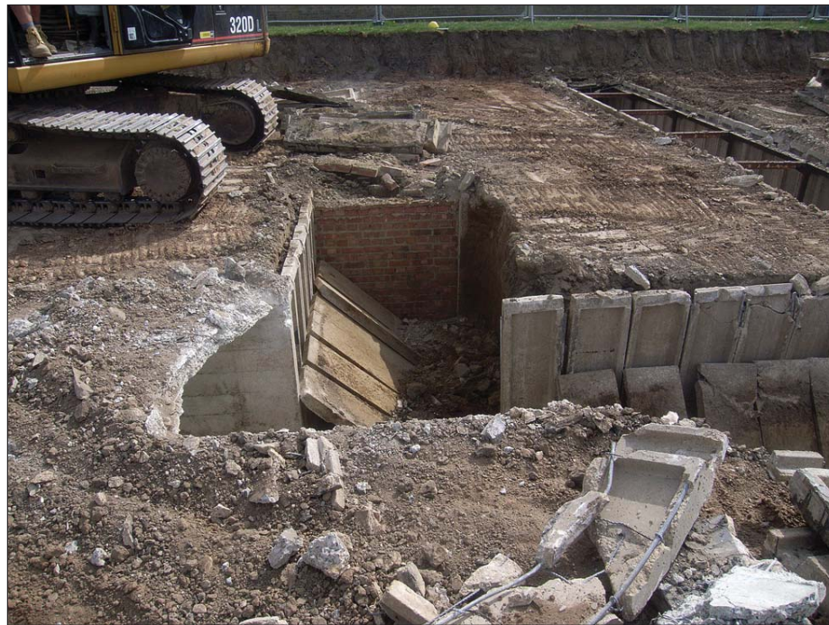
Plate 17: Bricked up entrance exposed during demolition works. Looking south
