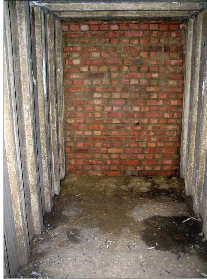
Plate 5: Bricked up former entrance, Tr 1a. Looking south.
