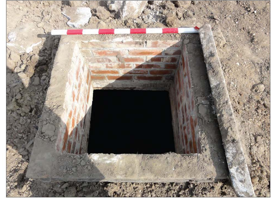
Plate 3: Surface view of manhole at north-west corner of shelter (Phase 1).
