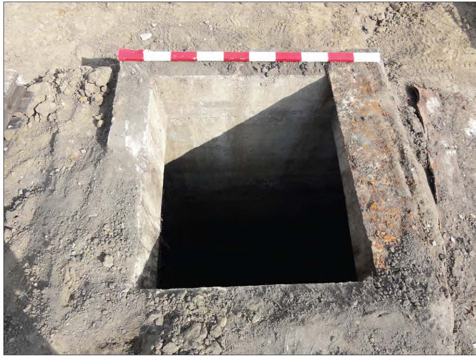
Plate 4: Surface view of manhole at north-east corner of shelter (Phase 2).
