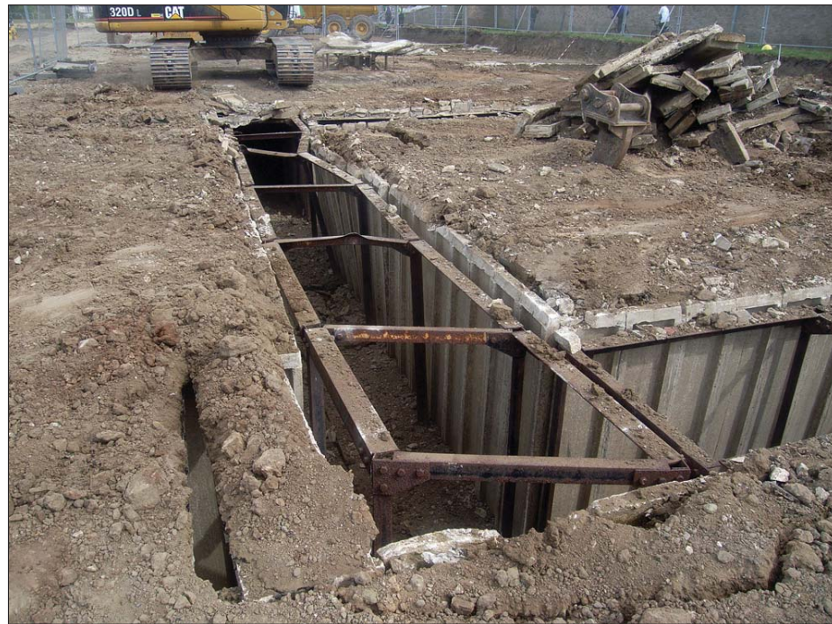
Plate 16: Junction of Tr 1b and Tr 1d during demolition. Looking south-east.
