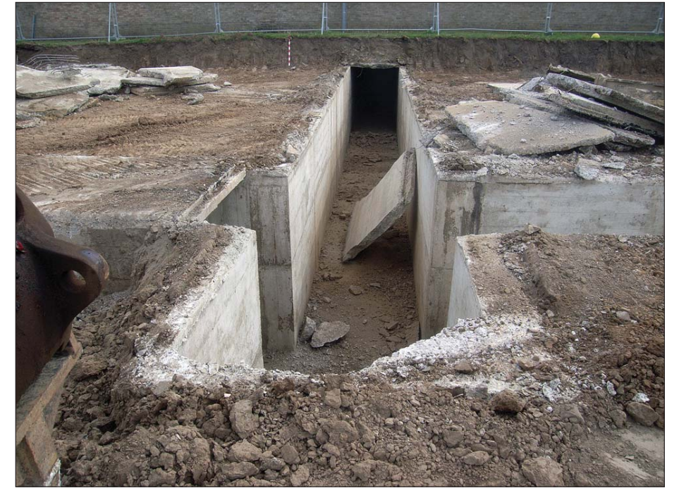
Plate 15: Tr 2b during demolition. Looking south.
