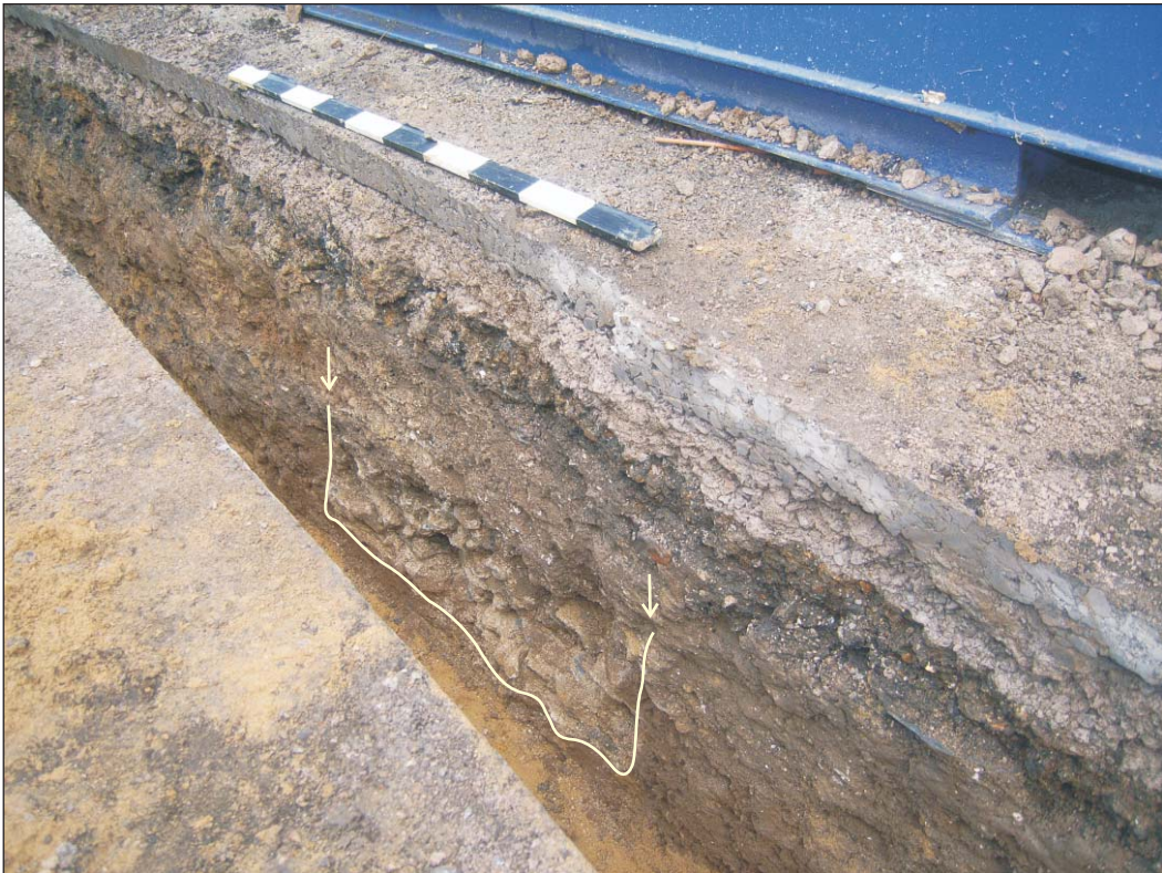
Plate 37: Trench 19 - Wall footing 1910
