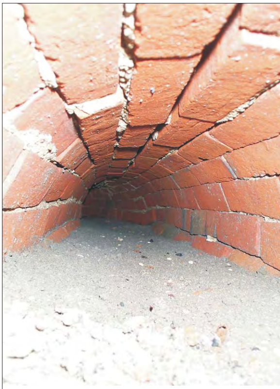
Plate 3: Trench 2 - Interior of drain 215 , looking west
