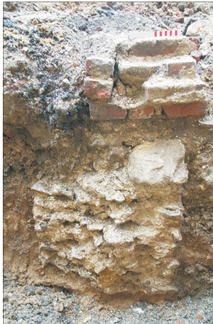
Plate 15: Underpinning Trench - Medieval wall foundation 306 seen in section
