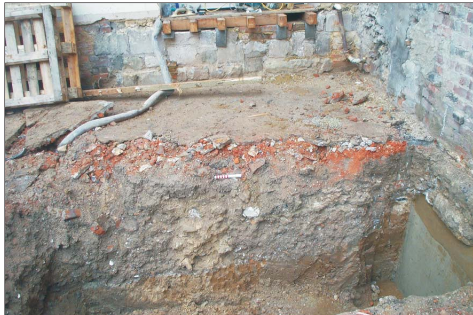
Plate 14: Underpinning Trench - Medieval wall foundation 308 seen in section
