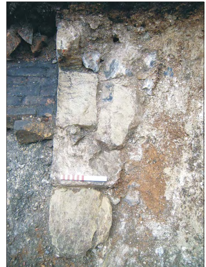
Plate 28: Trench 15 - Wall footing 1580 viewed from the south
