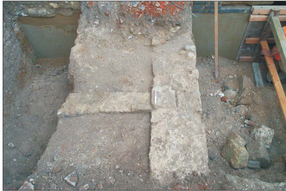
Plate 12: Underpinning Trench - Medieval wall foundations 304/305/308 seen in plan
