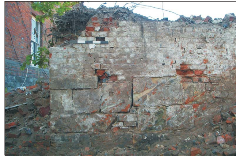
Plate 19: Remains of extant wall after Victorian cellar demolition
