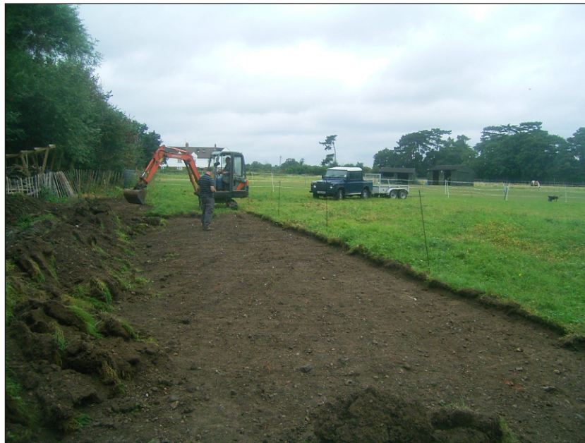
Plate 1: Excavation of topsoil looking north
