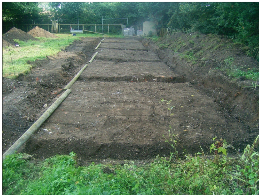
Plate 4: Excavated area looking south
