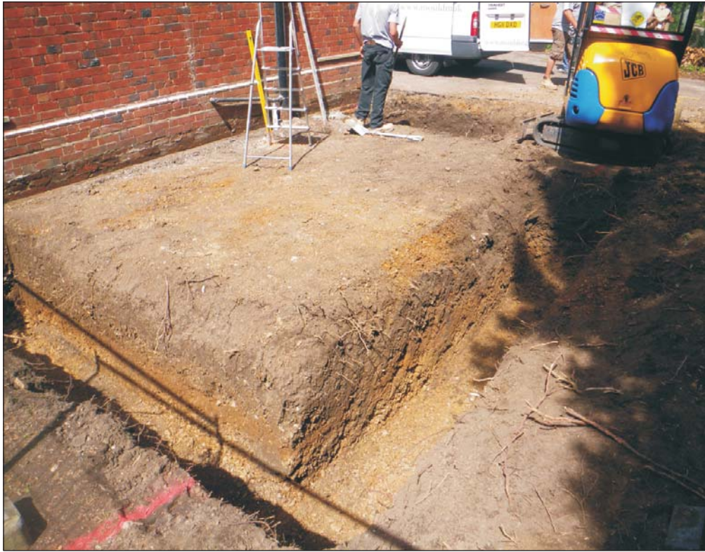
Plate 2. General view of works
