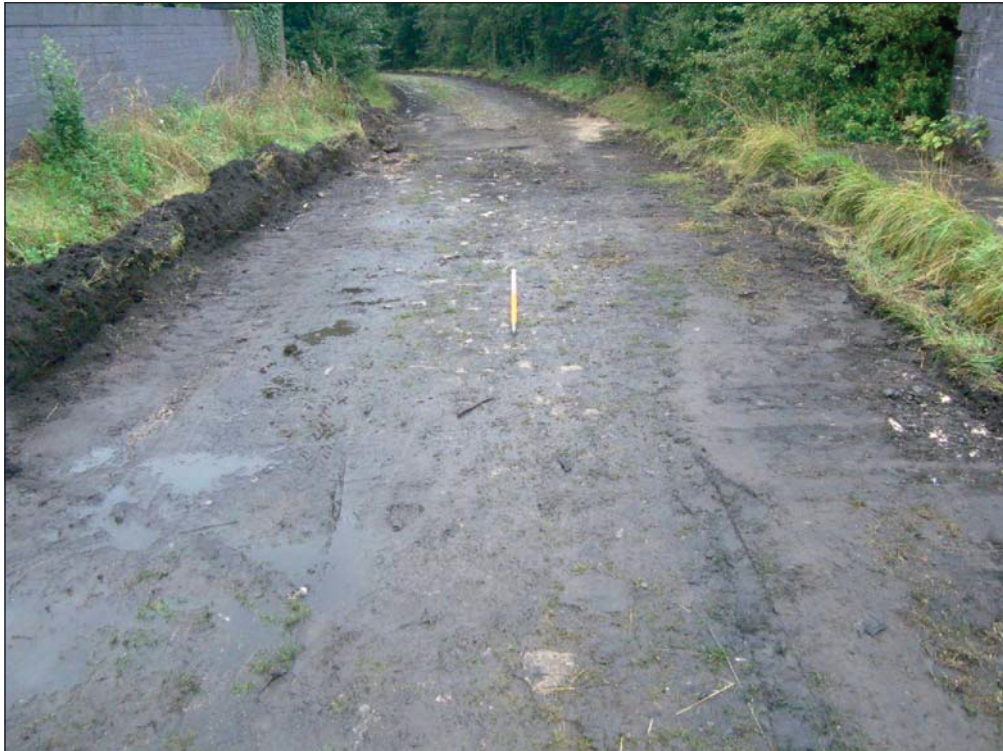
Plate 3: Average depth of strip on central section of watching brief. Facing north.
