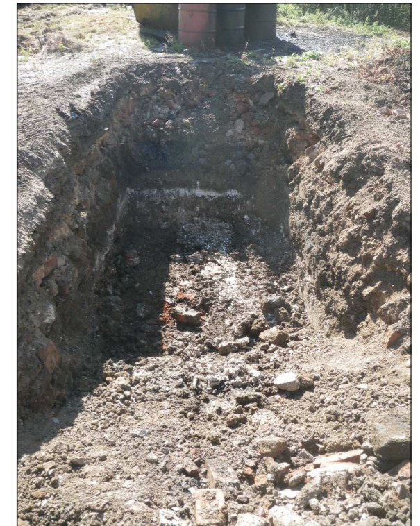
Plate 4: Trench 4 from the south
