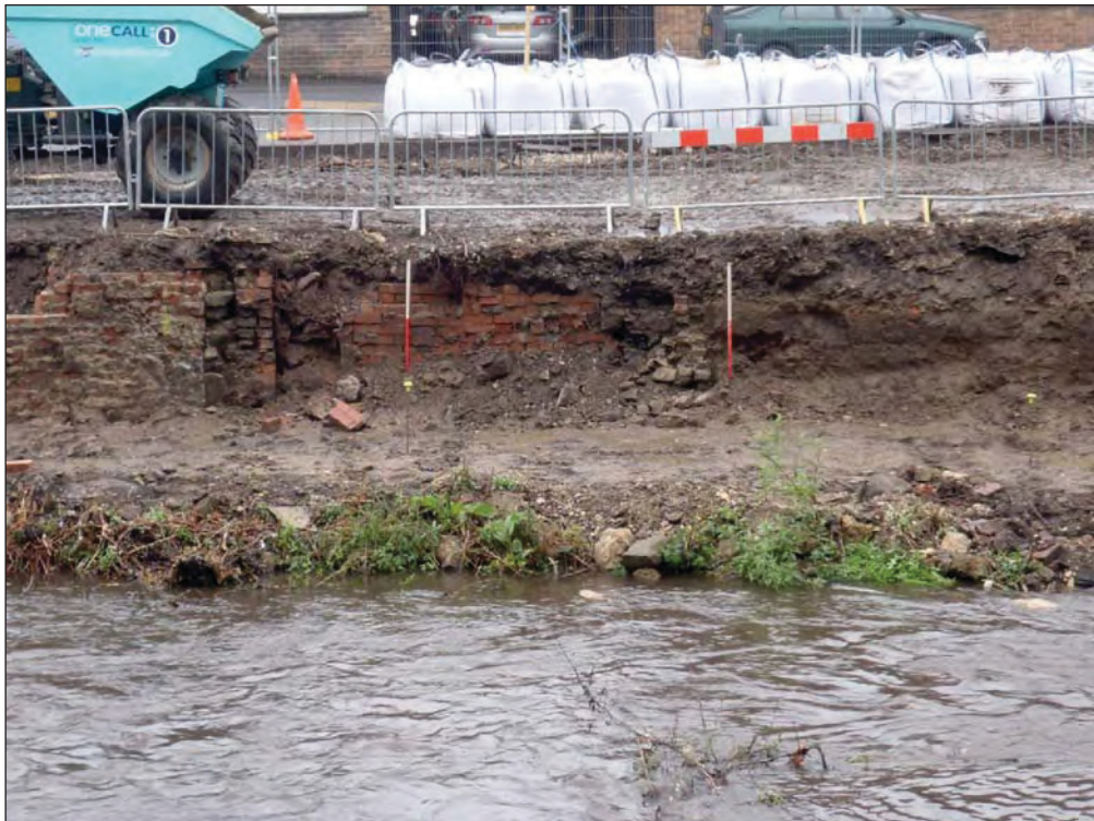
Plate 12: aM 603 - 608 & 617, northern riverside area, looking northeast.
