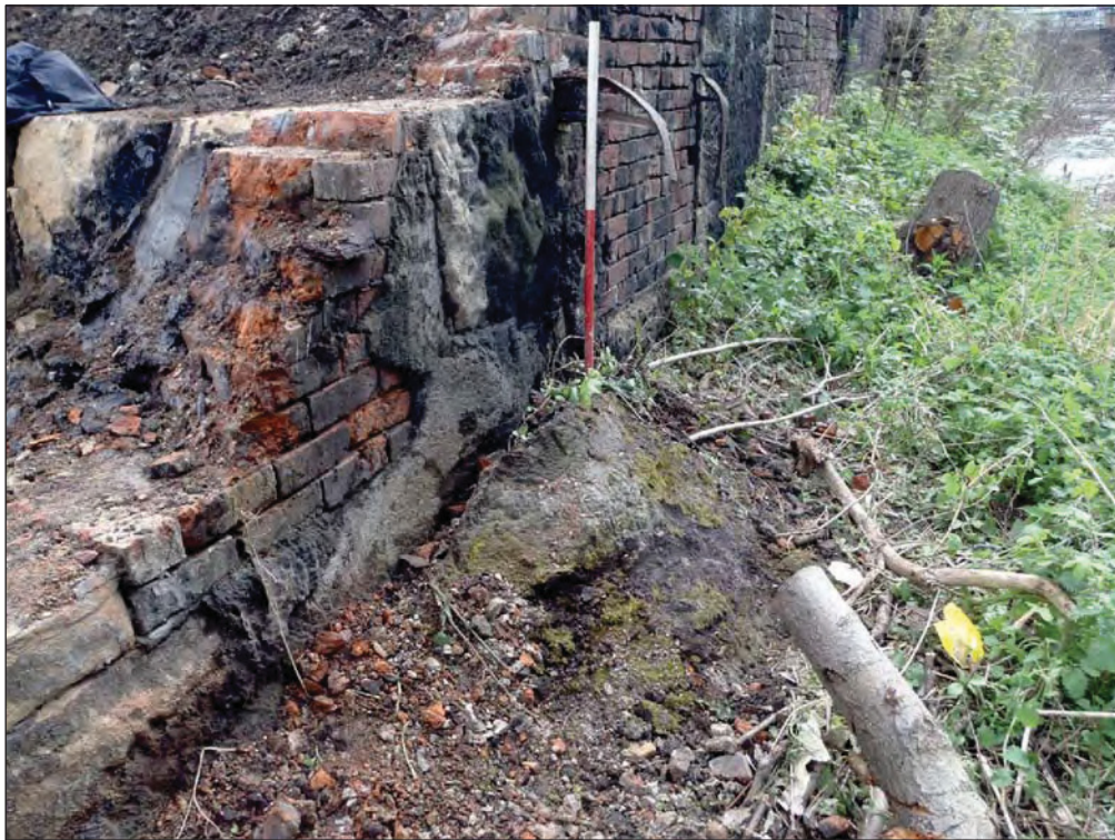
Plate 7a. Like material 663 near machine base 659, southern area, looking southeast.
