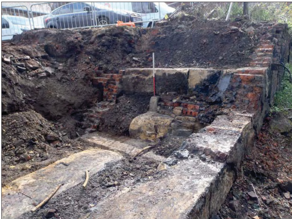
Plate 6: Machine 659, south part of Site, looking southeast.
