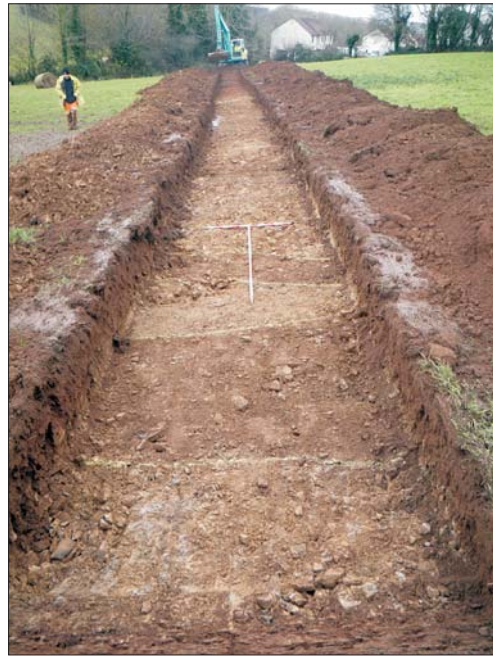
Plate 2: Trench 3 viewed from the north-east
