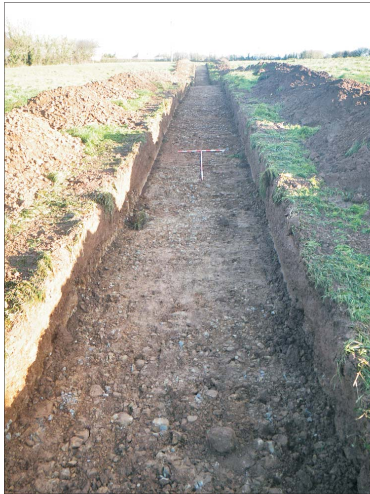
Plate 13: Trench 14 viewed from the south-west
