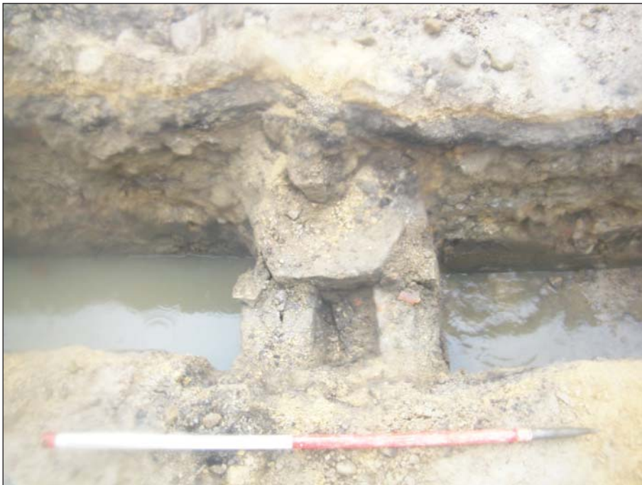
Plate 14: Detail of east-west aligned stone culvert 1013 in path south from Flora's Temple
