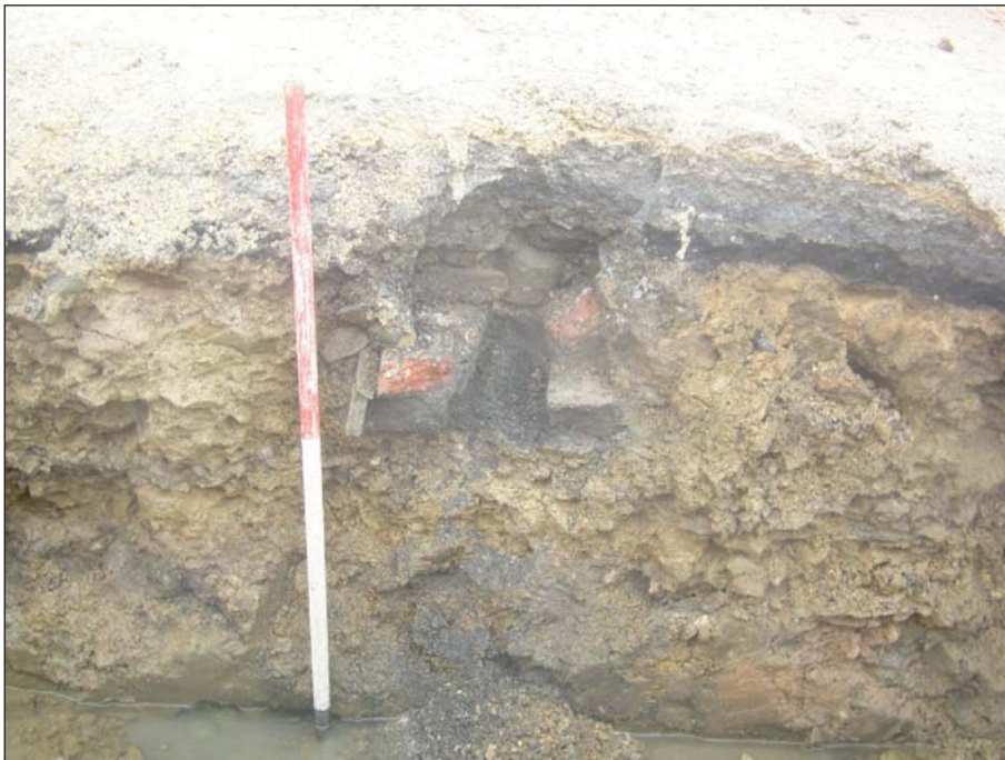
Plate 20: Example of brick lined culvert 1012 in path south from Flora's Temple
