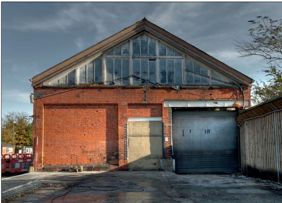
Plate 6: West facing elevation
