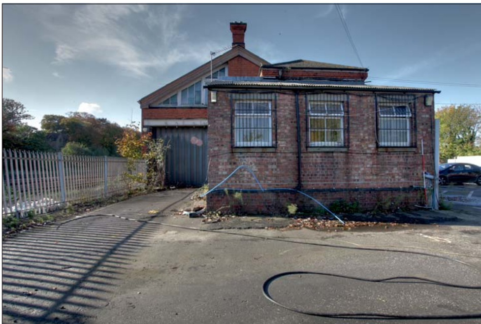
Plate 8: East facing elevation showing office extension
