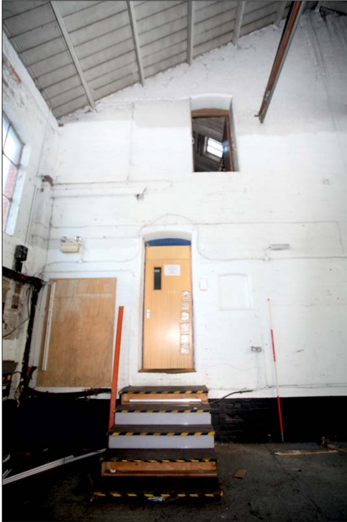
Plate 11: East wall of shed showing access into office and attic areas
