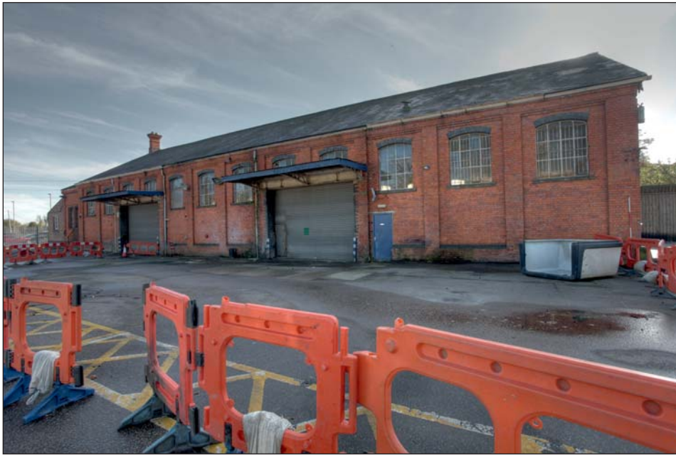
Plate 3: North facing elevation from north-west
