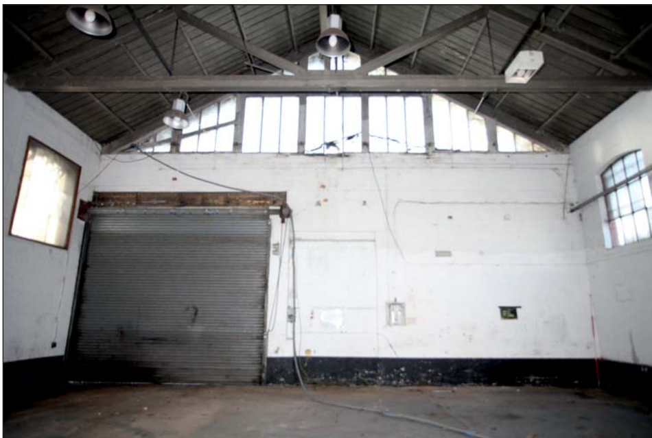
Plate 10: West wall of shed
