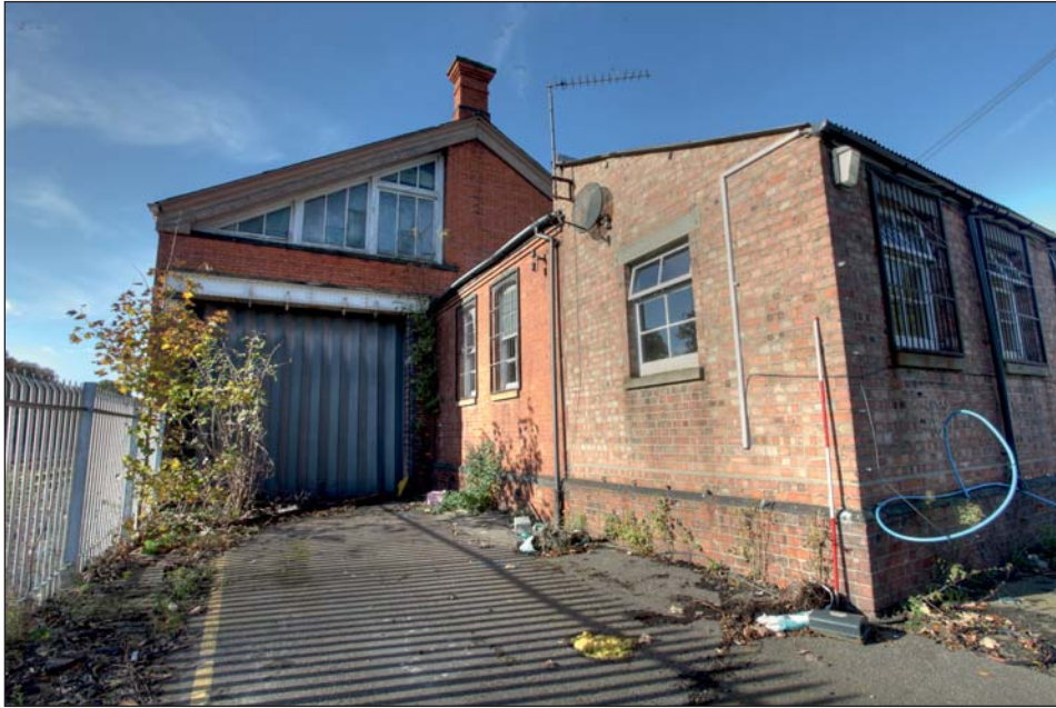
Plate 5: East facing elevation of shed from south-east, also shows south elevation of office
