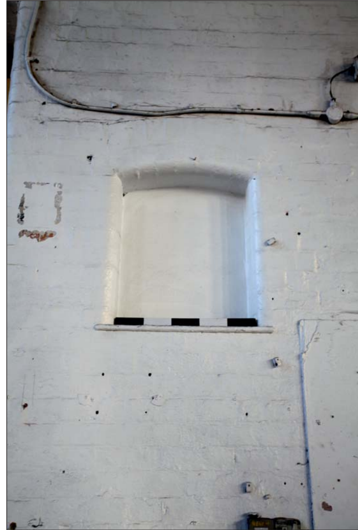
Plate 12: Detail of hatch in east wall of shed
