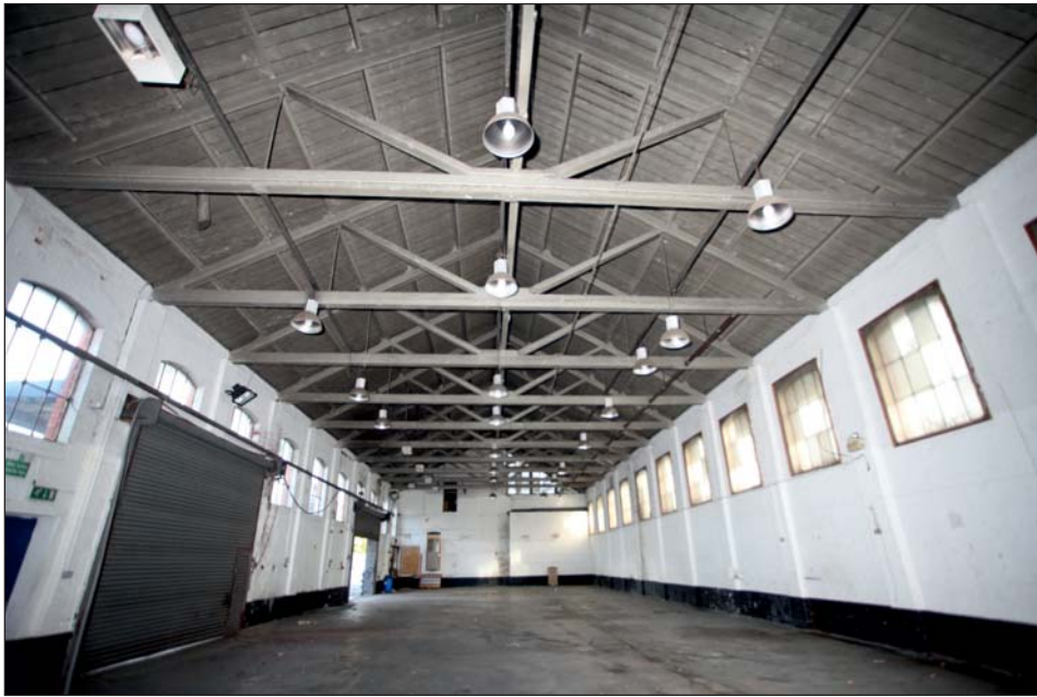
Plate 9: Interior of shed viewed from west
