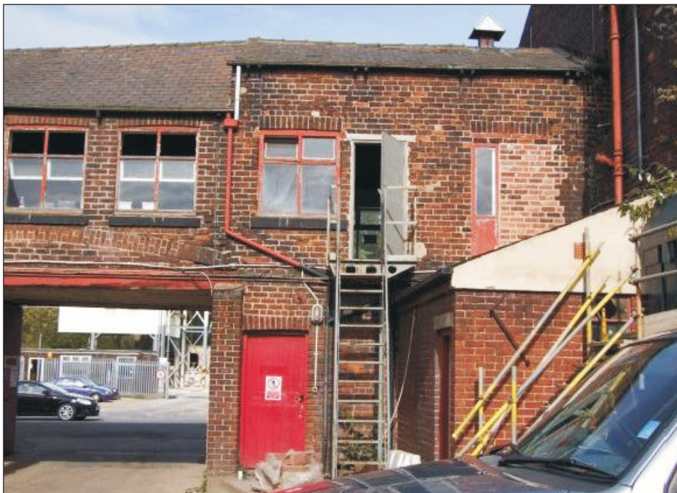
Plate 6: General view of southwest elevation of the Northeast Range (Film D.14)
