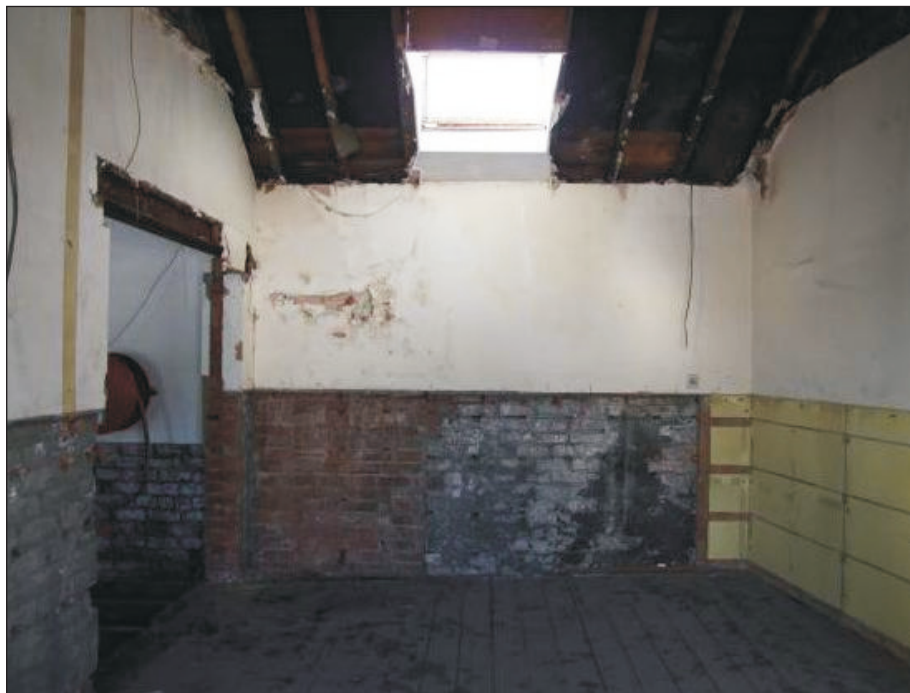
Plate 16: General view of F1, showing blocked opening & skylight (Film D.24)
