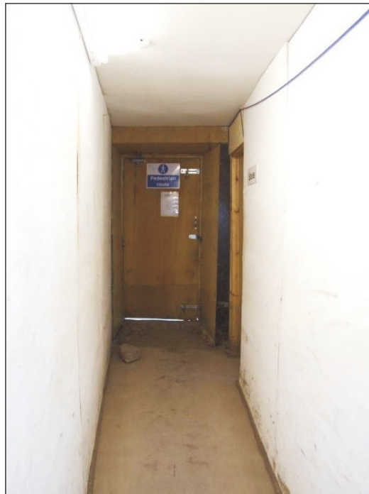
Plate 44: General view of modern corridor inserted into G16, with doorway leading to the former adjacent site (Film D.71)
