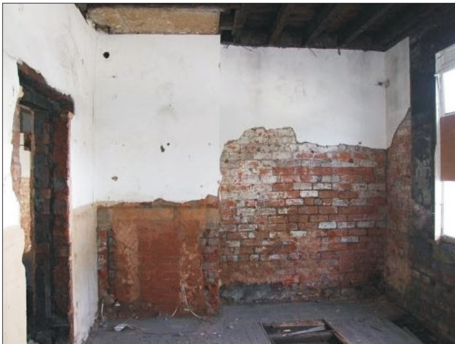
Plate 10: General view of G2, showing blocked fireplace (Film D.19)
