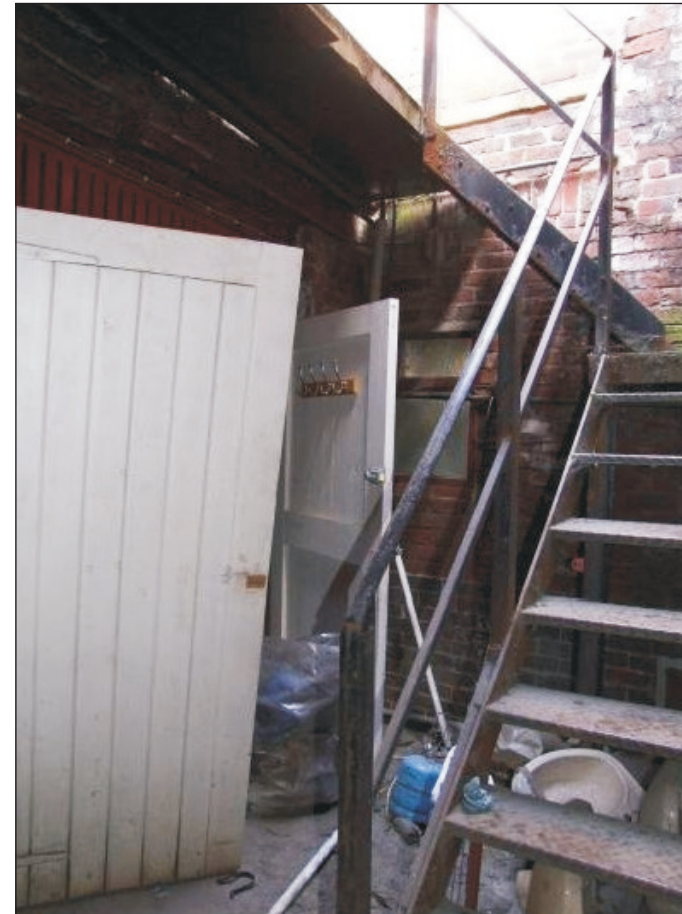
Plate 64: General view of external staircase G7 (Film D.99)
