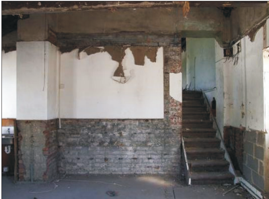
Plate 19: General view of F4, showing flue & stairs to F5 (Film D.29)
