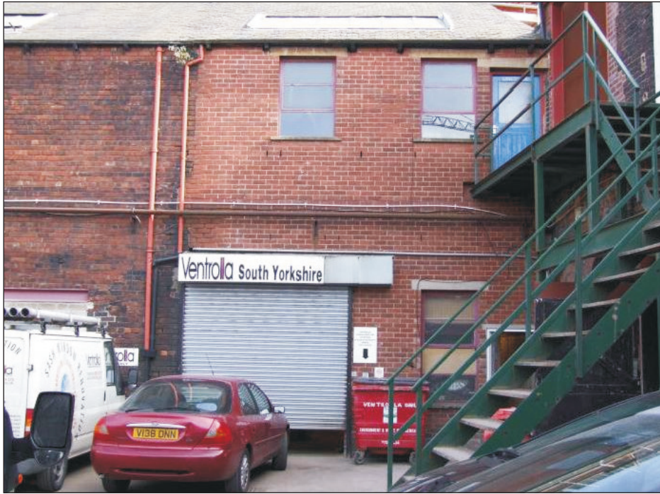
Plate 25: General view of the northwest elevation at the southwest end of the Southeast Range (Film D.37)
