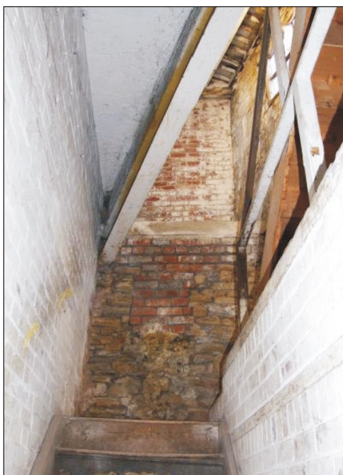
Plate 47: General view up staircase G17 (Film D.77)
