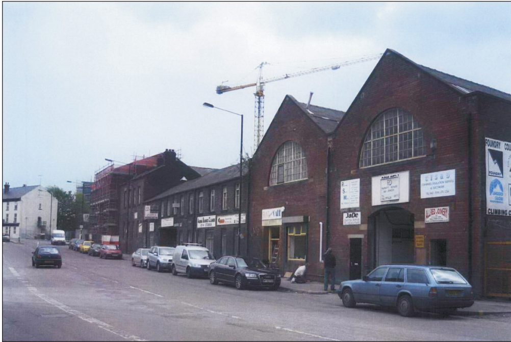
Plate 1: General view of Caledonia Works from Mowbray Street (Film D.10)
