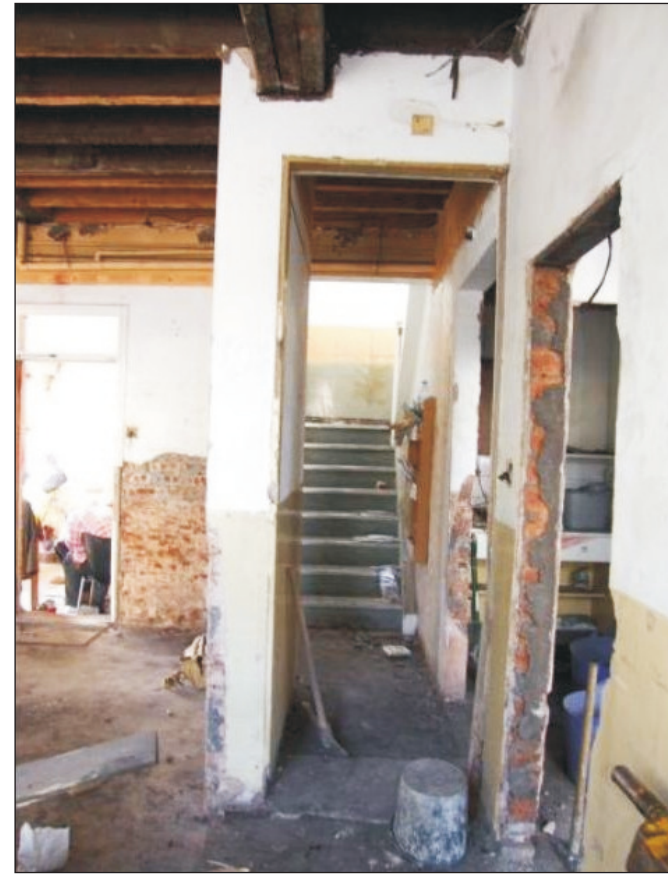
Plate 8: General view of G3, looking towards staircase G8 (Film D.16)
