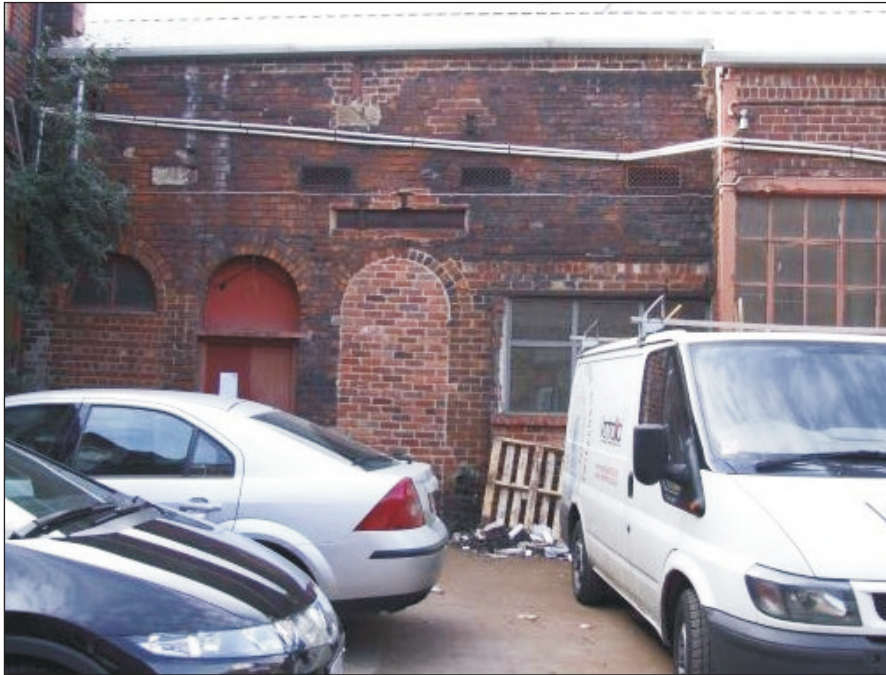
Plate 55: View of the southwest end of the southeast elevation of the Northwest Range, showing blocked arched openings and cast iron vents (Film D.84)
