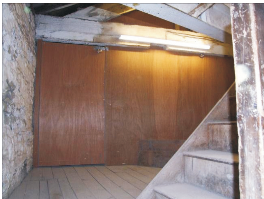
Plate 48: General view of staircase F15 & roof void F14 (Film D.78)
