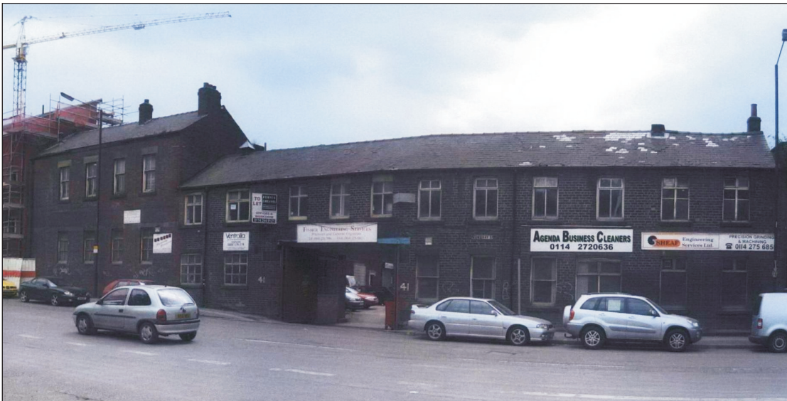
Plate 2: General view of the principal facade of the Caledonia Works, fronting Mowbray Street (Film D.04)
