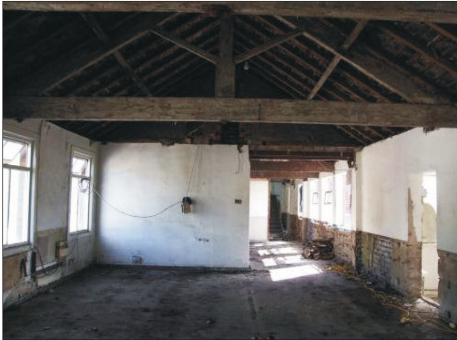
Plate 17: General view of F2, showing joggled King-Post roof trusses (Film D.26)
