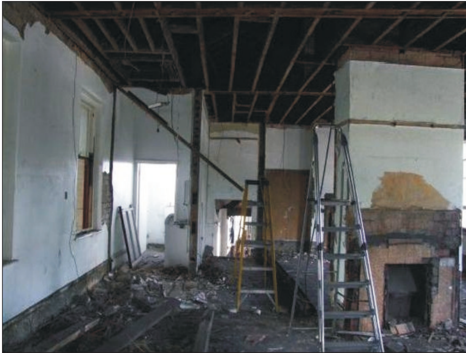
Plate 21: General view of F5, showing fireplace, and F6 beyond (Film D.31)
