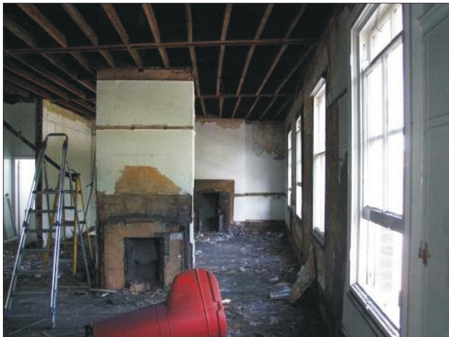
Plate 20: General view of F5, showing fireplaces (Film D.30)
