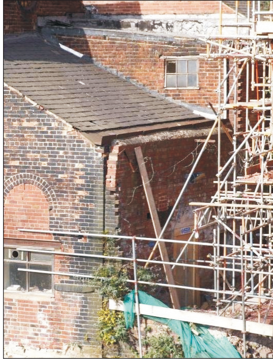
Plate 39: View of the southeast corner of the Southwest Range, showing doorway and possible blocked wall box in the southeast elevation - formerly Times Steel Works (Film D.62)
