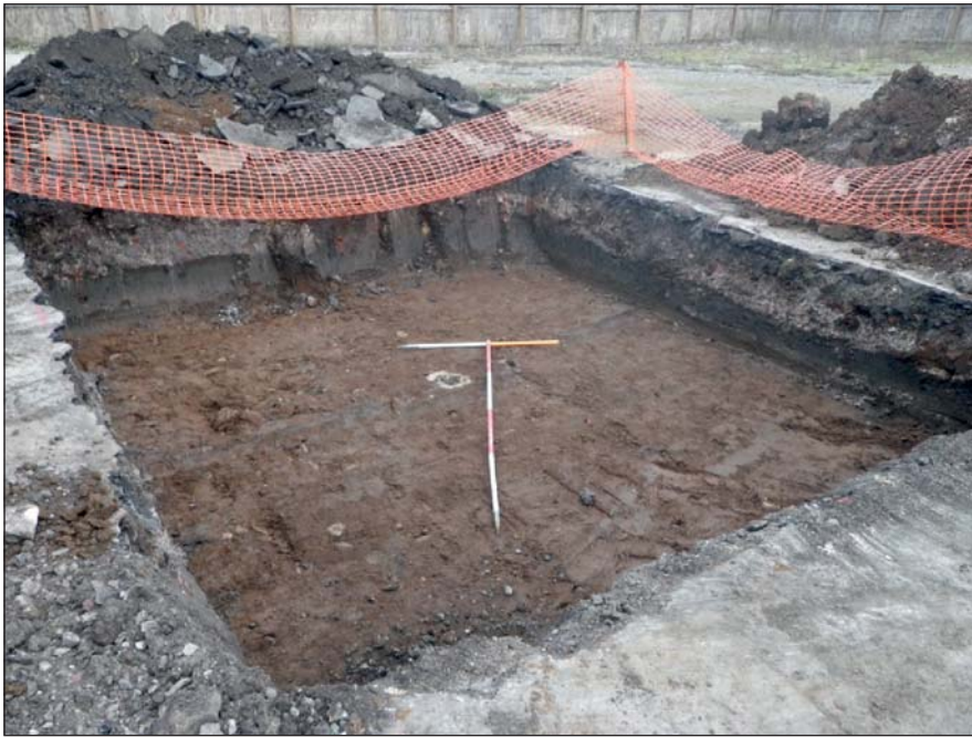
Plate 1: Trench 1, garden feature 107 in foreground, looking north.
