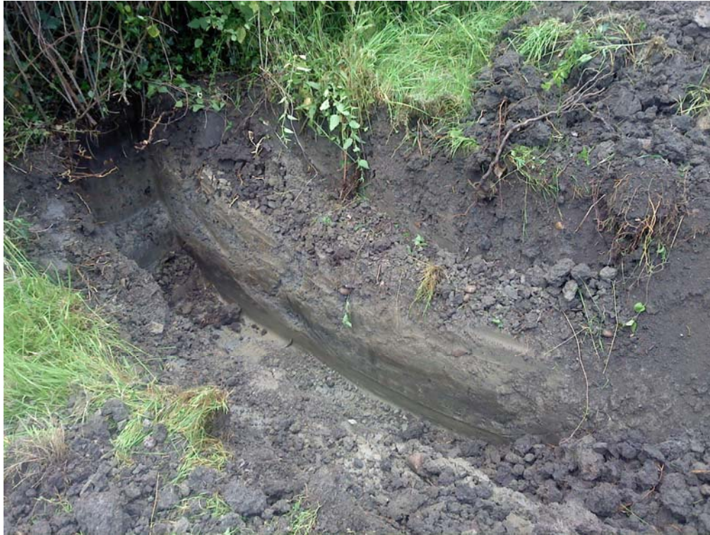
Plate 1: Launch and reception pit north of Bishampton
