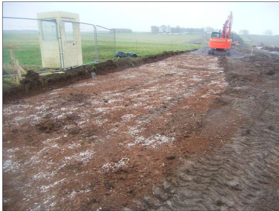
Plate 4: Formation level of trackway following machine excavation
