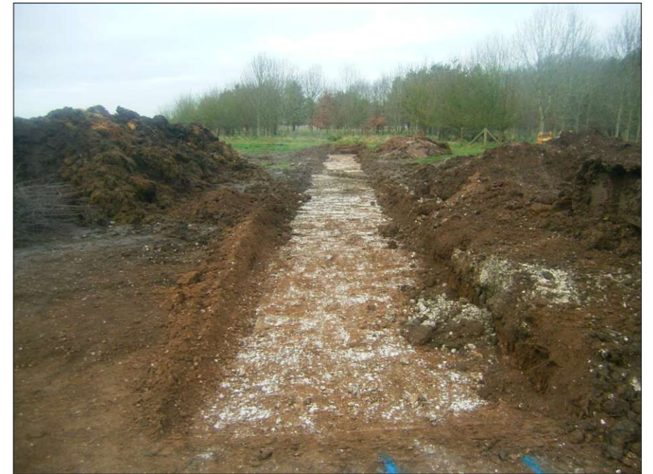
Plate 3: Drainage trench at Mile Ball
