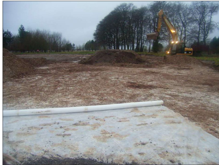
Plate 2: Stripping of marshalling/muster area, Mile Ball
