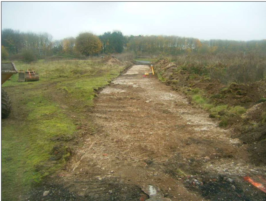
Plate 2: Northern end of Shuttle Road, following machine excavation
