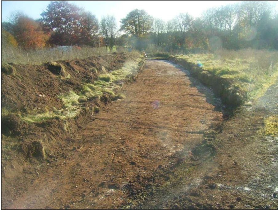
Plate 1: Southern end of Shuttle Road, following machine excavation
