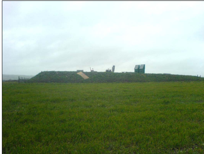
Plate 1: Grimstone Reservoir looking west
