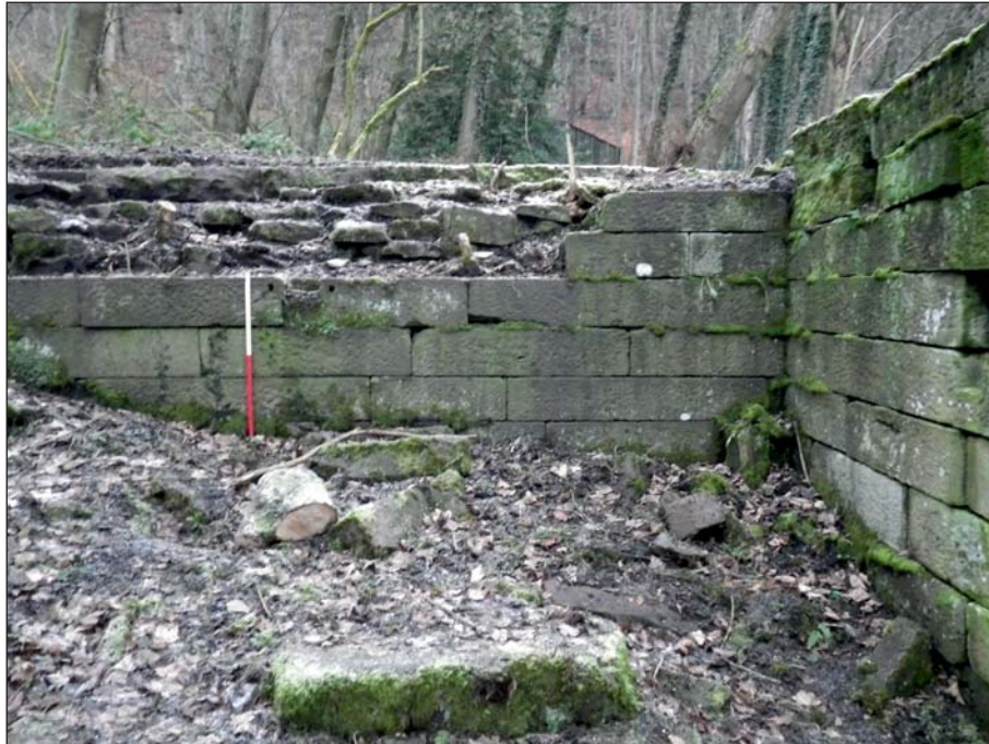
Plate 11: South facing elevation of 107 , defining the presumed location of Wheel 2
