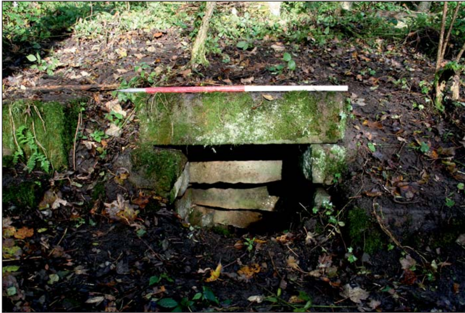
Plate 13: Detail of void between 105 and 106 , showing stepped roof of goit between the dam and Wheel 3
