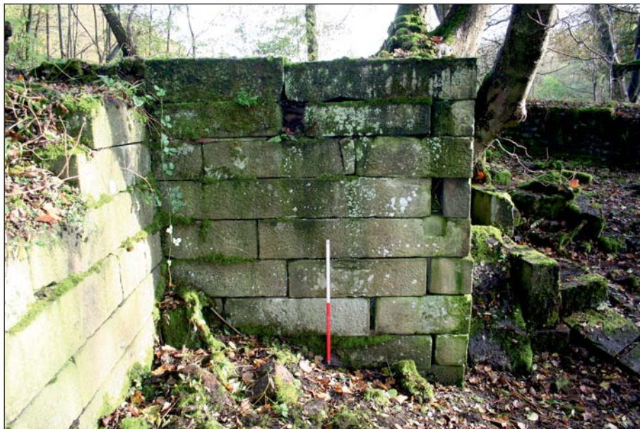
Plate 12: Possible beam slot in west facing elevation of 107
