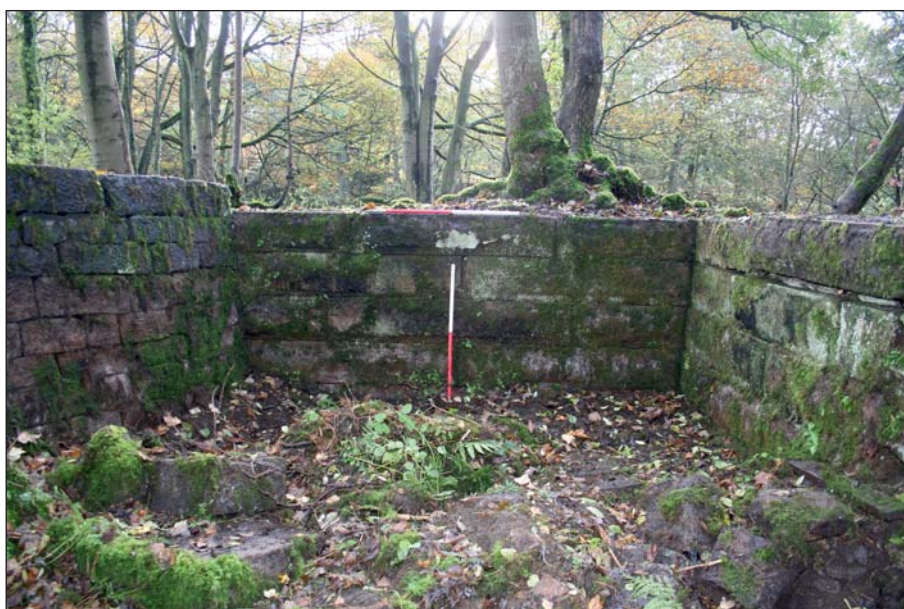
Plate 6: North elevation of 108 within forebay
