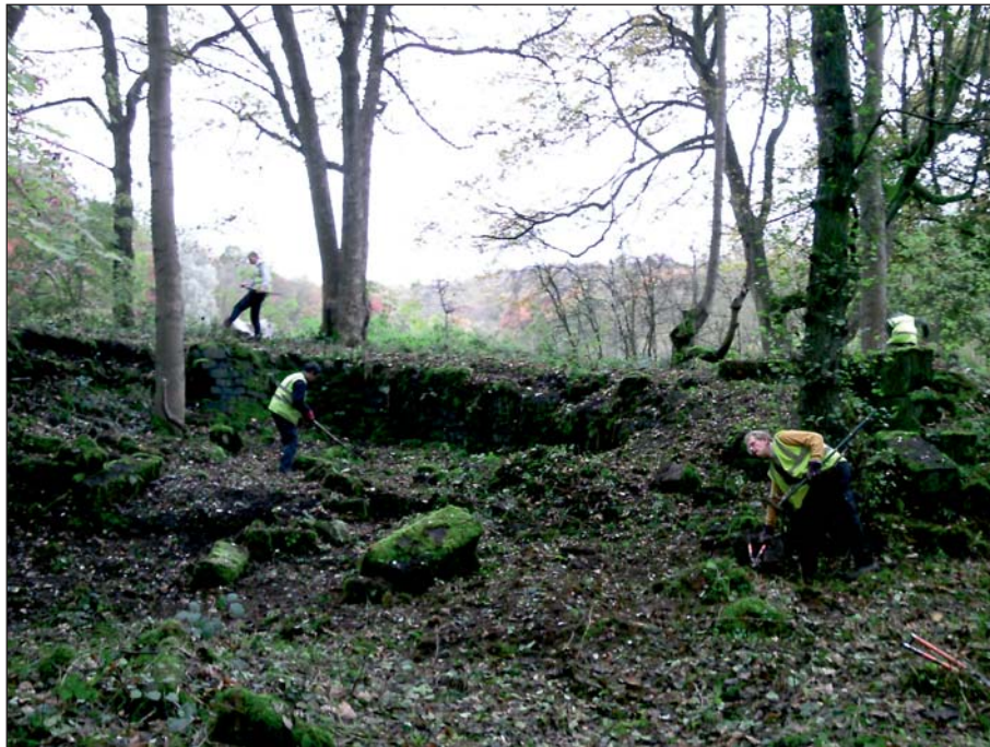
Plate 1: Volunteers working on clearing the mill site
