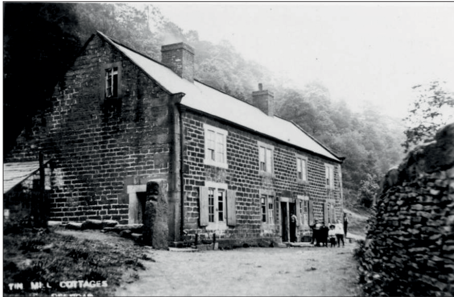
Plate 17: Workers cottages (Courtesy of Hunshelf Parish Council)
