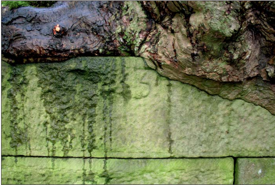
Plate 9: Masonry marks, a '3'
