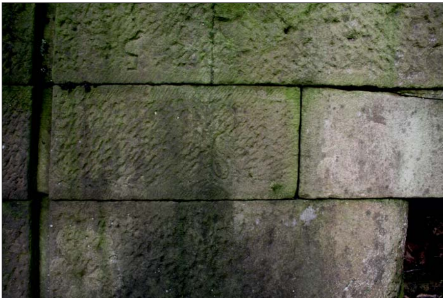
Plate 10: Masonry marks, a '5' (inverted) and '6'
