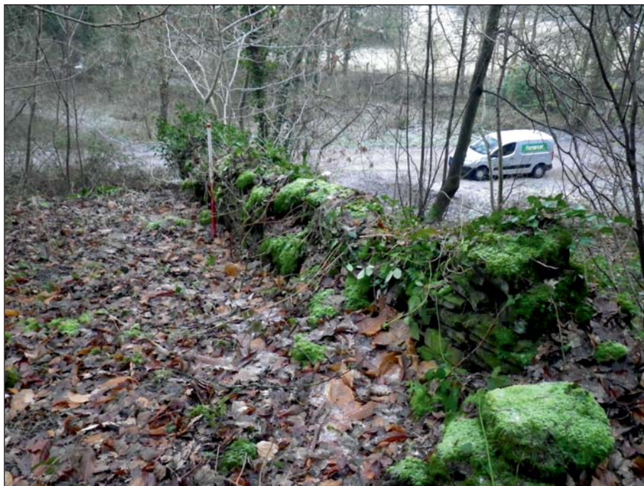
Plate 16: Example of revetment walls on hillside above the mill
