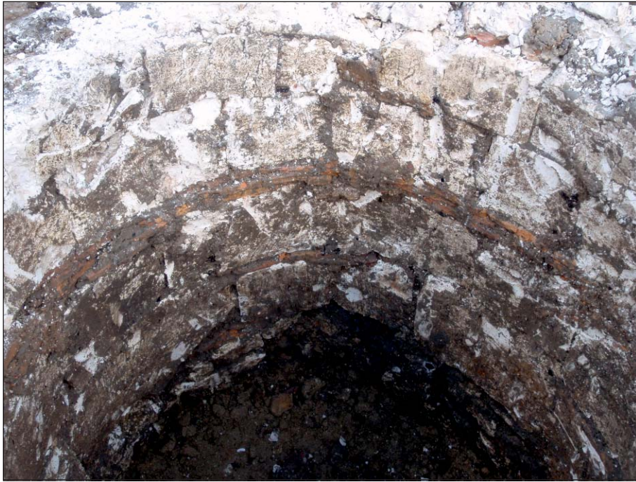
Plate 5: Detail of well 207, showing tile lacing courses
