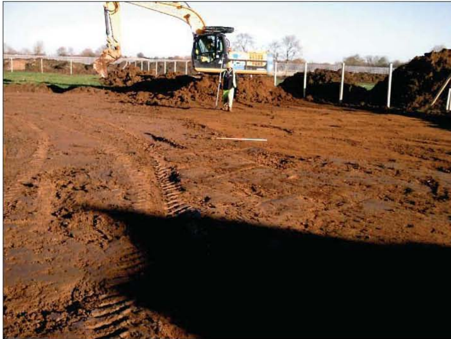
Plate 3: Depth of material removed during strip for Trench 2 (compound and parking)
