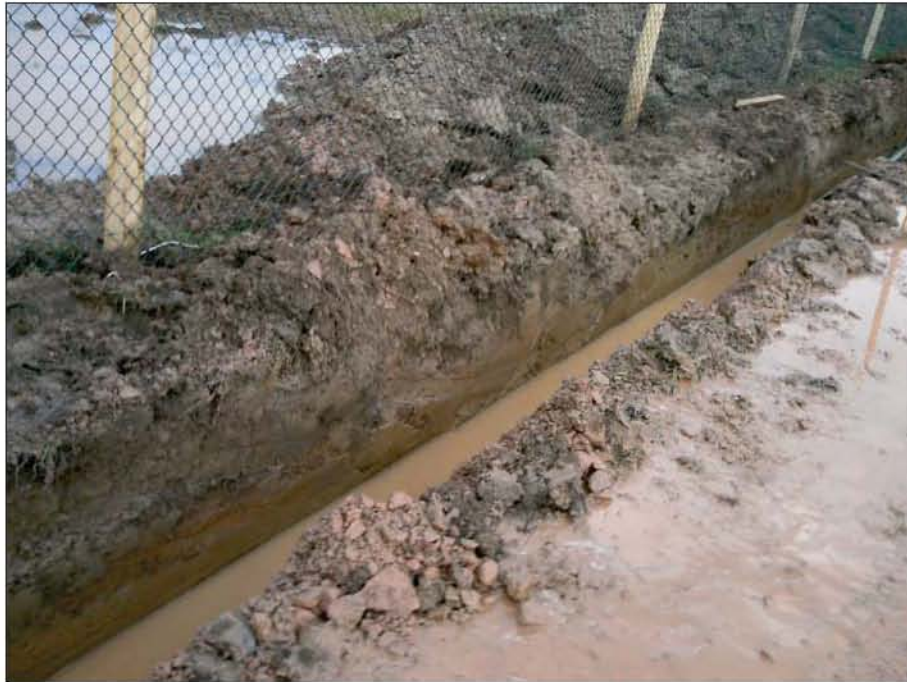
Plate 7: Depth of excavation for Trench 4 services
