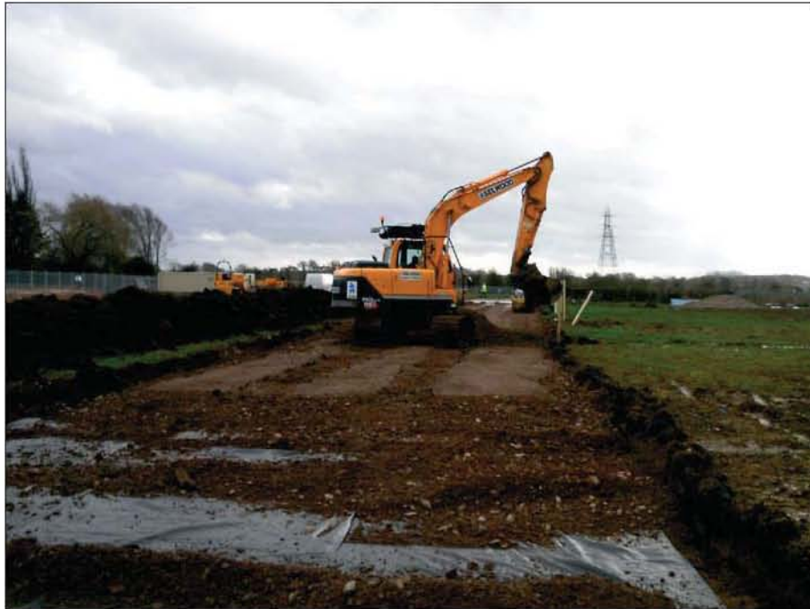
Plate 1: Depth of material removed during strip of Trench 1 (Haulage Road)
