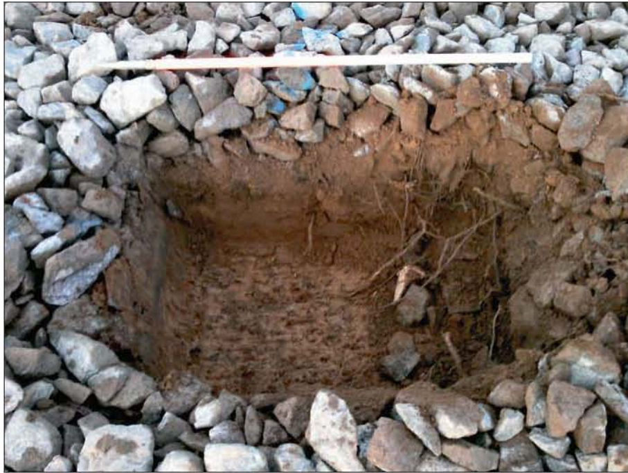
Plate 5: Depth of material excavated for Trench 3 foundation pads
