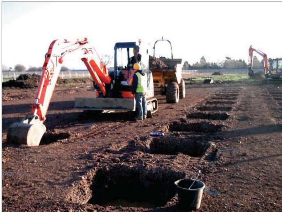
Plate 4: Excavation of foundation pads in Trench 3
