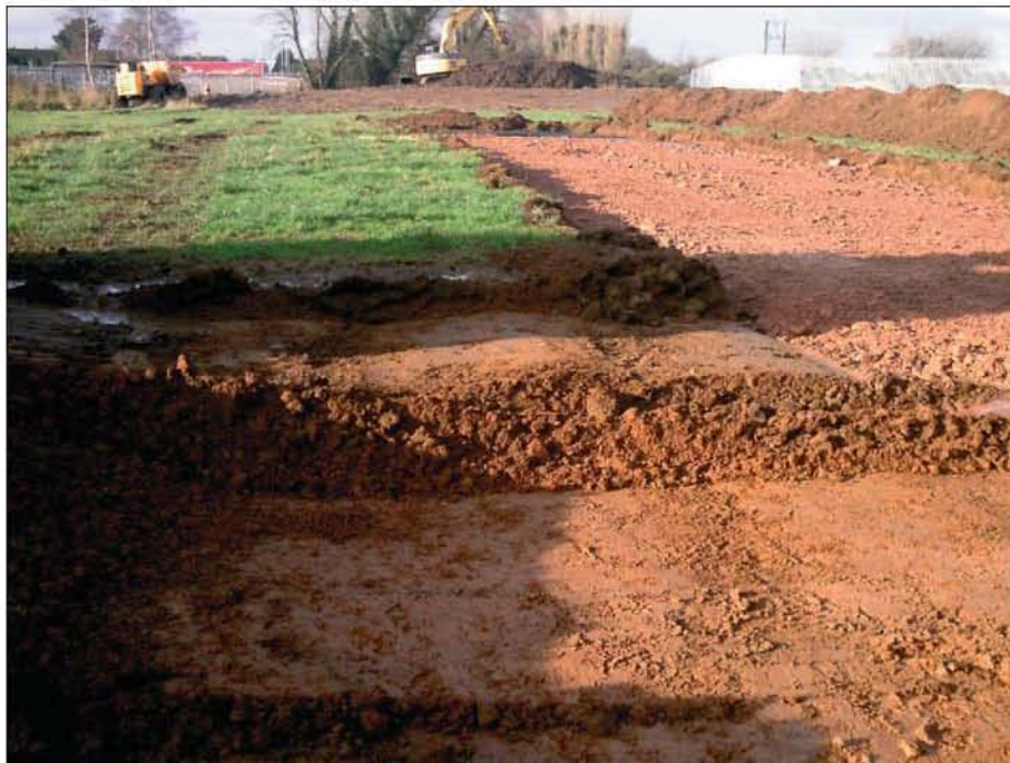
Plate 6: Depth of material stripped in Trench 3
