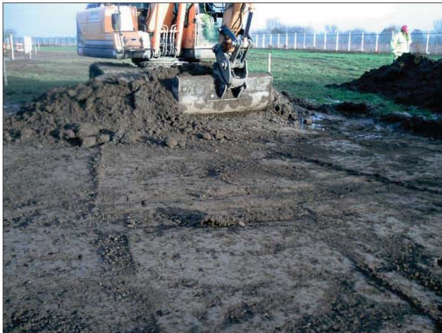
Plate 2: Removal of topsoil during strip for Trench 2 (compound and parking area)
