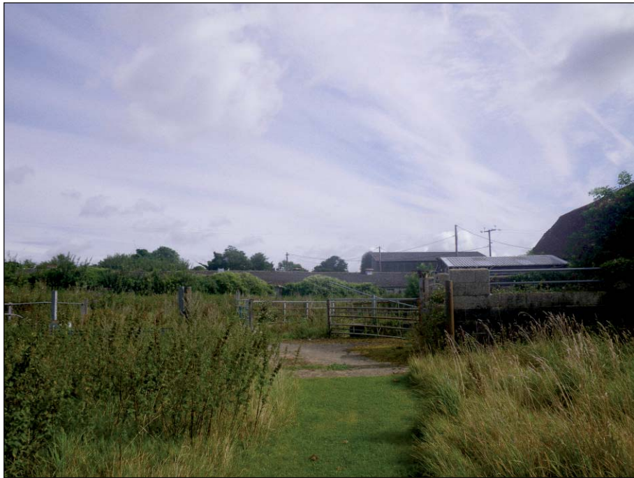
Plate 1: Outbuildings and shed within the Scheduled Monument, view from south-east
