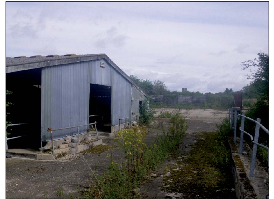
Plate 6: View towards Knowlton Church from south
