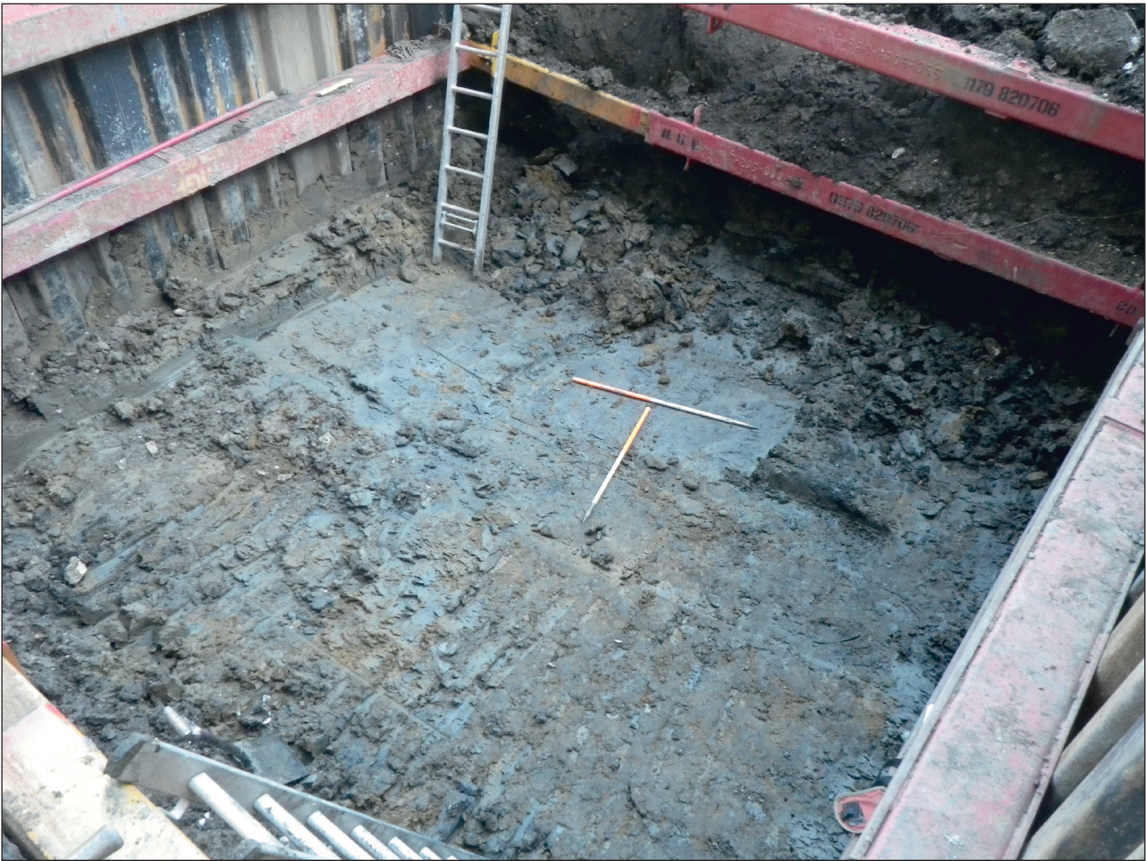
Plate 3: General shot of base of excavation area
