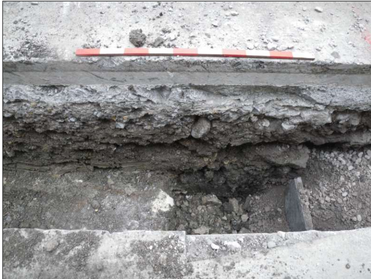
Plate 2: West facing section of Trench 3
