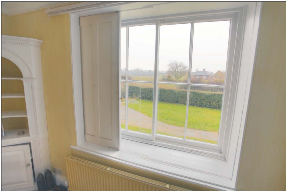
Plate 10 : Sliding shutter within horizontal sliding sash window
