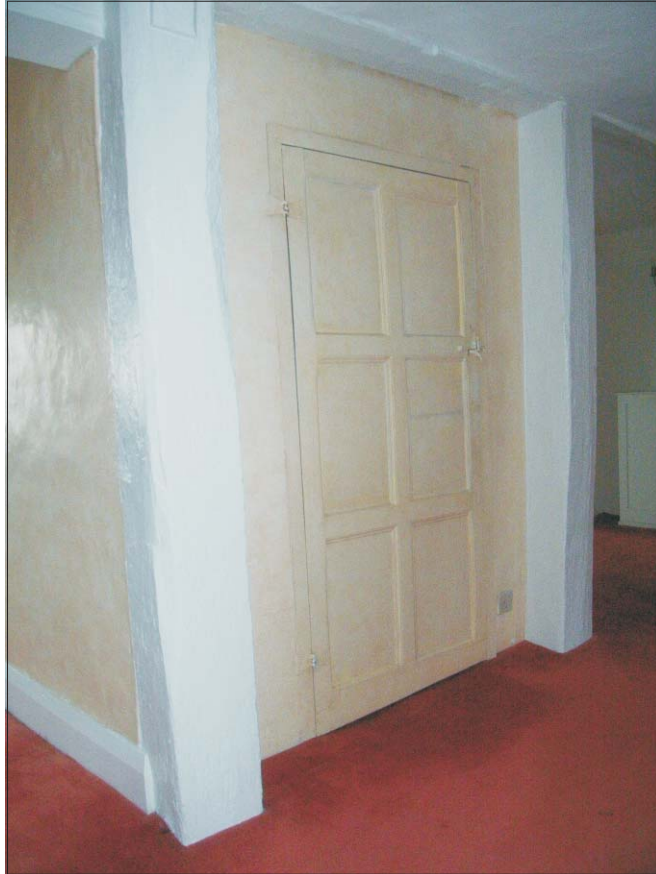
Plate 19 : First floor - Entrance to airing cupboard
