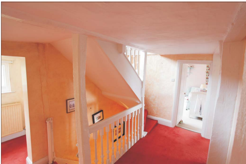
Plate 18 : First floor - Landing
