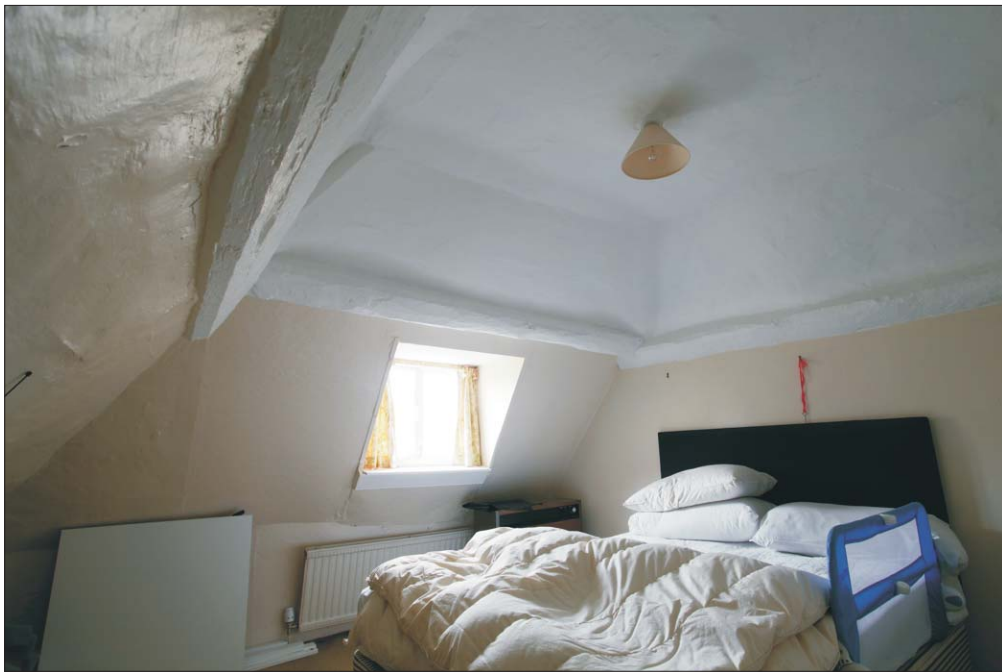
Plate 24 : Attic floor - Bedroom 5
