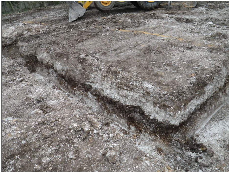
Plate 1: Made ground over buried topsoil and subsoil, from south-east
