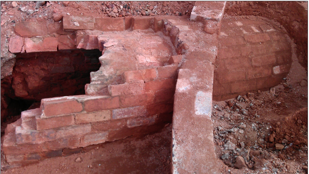
Plate 5: Angled smoke flue passing through outer wall of damper area
