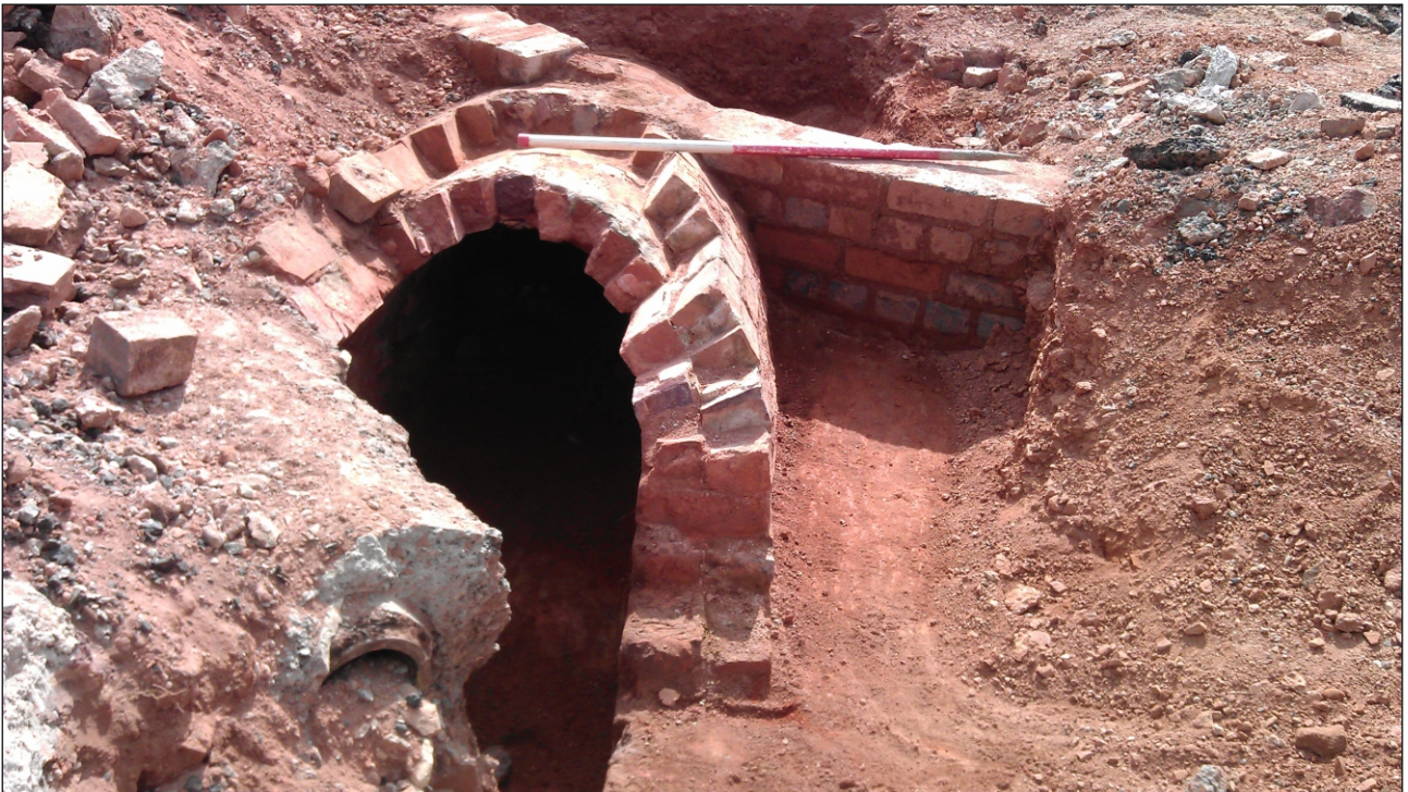
Plate 3: Smoke flue showing arched brick profile
